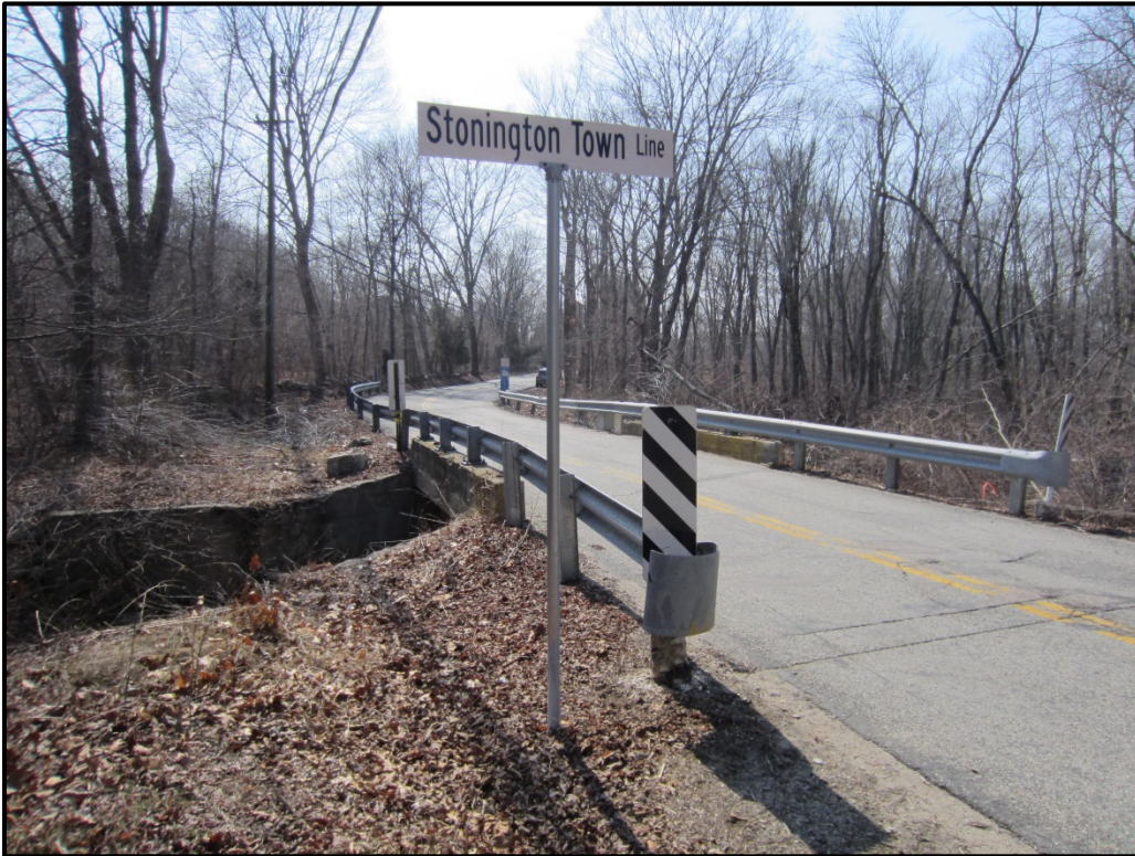
Photo 10- Looking Southerly along Roadway (3/8/2016)
