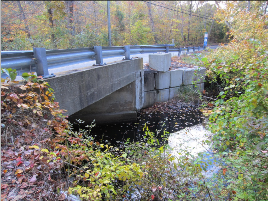
Photo 5- Downstream Bridge Face (10/16/2015) Note Concrete Block Wingwall
