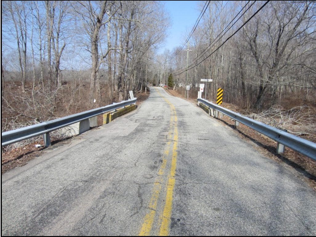
Photo 9- Looking Northerly along Roadway (3/8/2016)
