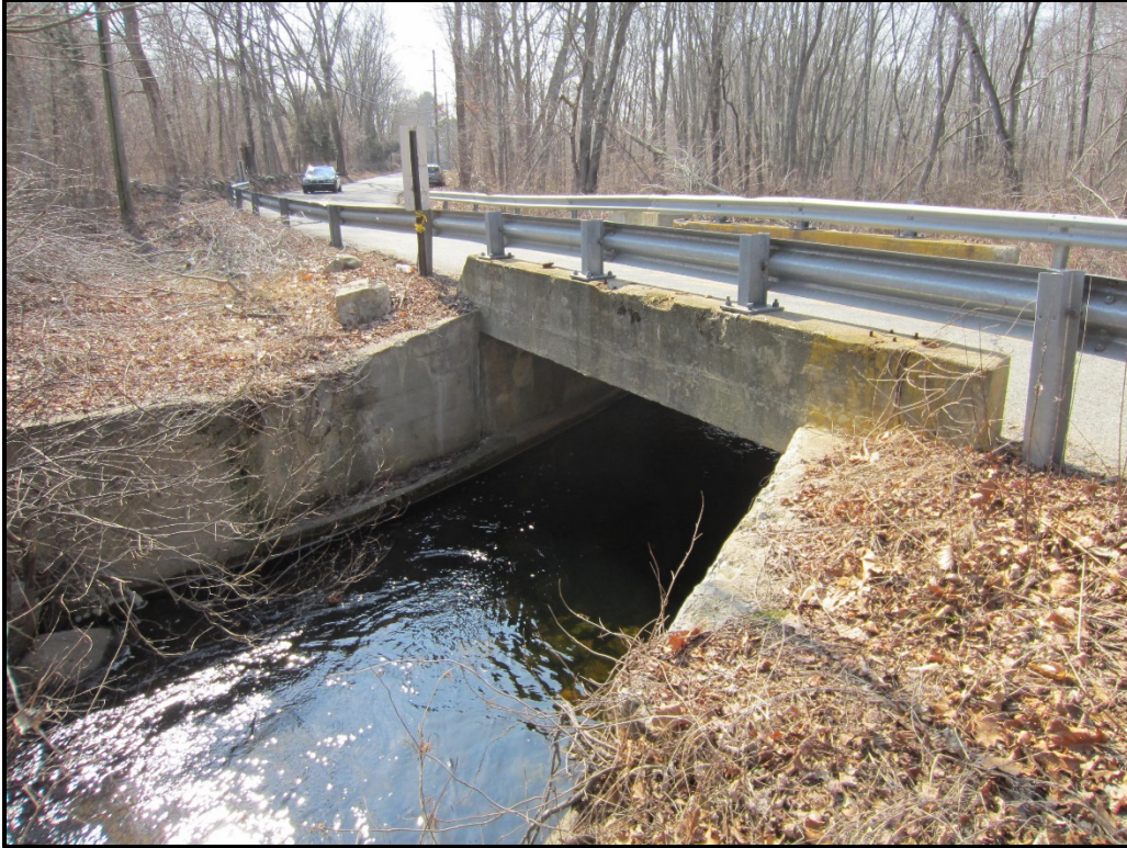
Photo 3- Upstream Bridge Face (3/8/2016)
