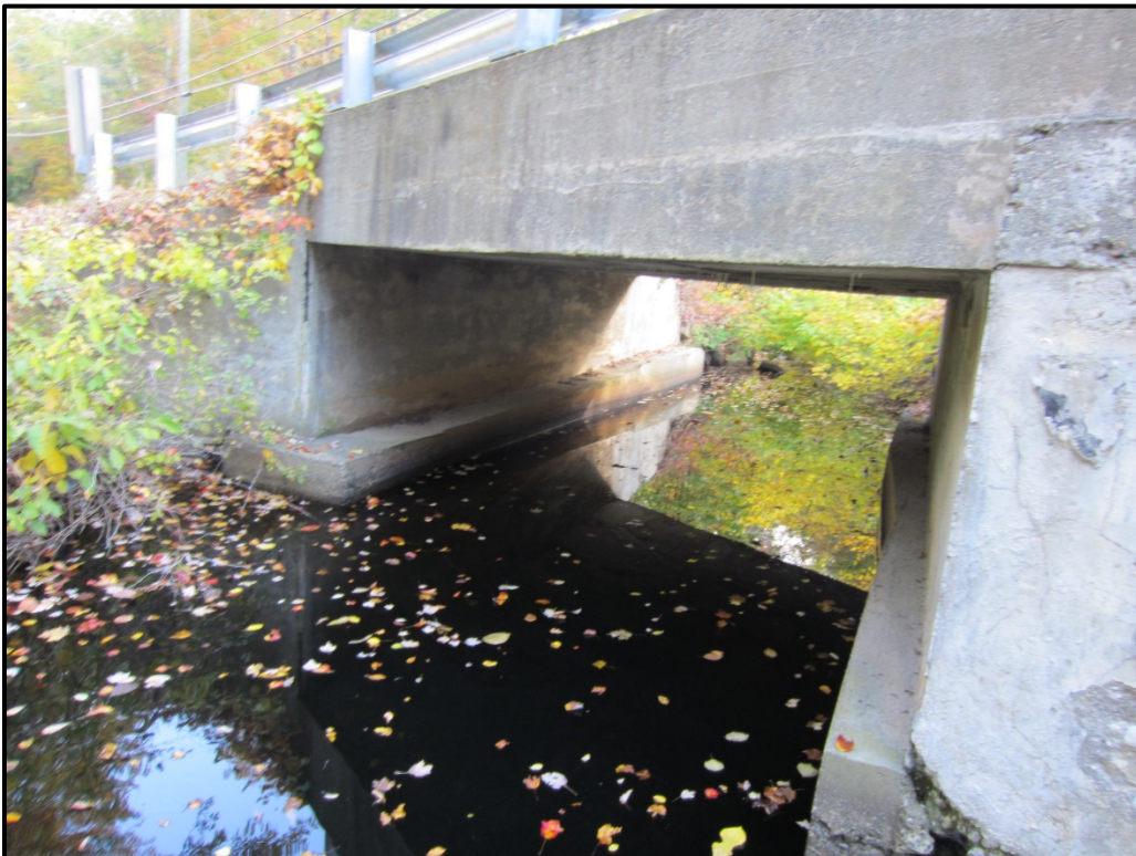
Photo 8- Looking Upstream through Bridge Opening (10/16/2015) Note Concrete Shelves both Sides
