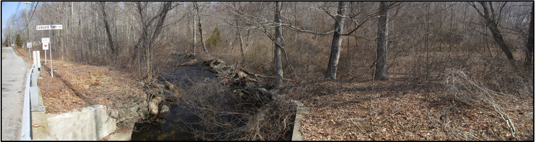
Photo 1- Looking Upstream from Bridge (3/8/2016)
