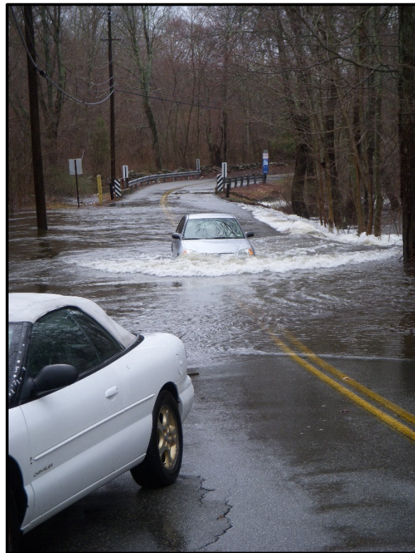
Photo 12- Looking Southerly towards Bridge (3/30/2010)
