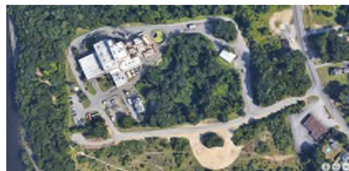
Preston Waste Energy Facility
