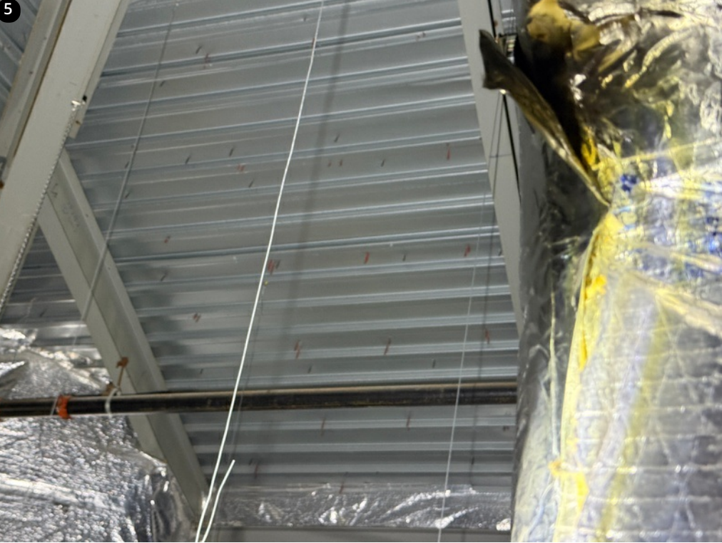
Fasteners observed penetrating deck- 11/23/24
