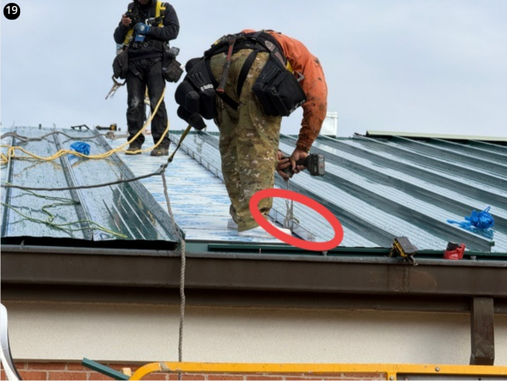
Crew fastening clips on field section- 11/27/24
