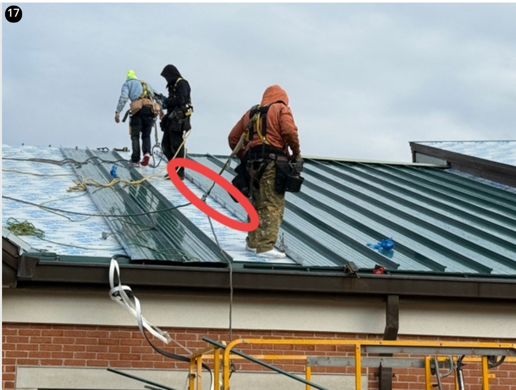
Crew installing panels on field section- 11/29/24
