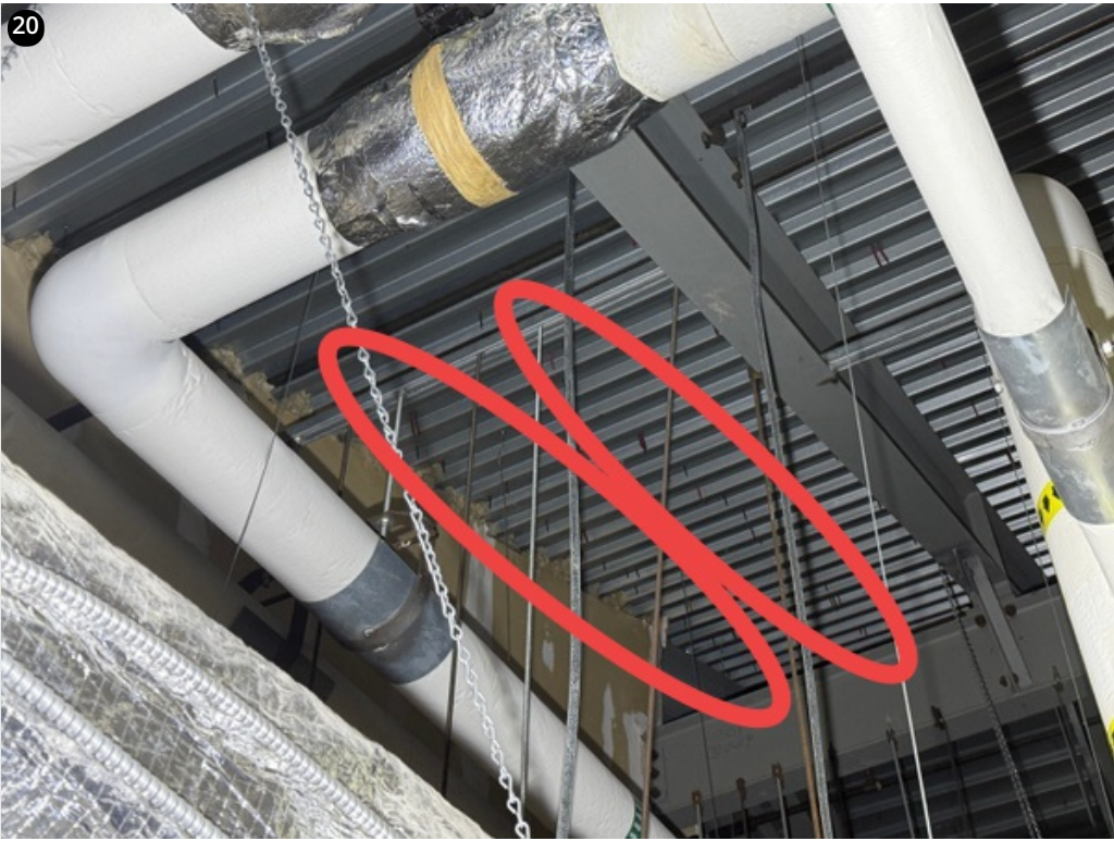
Fasteners observed penetrating deck- 11/29/24
