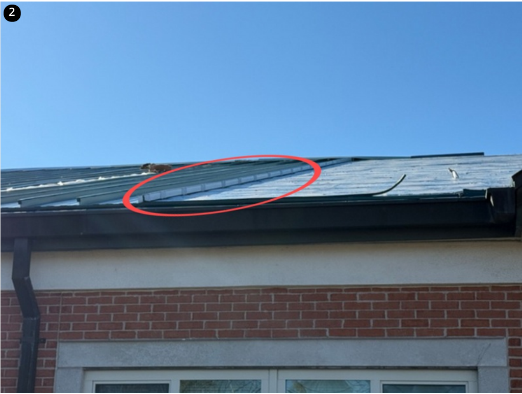
Panels installed Saturday 11/23/24
