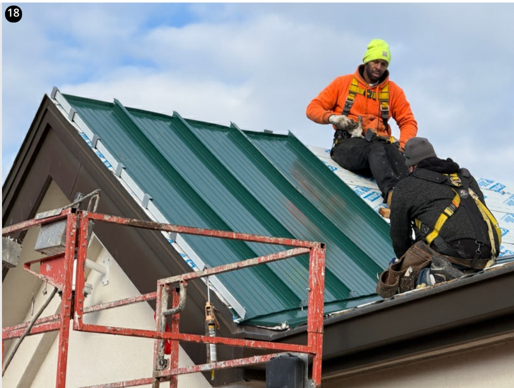
Crew installing panels on dormer- 11/29/24
