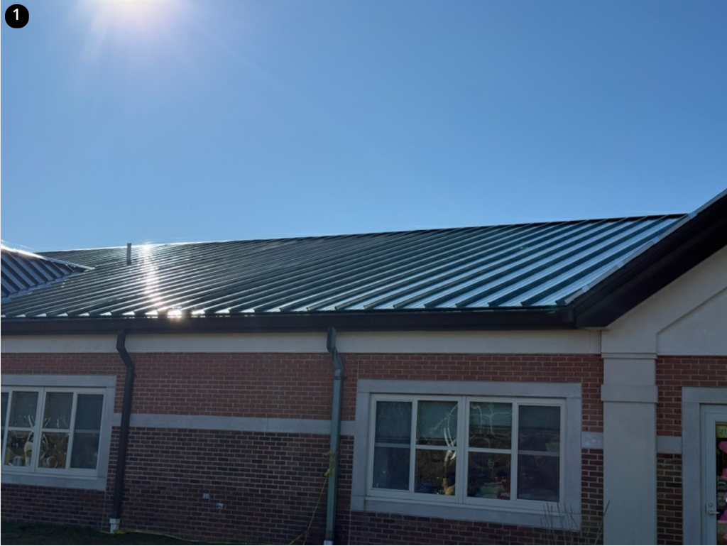
Panels installed Saturday 11/23/24
