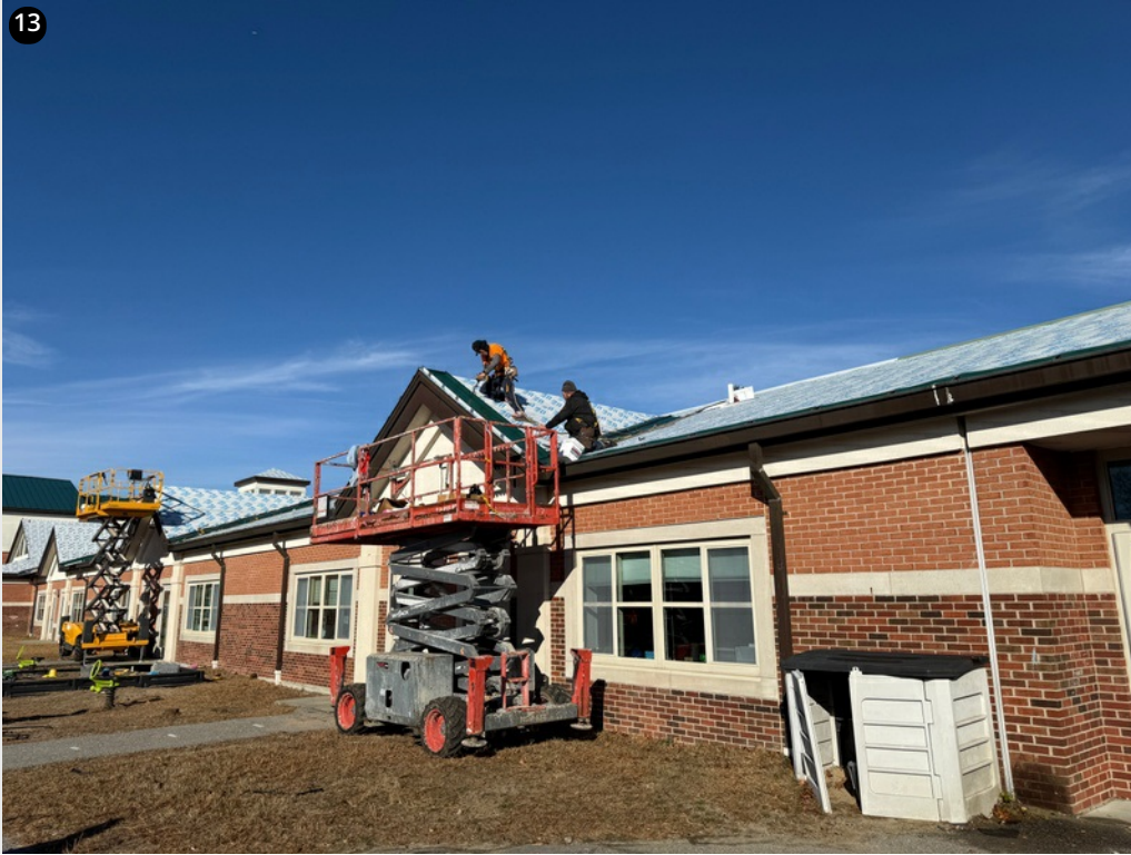
Crew installing panels on dormer- Courtyard side- 11/27/24
