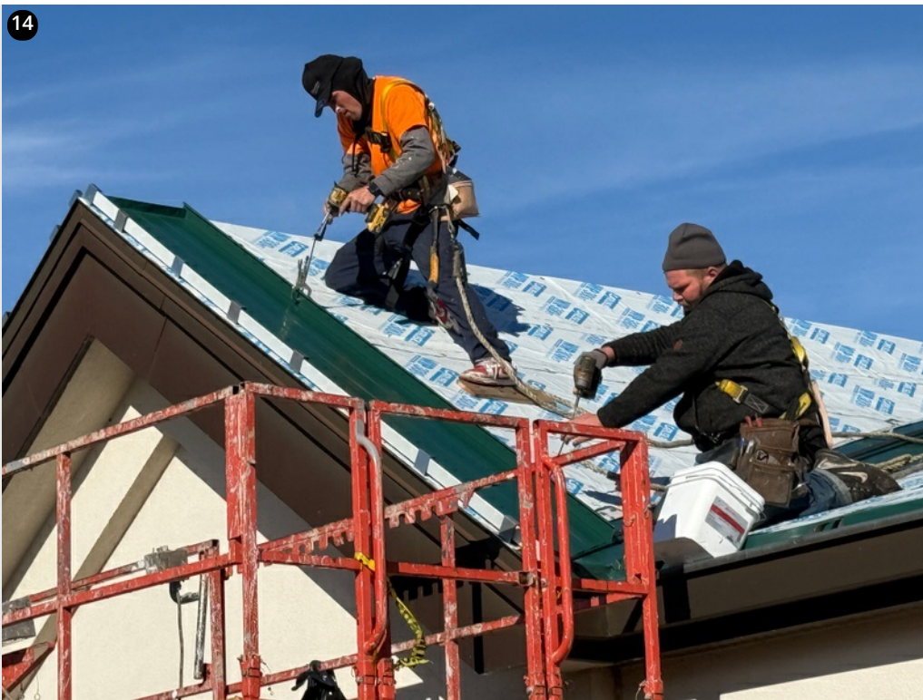
Crew fastening panel clips on dormer using 16" fasteners- 11/27/24
