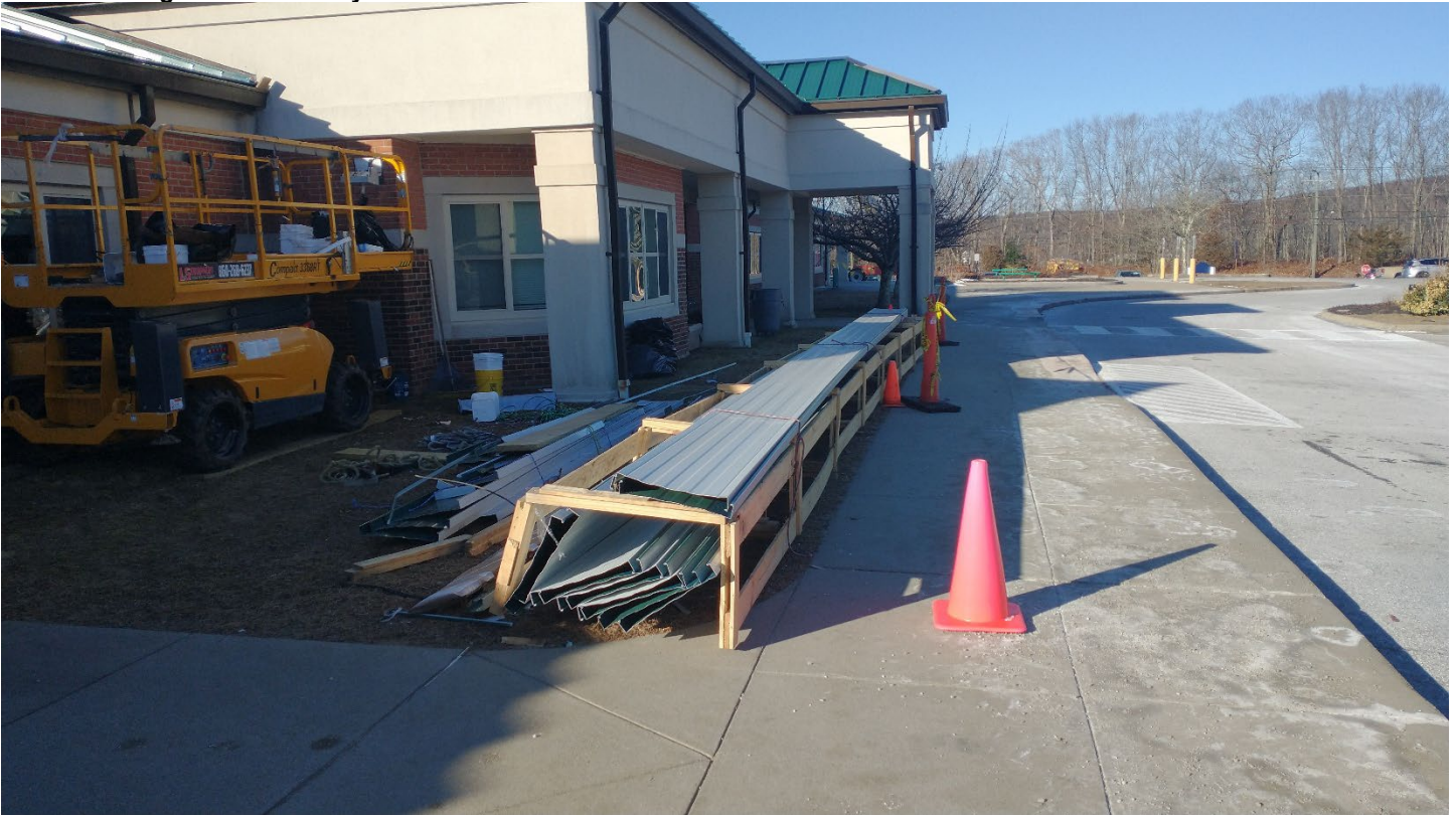
Area for storage of the workdays material.
