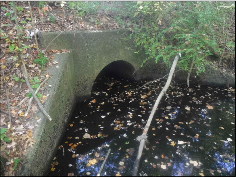
UPSTREAM (48" RCP SQUARE EDGE WITH HEADWALL)
