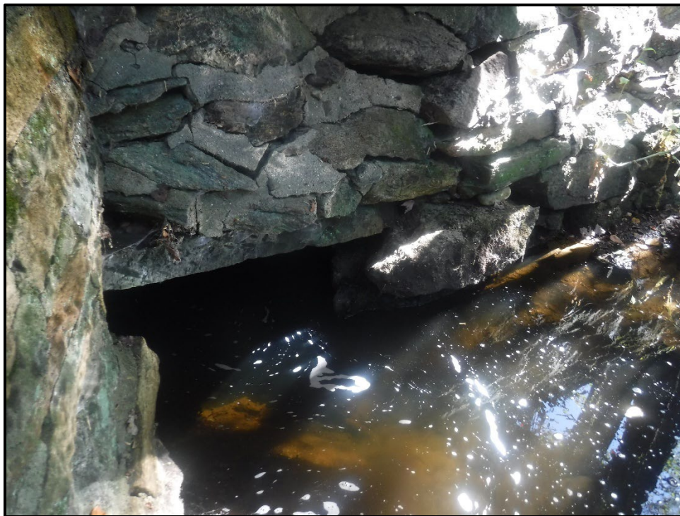
Multi-Stage Structure Outlet (Downstream)
