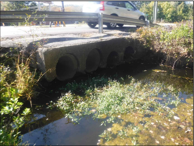
UPSTREAM (4 x 24" RCP SQUARE EDGE WITH HEADWALL)
