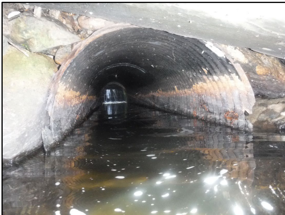
Internal Photo of 36" Culvert (Multi-Stage Outlet) with Flow Seen Penetrating Stop Boards at Head of Pipe.
