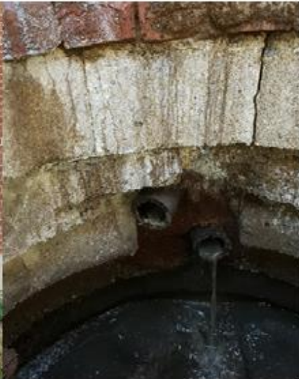
Figure 4: Force Main Discharge
