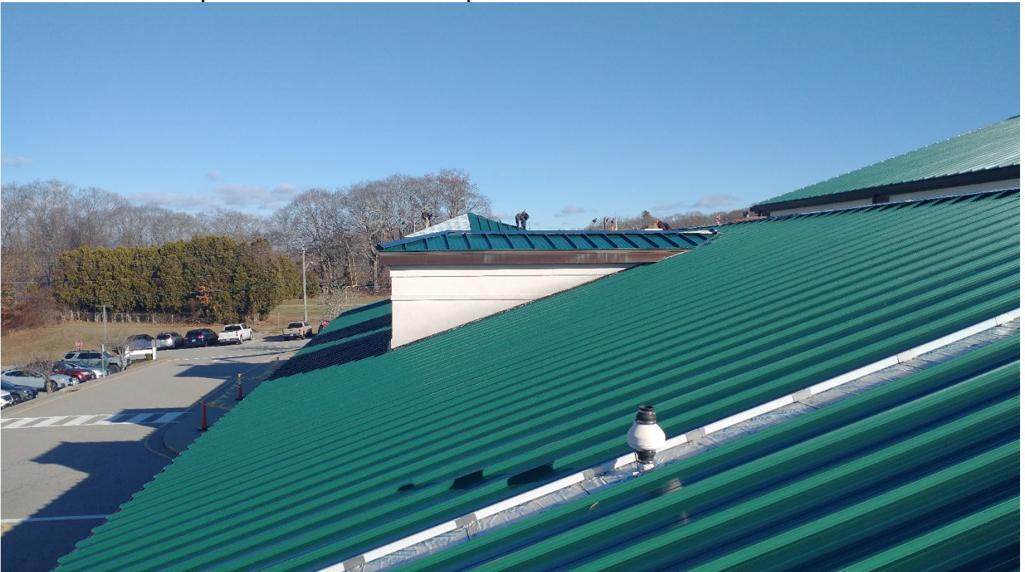
Roof A – Vent needs temp removal to install the new roof panels
