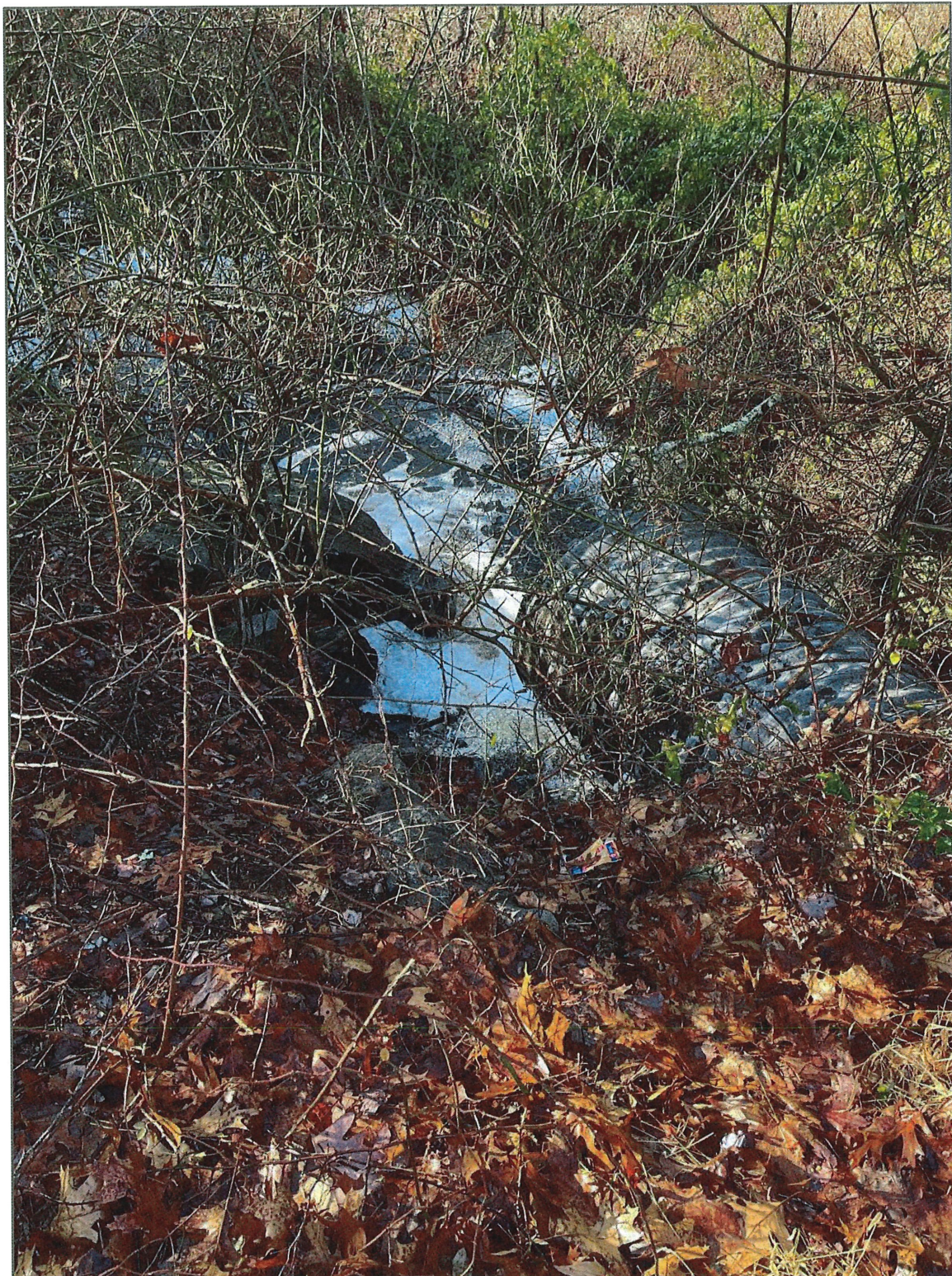
Photo 9: Auxiliary spillway outlet
