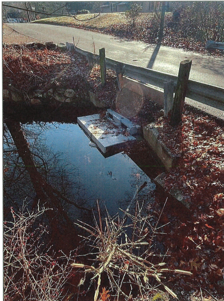
Photo 6: Principal spillway inlet with cover
