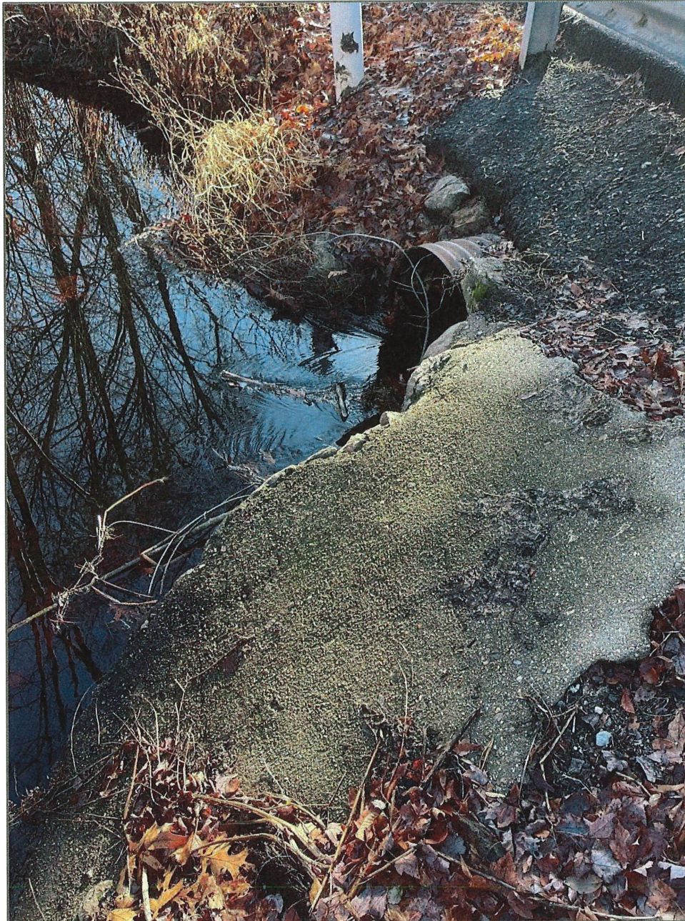
Photo 8: Auxiliary spillway inlet
