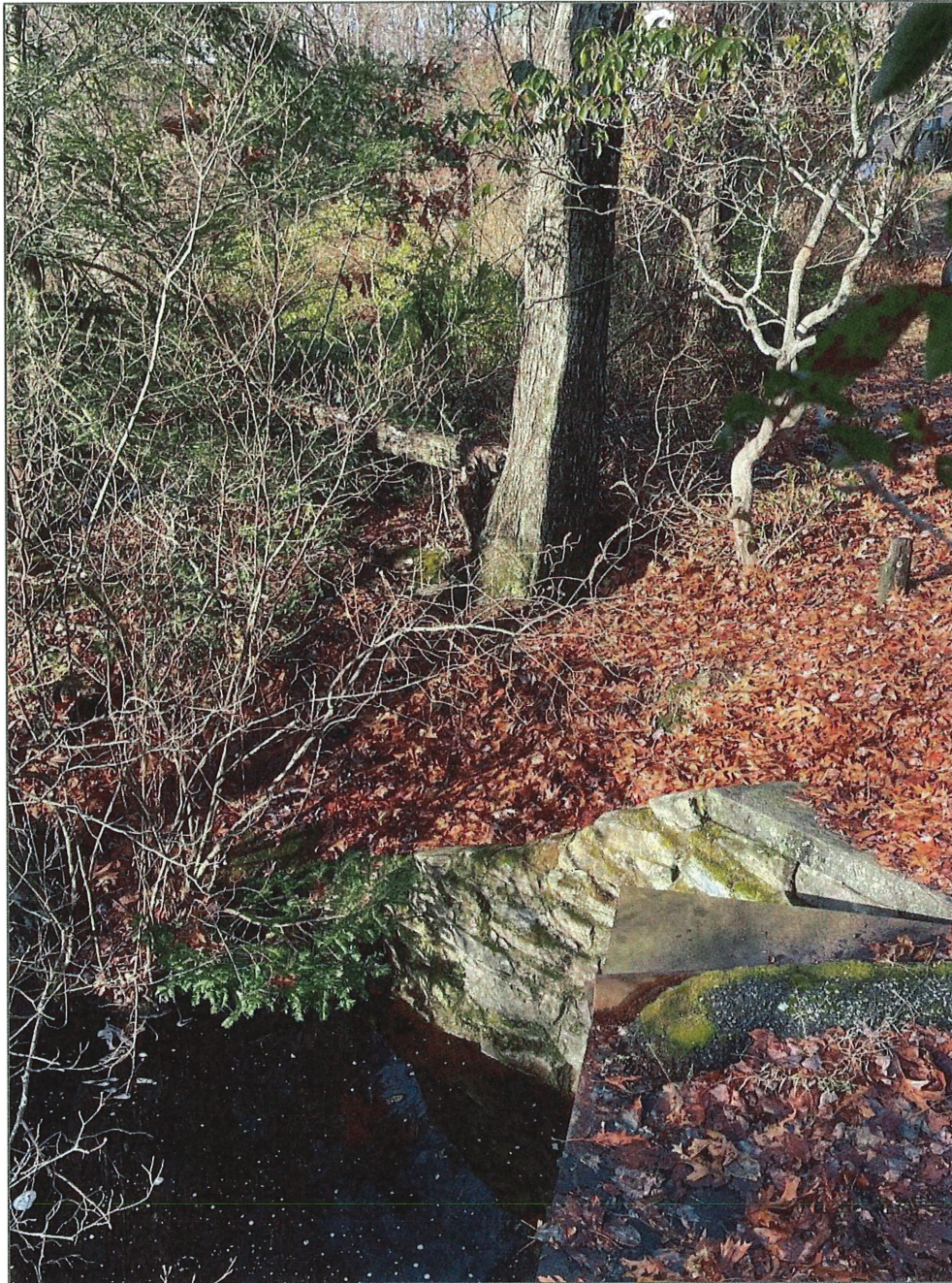
Photo 2: Downstream face of embankment
