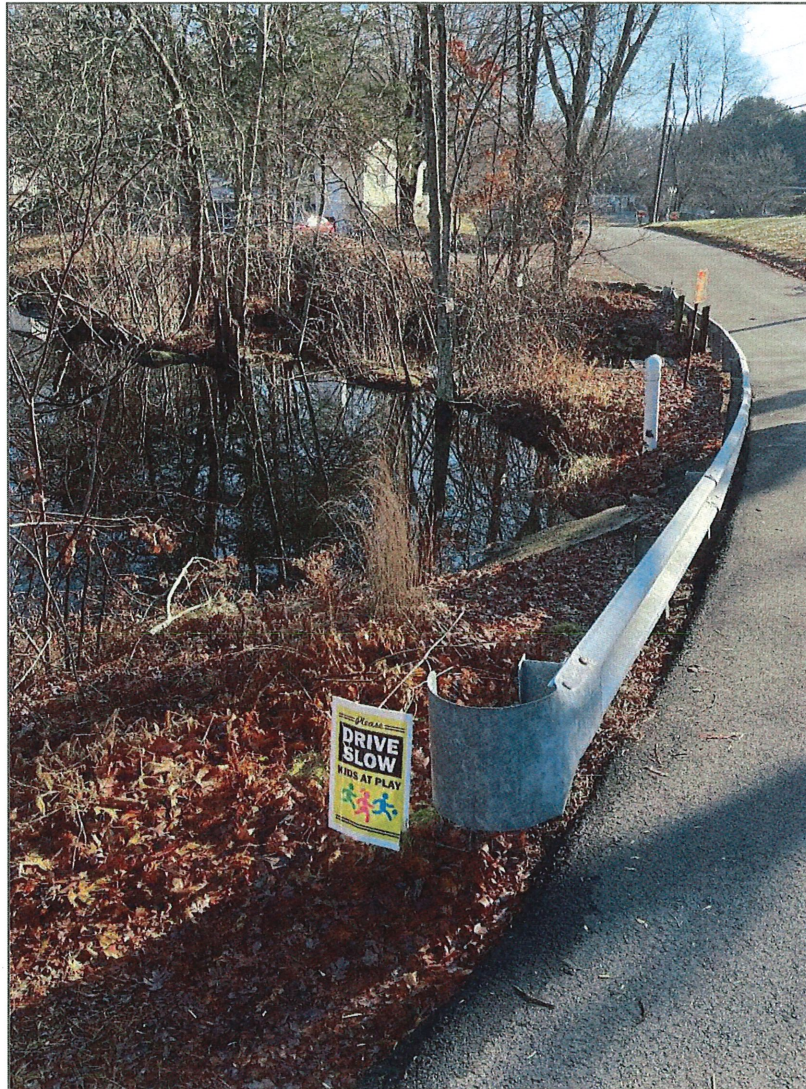
Photo 1: Upstream face of embankment
