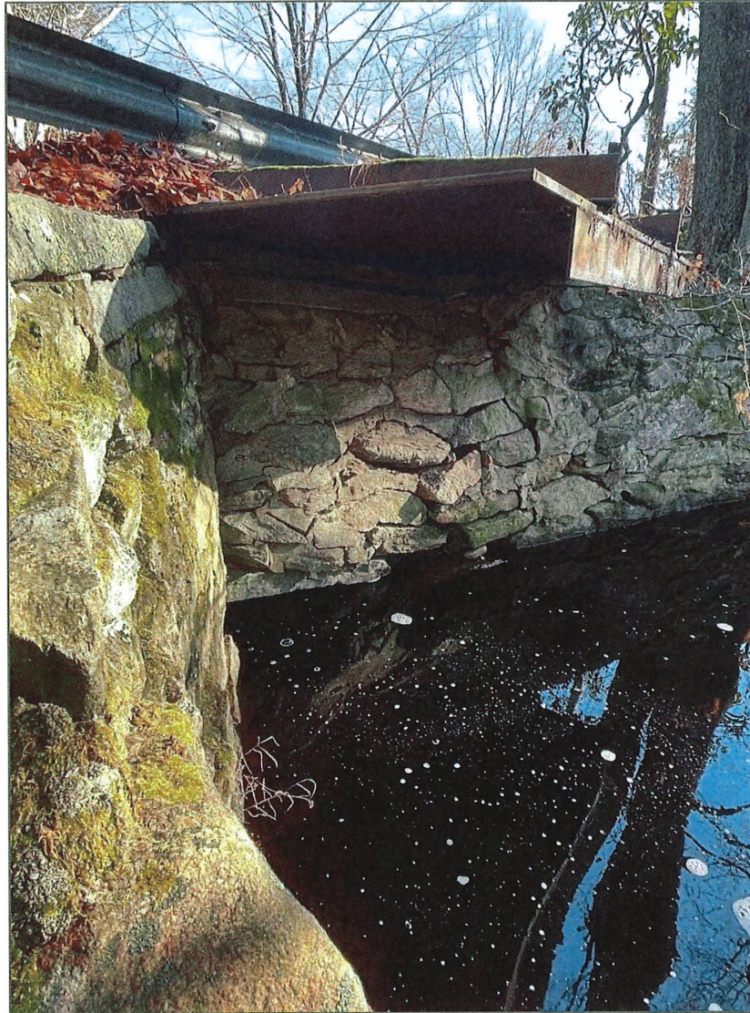
Photo 7: Principal spillway outlet
