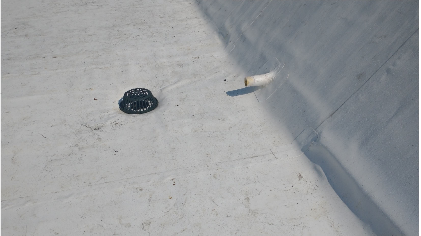
Roof B – Roof drain & over flow pipe
