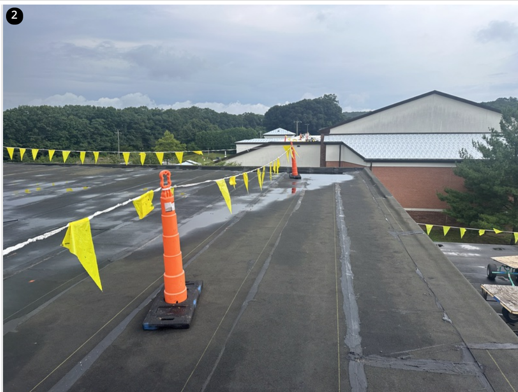
Good slope toward corner drain
