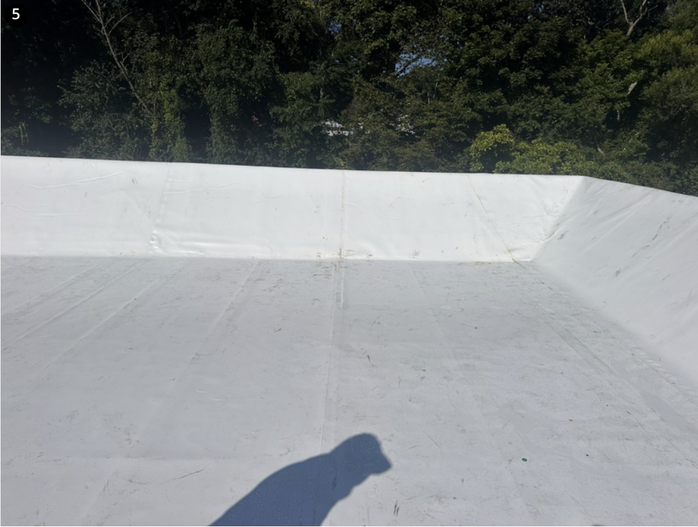
Overview- Cap sheet installed on North West corner
