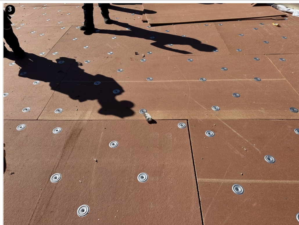
Overview- Fastening pattern on cover board
