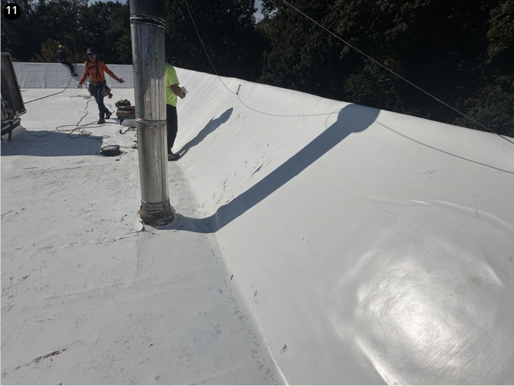
Cap sheets installed around stack
