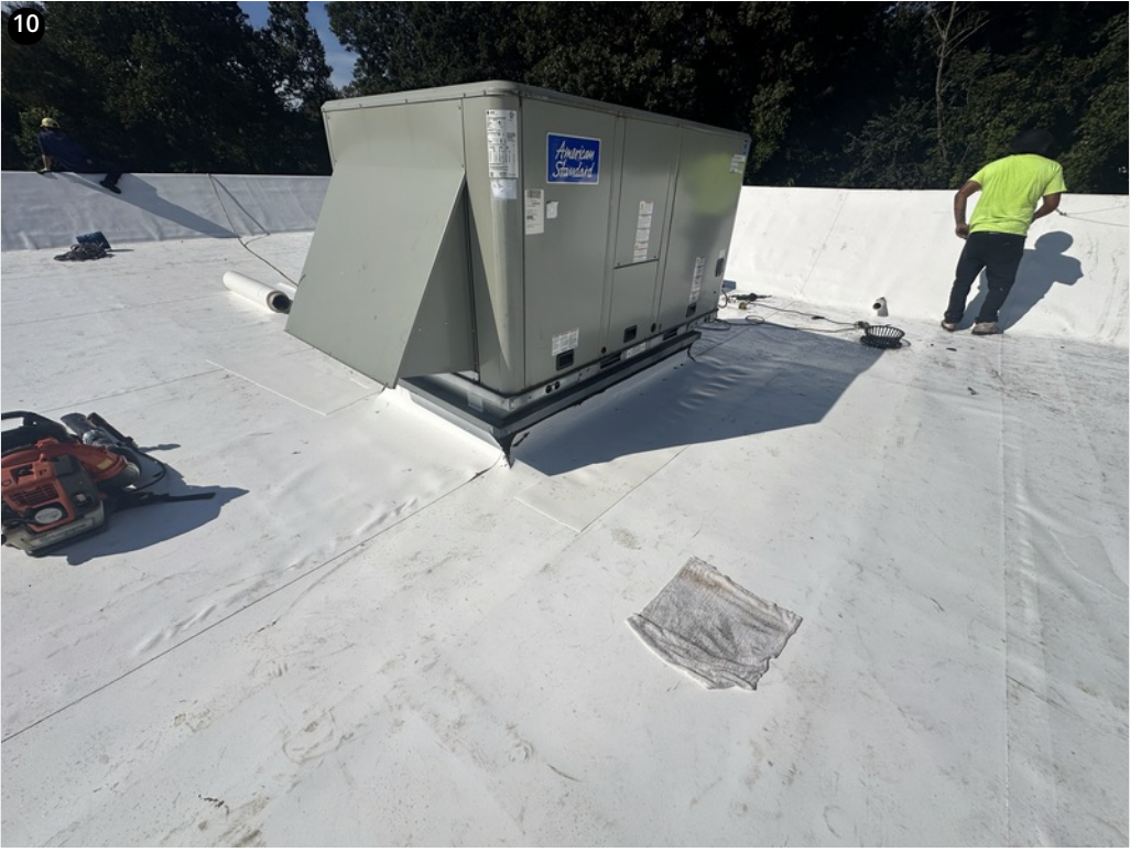
RTU- Curb flashings prepped
