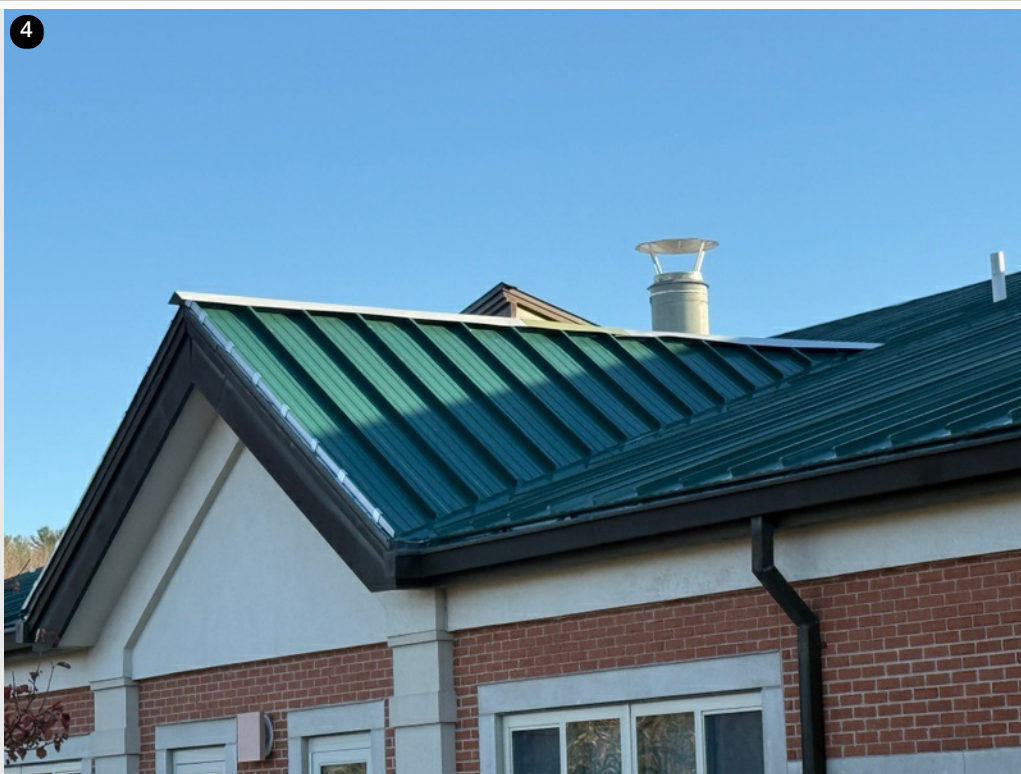
4 Temporary caps installed on all ridges in preparation for incoming rain- 11/20/24
