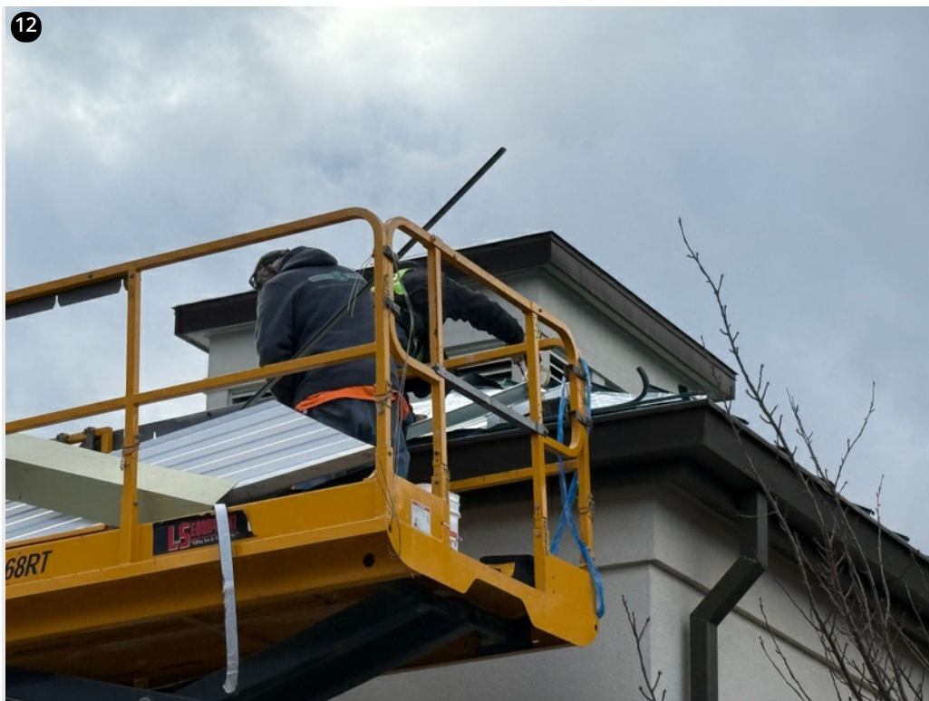
Crew fastening clips on dormer above side entrance- 11/22/24
