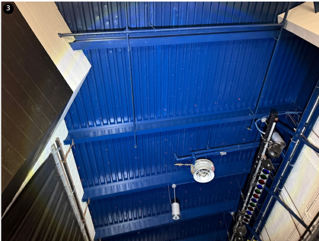
3 Fasteners observed properly penetrating deck- 11/18/24
