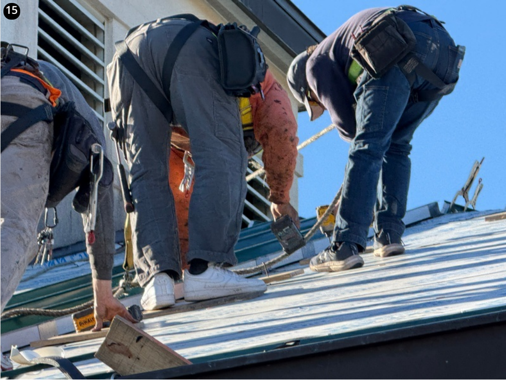
Crew fastening clips using red 8" fasteners- 11/15/24
