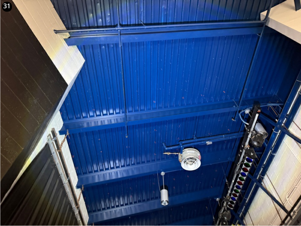
11/18/24- Fasteners visible properly penetrating deck
