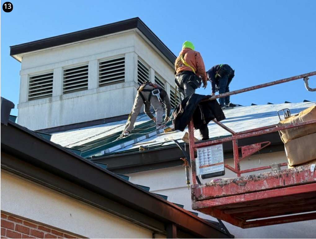
Crew fastening clips using 8" red fasteners- 11/15/24
