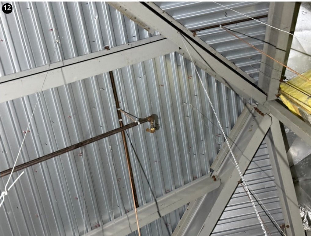
11/14/24- Fasteners observed properly penetrating deck
