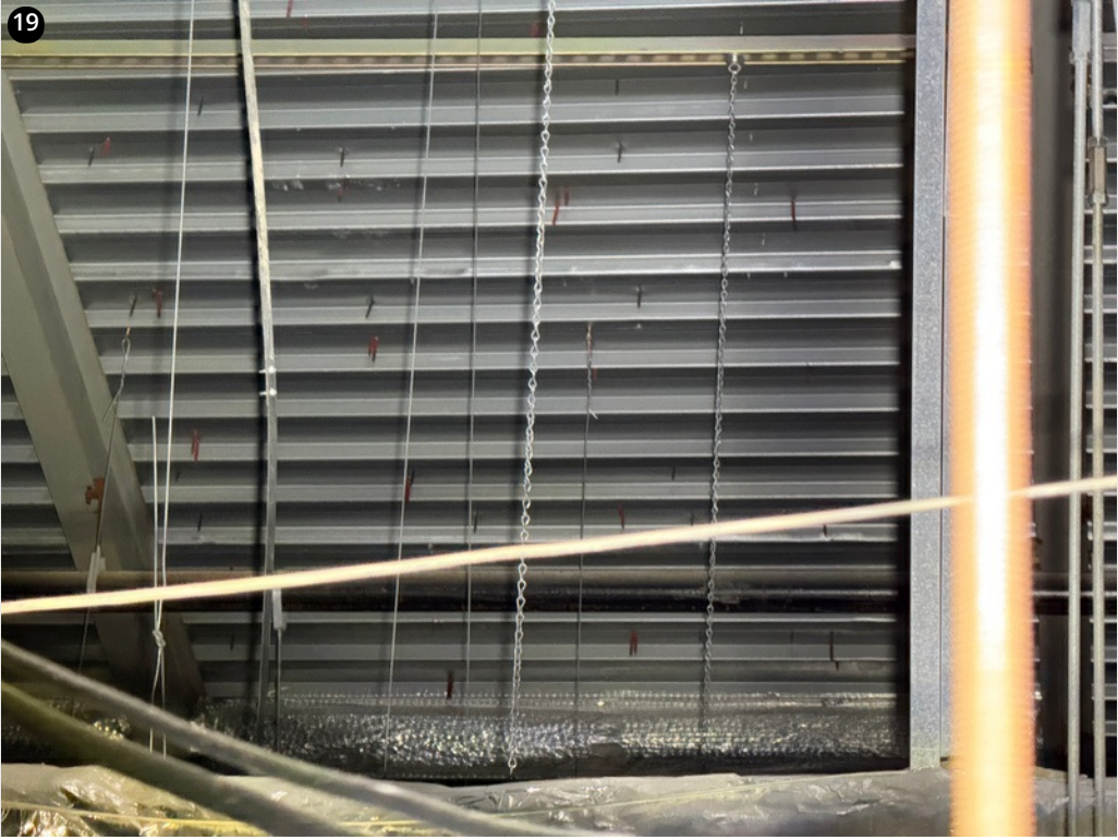
11/15/24- Fasteners observed properly penetrating deck
