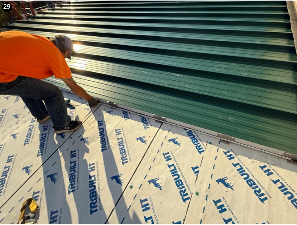
Clips spaced at 1'8" and 2'4" according to zone- 11/18/24
