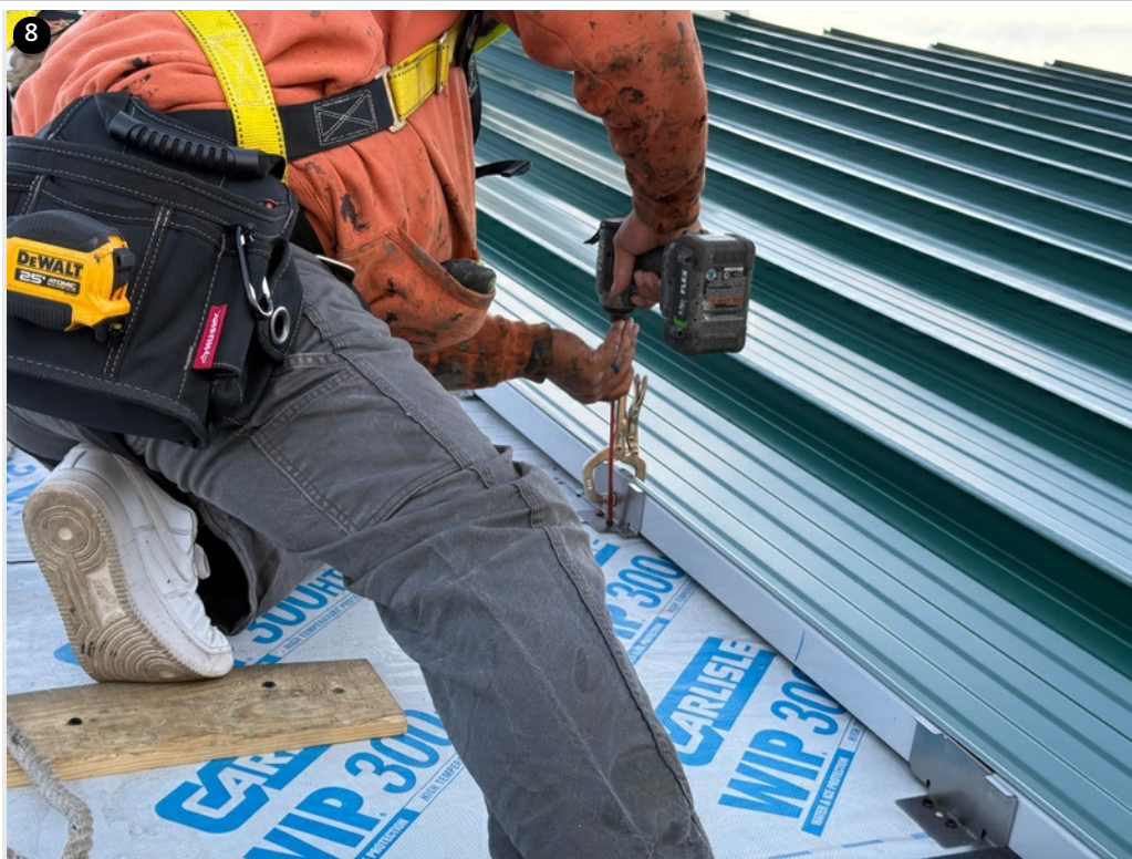
8 Crew fastening clips spaced at 1'8" using 8" red fasteners- 11/14/24
