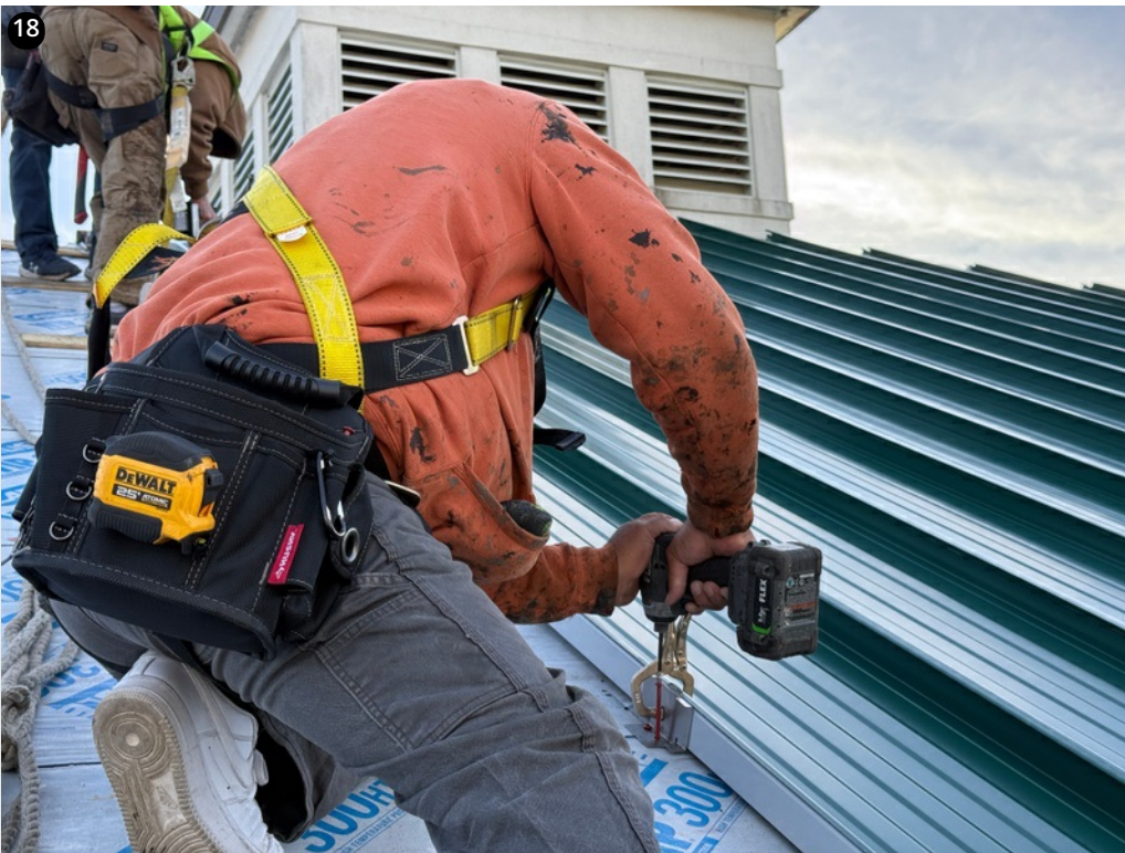
Crew fastening clips using red 8" fasteners
