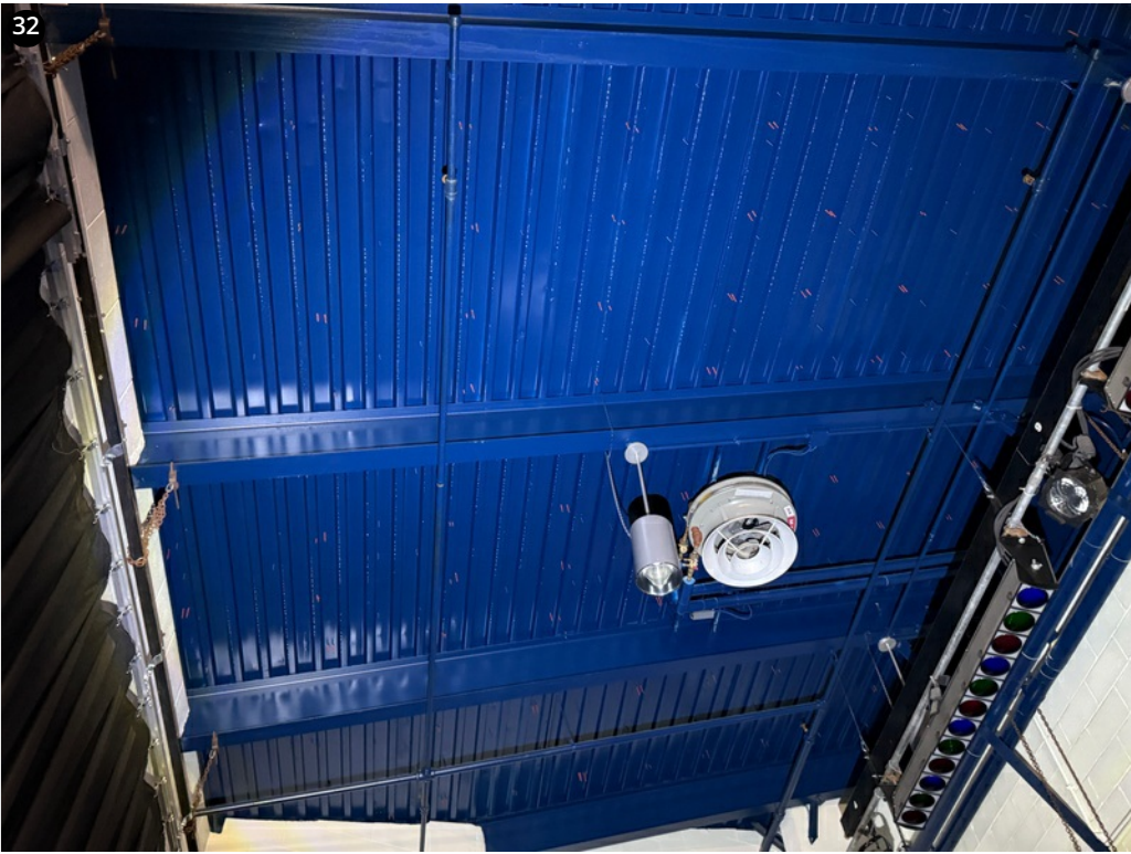
11/18/24- Fasteners observed properly penetrating deck
