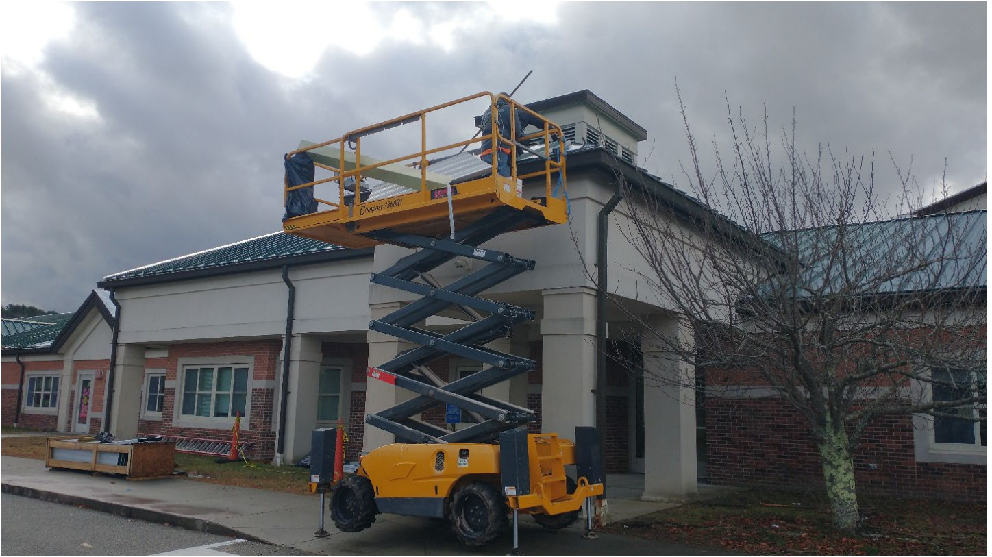
Roof A – North elevation work at time of site visit
