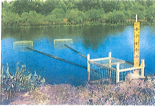
A Double Filter System™ in Virginia, USA. The Beaver Deceiver™ is the first filter and the two Round Fences represent the second filter. The black, plastic pipes in between create dam-leak separation, a powerful concept in thwarting an animal programmed to look for dam leaks in dams.
