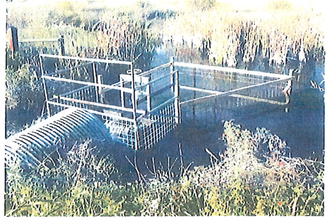
Simple, elegant, and durable, this trapezoidal Beaver Deceiver™ protects an irrigation weir in Colorado, USA.
