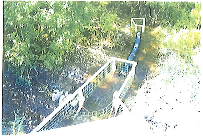
A Double Filter System™ composed of two Beaver Deceivers™. The initial fence has a Turtle Door™ (also used by other animals) on the left side (see photo below). The low, arched fence in the middle guides animals to the hole. The stones at the top prevent beavers from floating debris through the hole and into the culvert.
