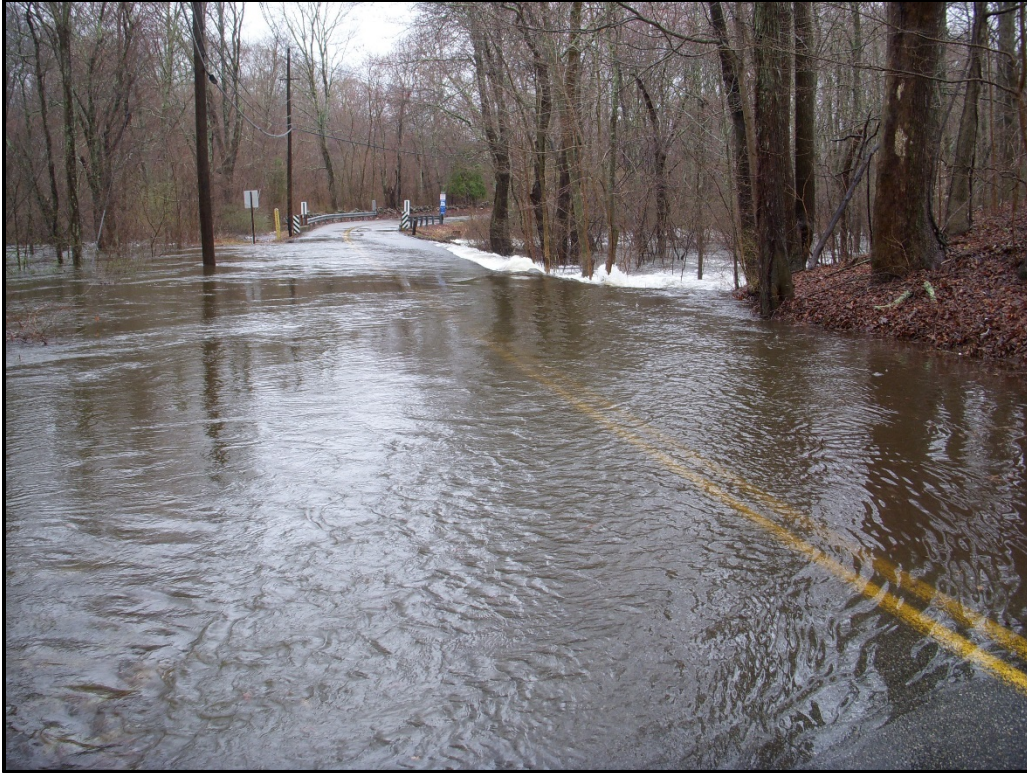
Photo 11- Looking Southerly towards Bridge (3/30/2010)
