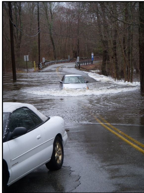
Photo 12- Looking Southerly towards Bridge (3/30/2010)
