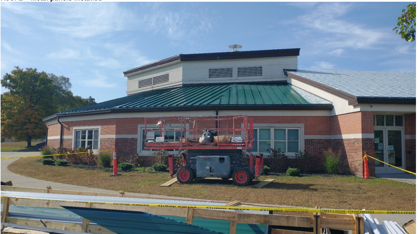
Roof E – Metal panels installed
