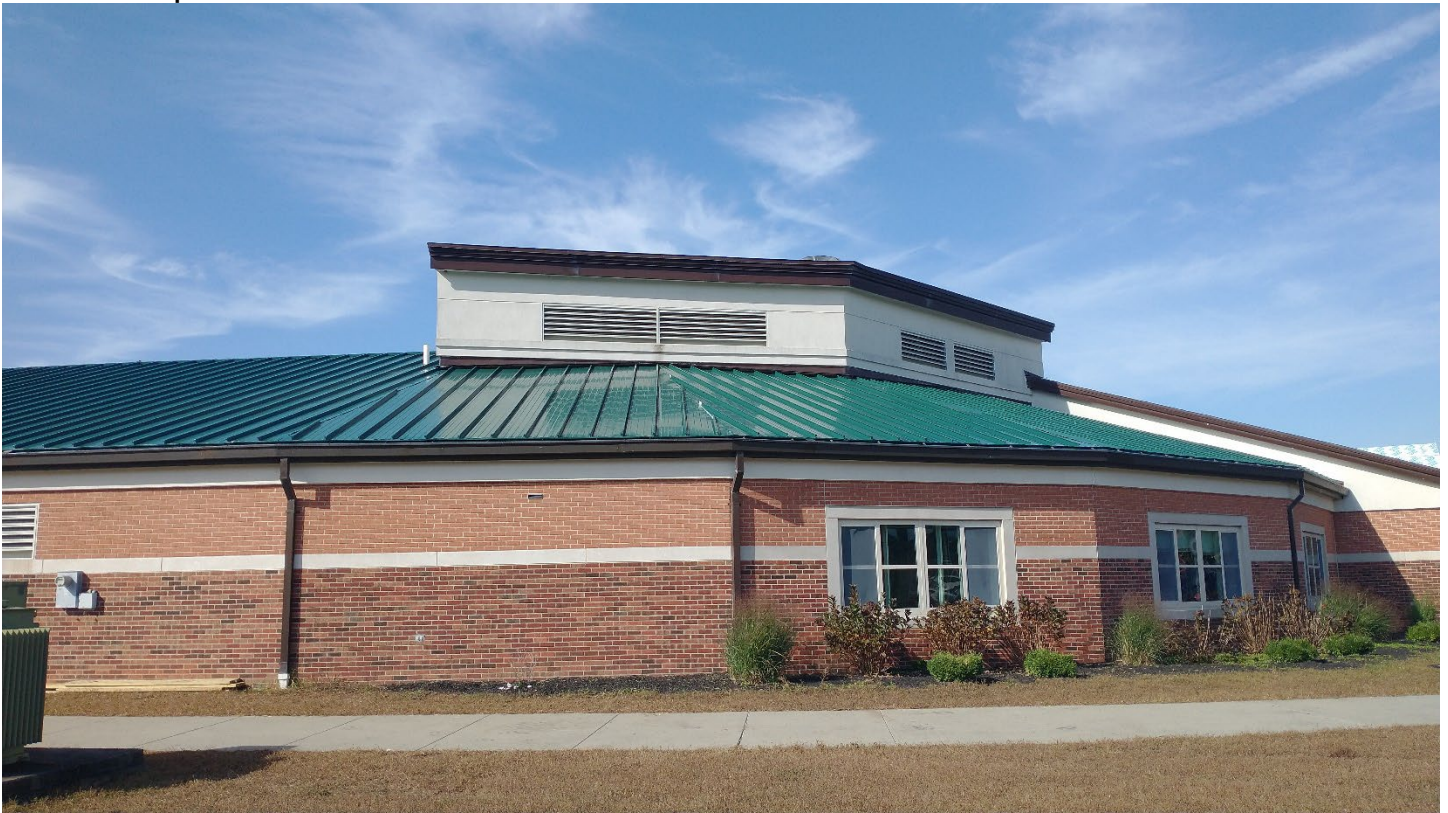
Roof E – Metal panels installed
