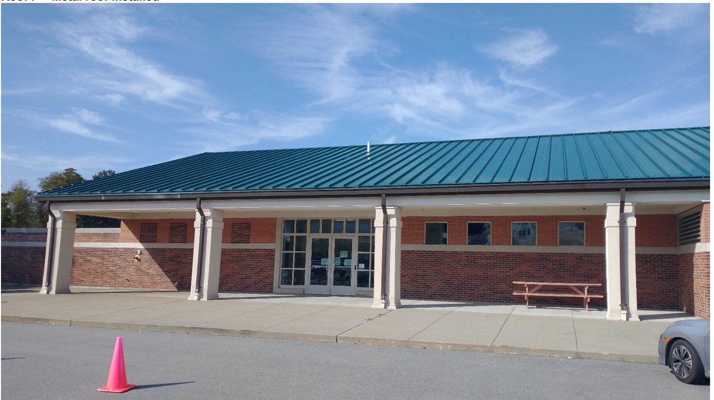
Roof F – Metal roof installed
