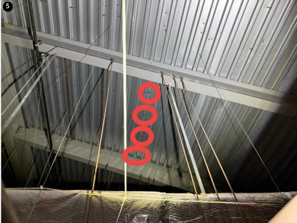
Fasteners visible penetrating deck on Kindergarten wing- 2/4/25
