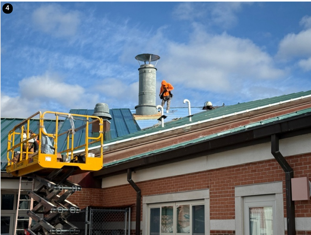
Crew building curb around stack penetration- 2/4/25
