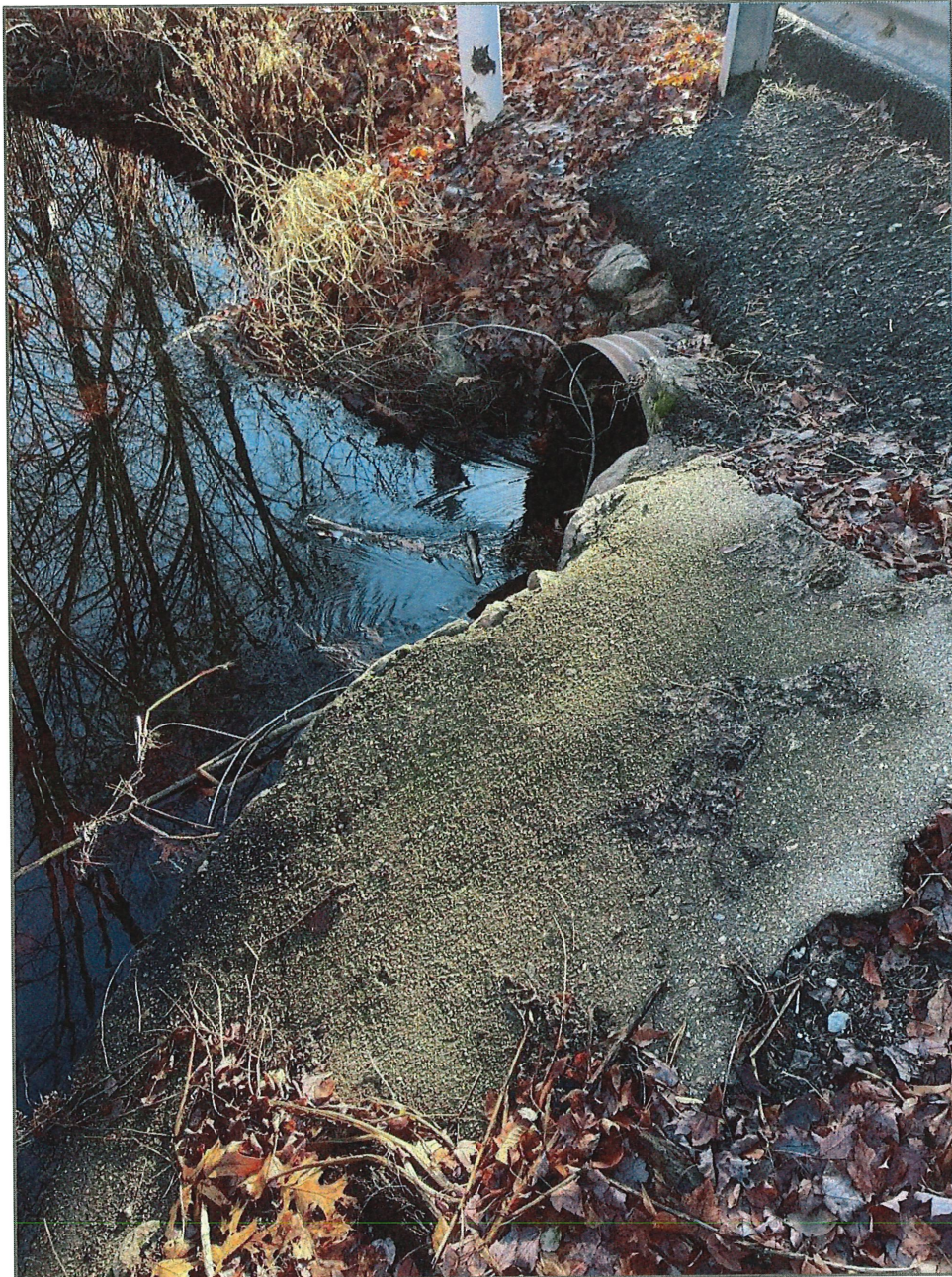
Photo 8: Auxiliary spillway inlet
