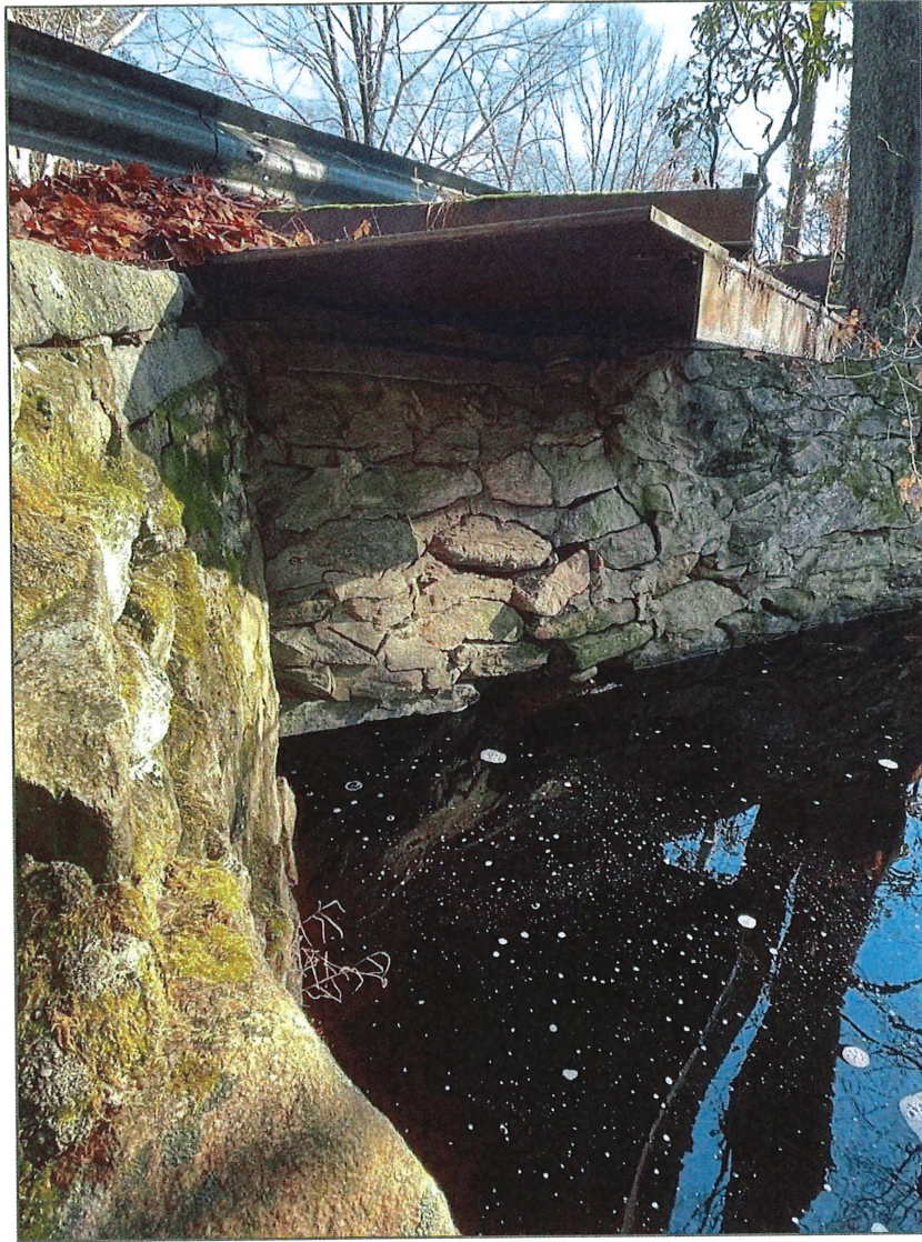
Photo 7: Principal spillway outlet
