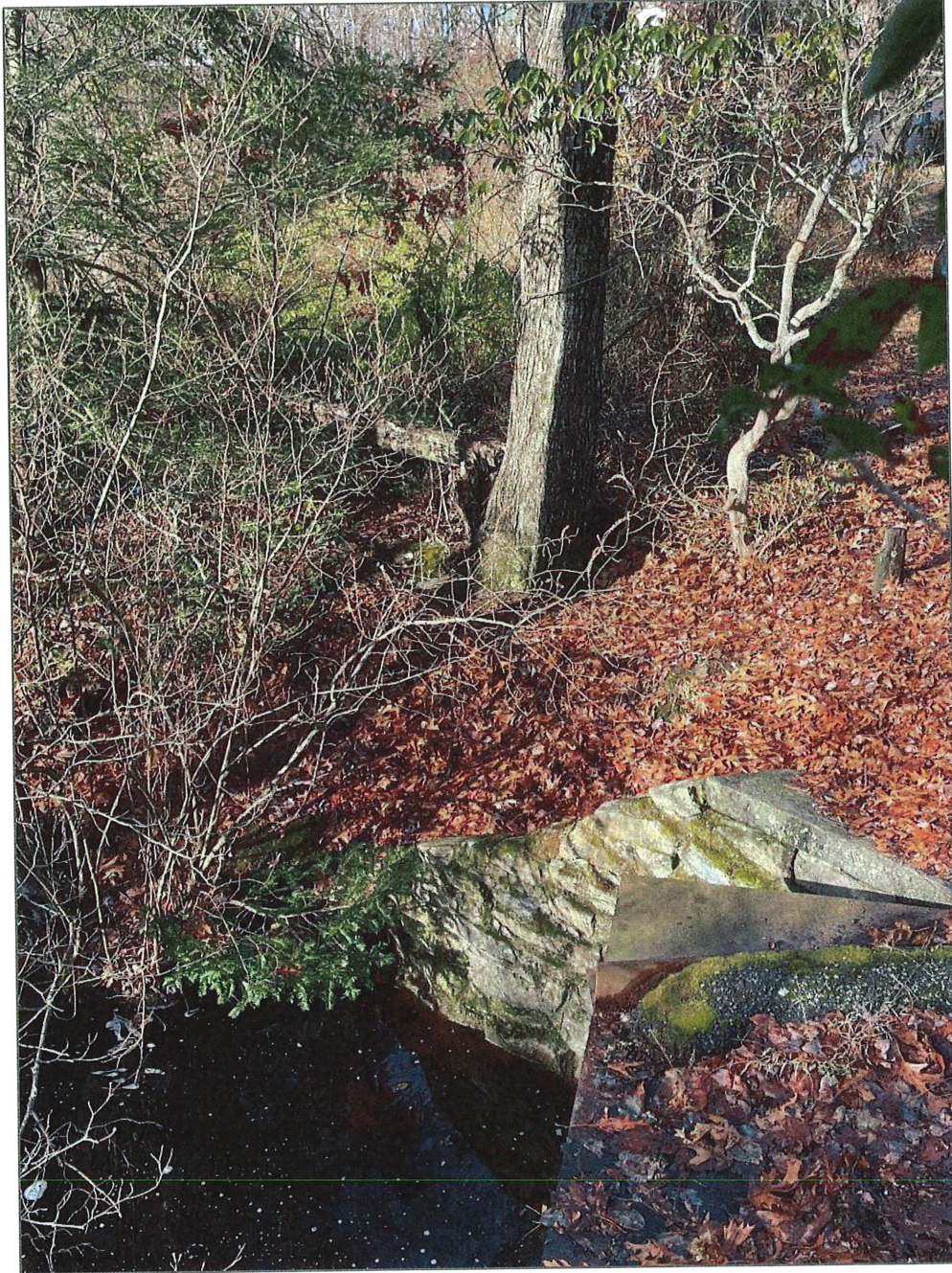
Photo 2: Downstream face of embankment
