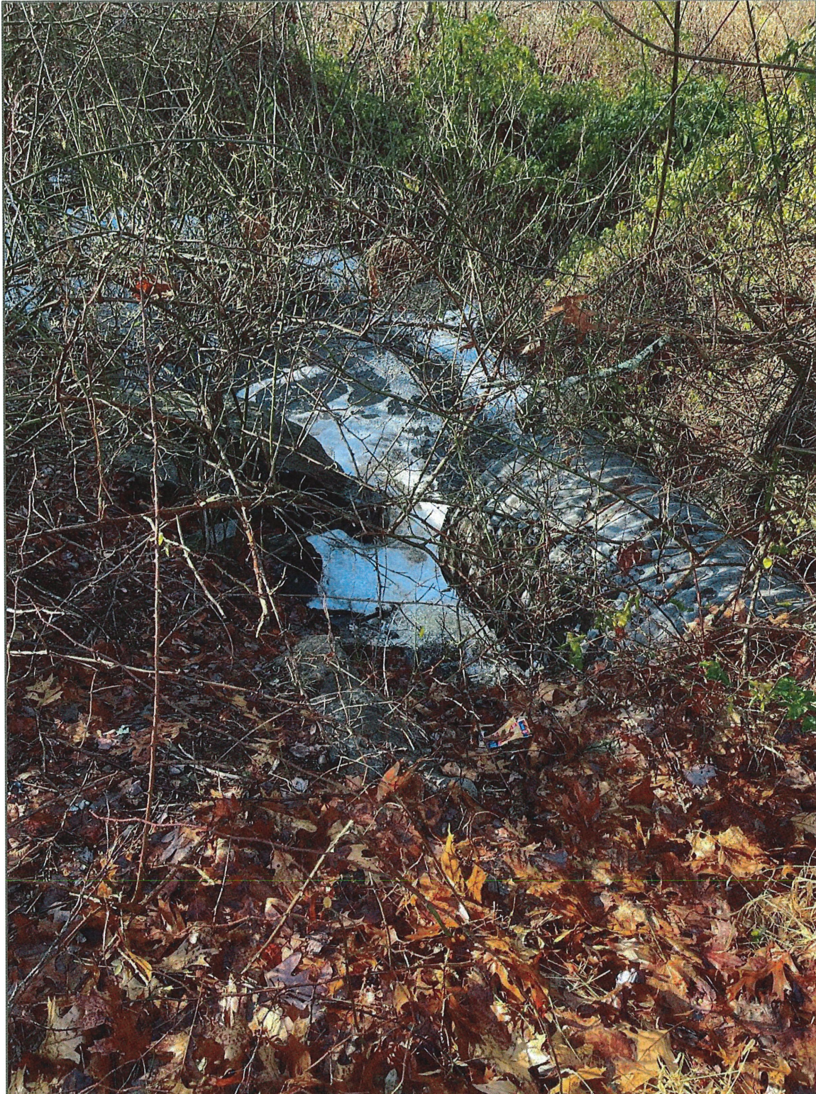
Photo 9: Auxiliary spillway outlet
