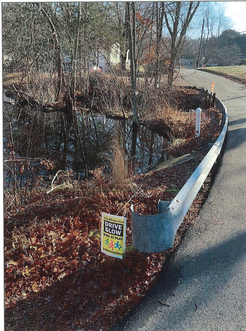
Photo 1: Upstream face of embankment
