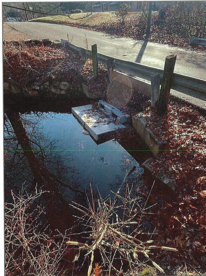
Photo 6: Principal spillway inlet with cover
