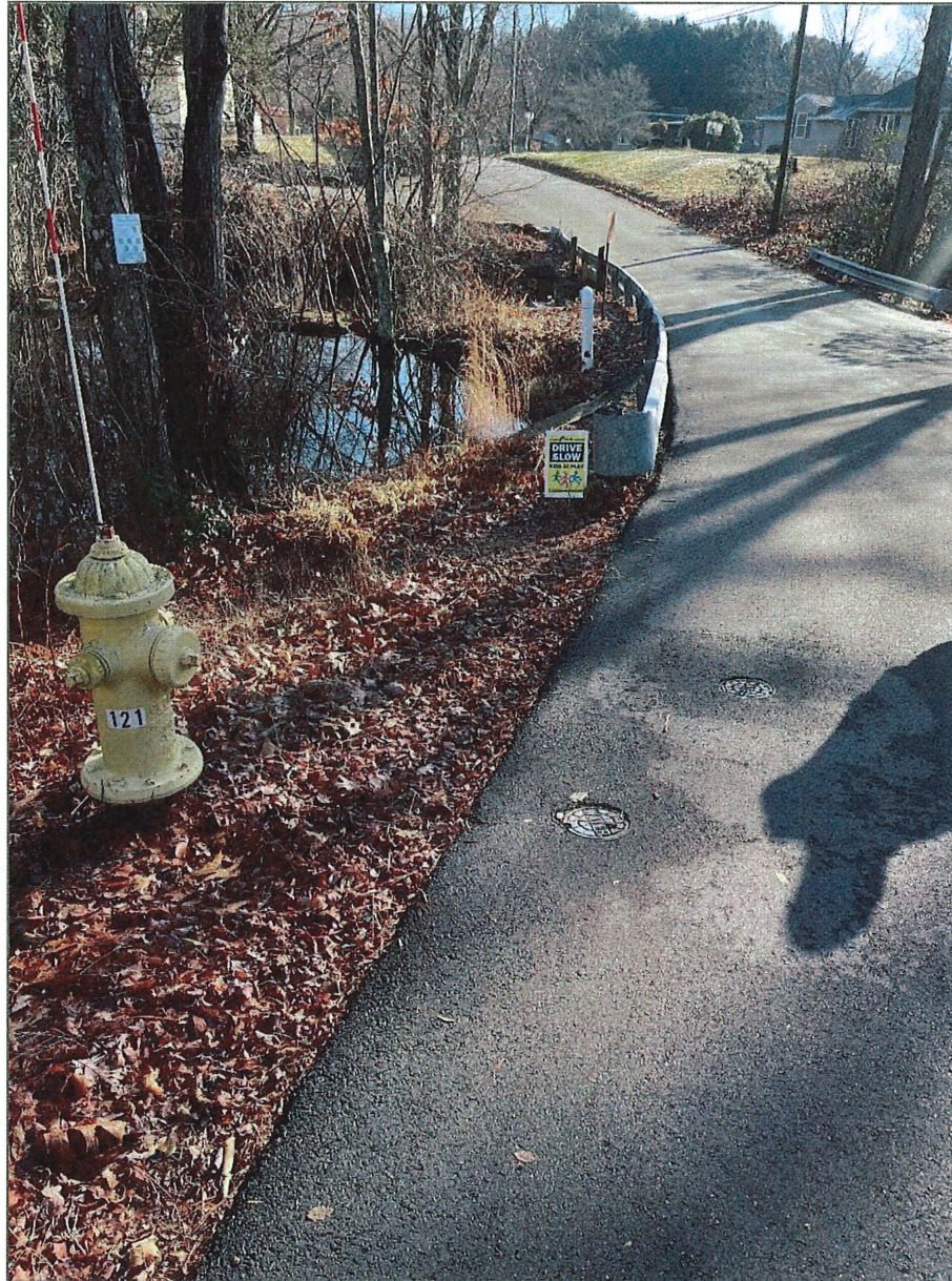
Photo 5: Water shut-off for hydrant and pipe crossing dam. Similar arrangement at left abutment
