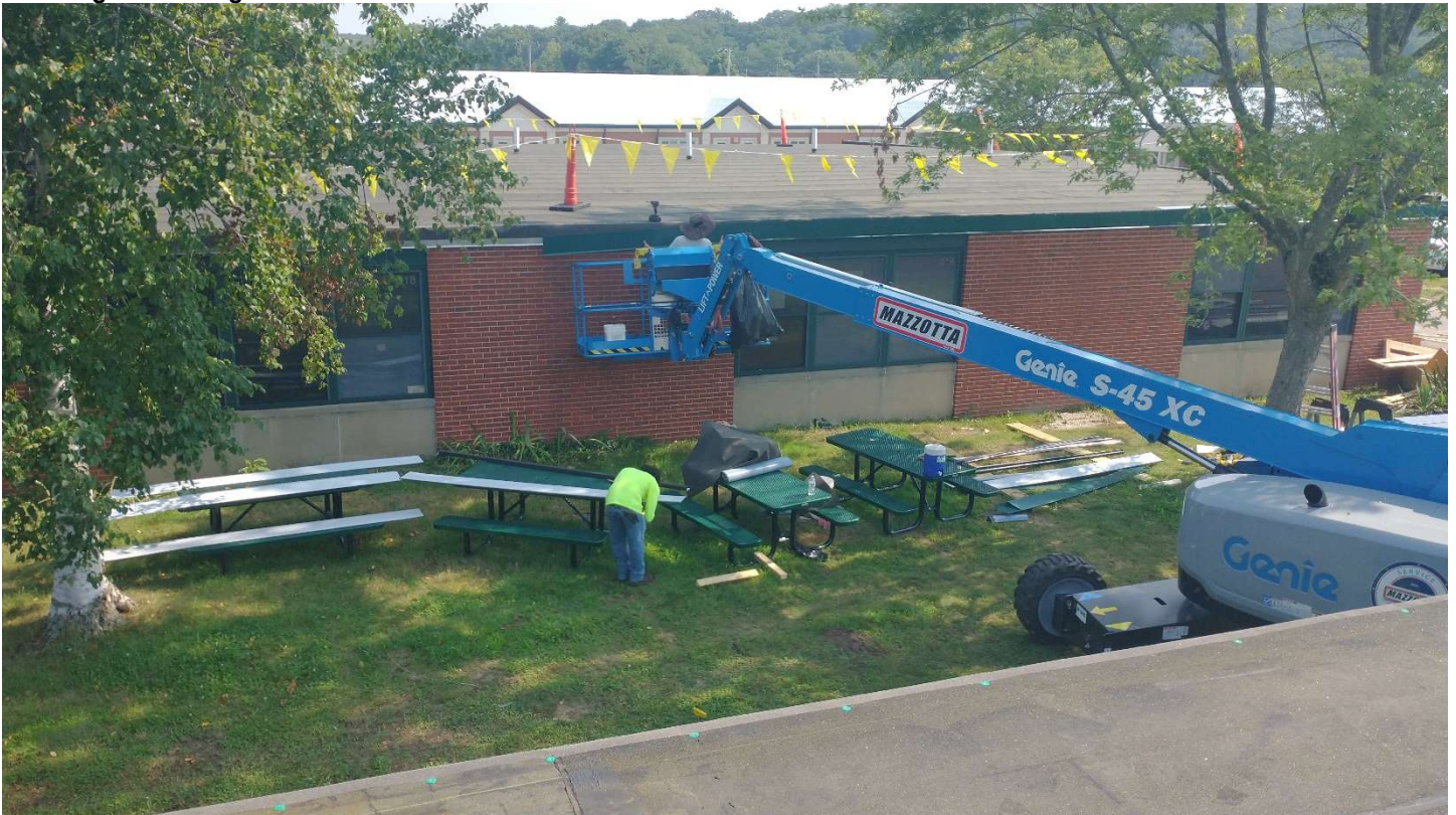
Roof edge trim being installed
