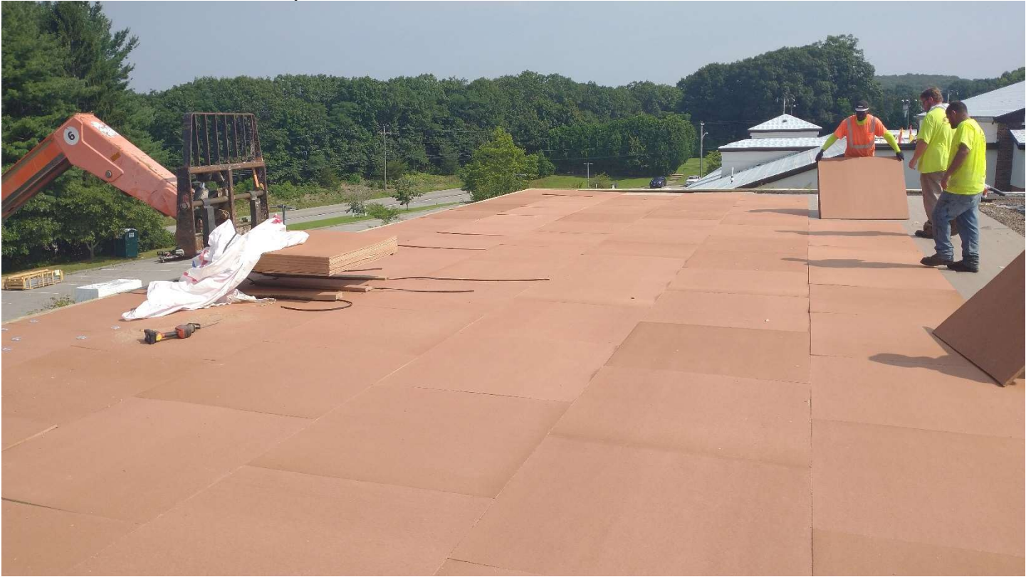
Roof B installation of the insulation panels
