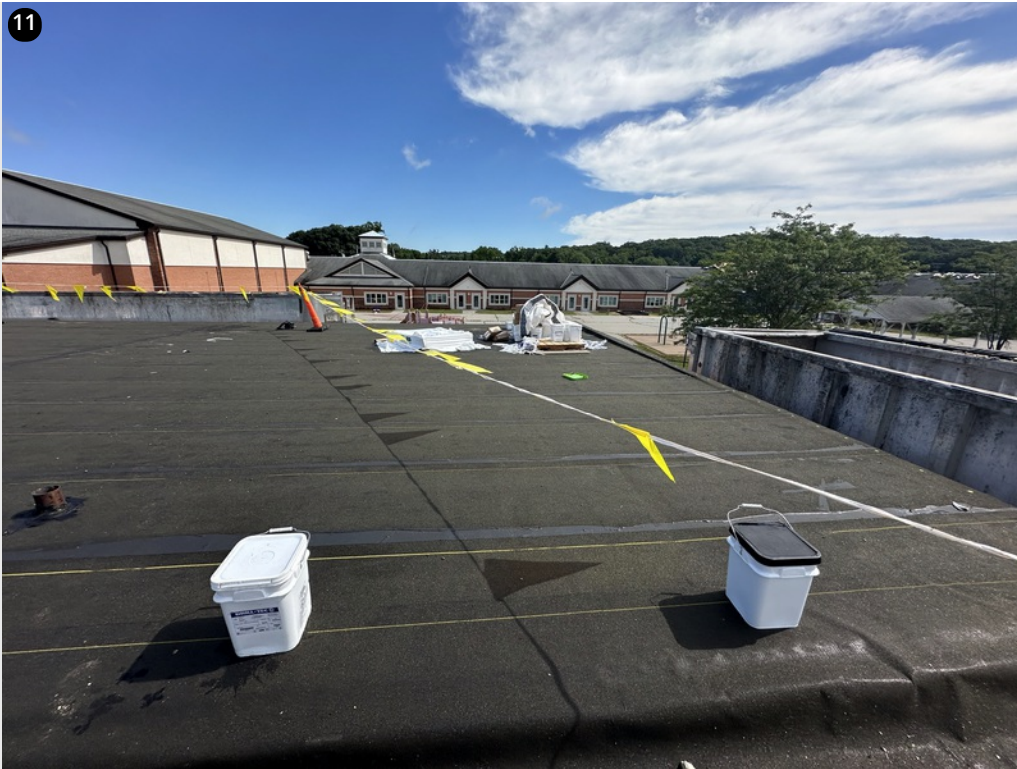
Night tie-ins complete and weighted
