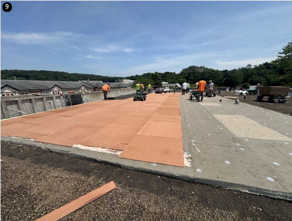
Coverboard being installed over insulation properly
