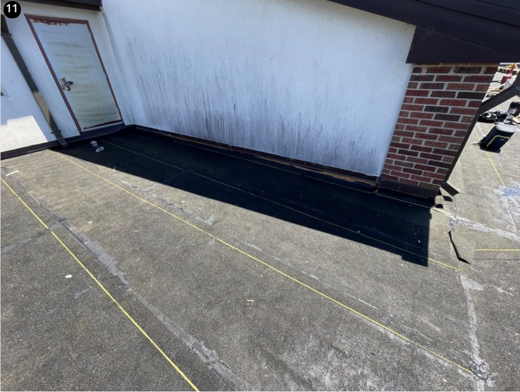
The crew will install the base sheet flashings prior to the cap sheet
