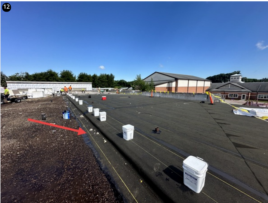
Night tie-ins complete and weighted
