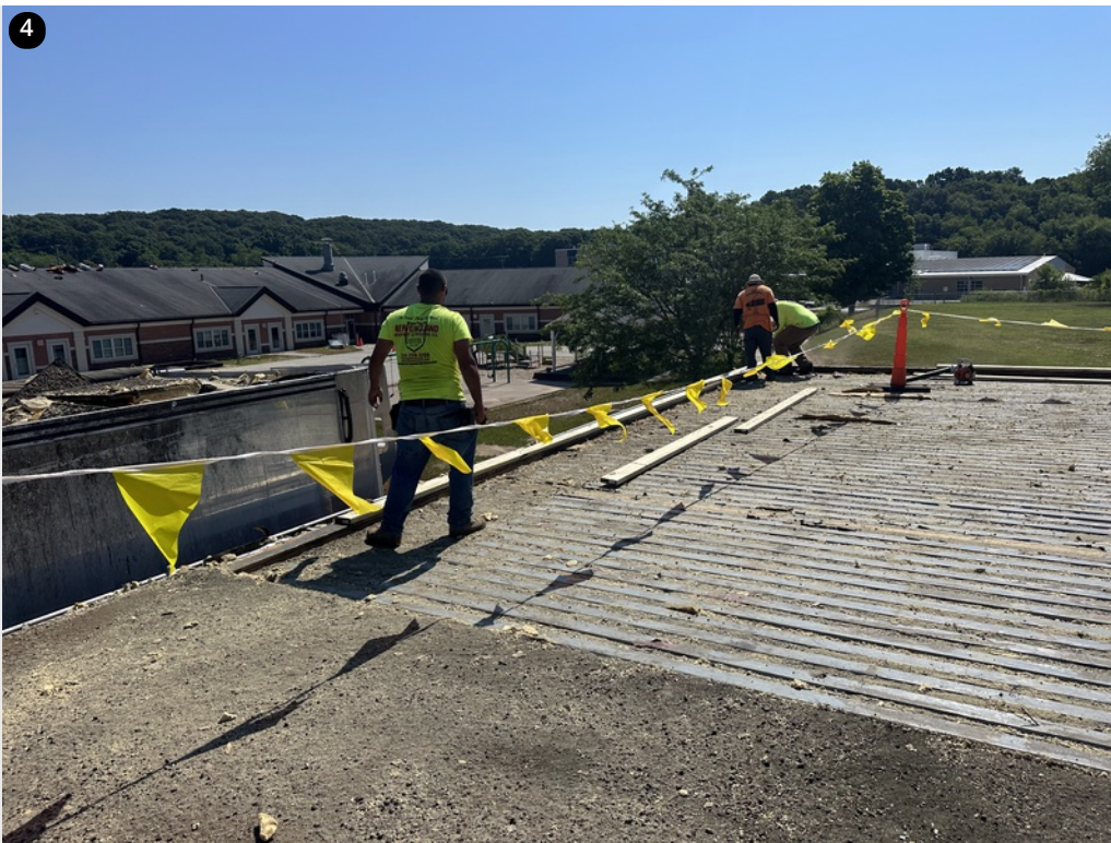
Crew installing pressure treated blocking to accommodate new system layers
