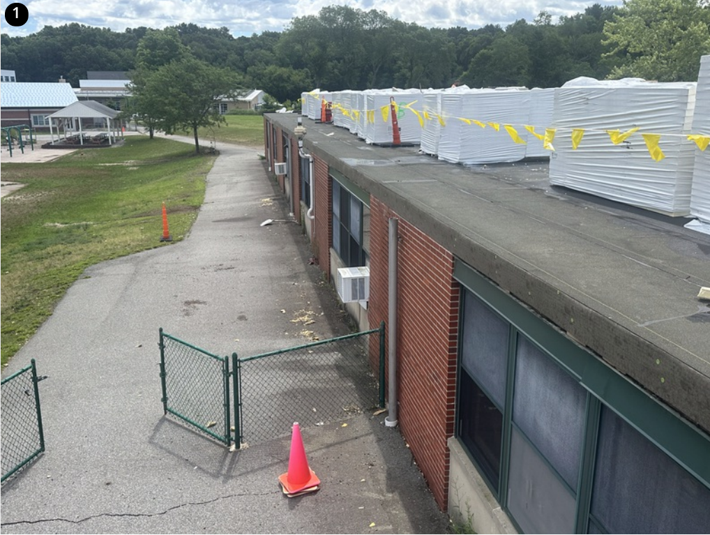
Exposed decking detail on perimeter temporarily fixed- No new leaks have been observed
