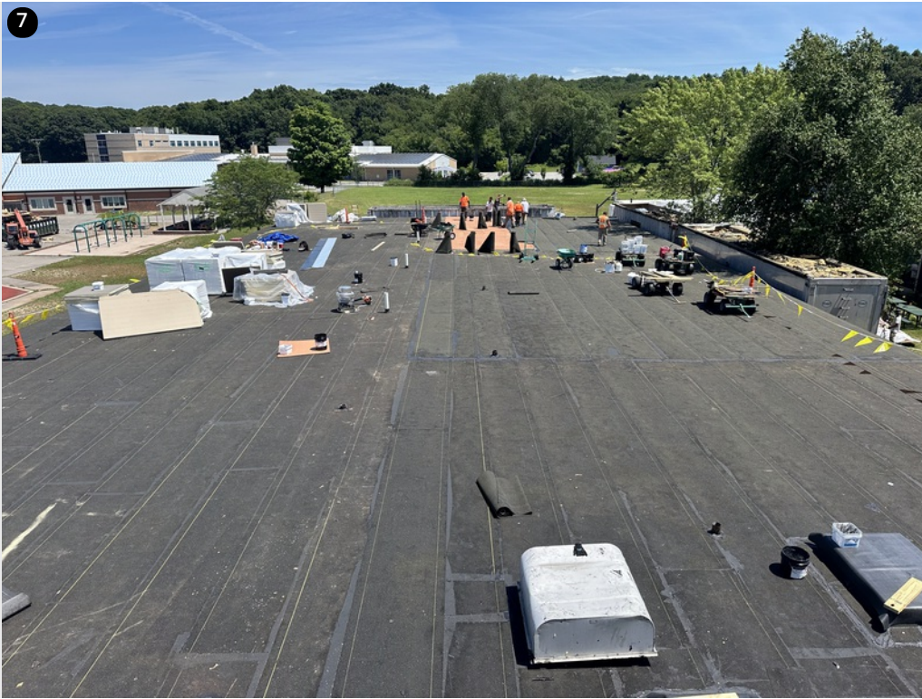
Overview- Crew installing base sheets on final area of playground side
