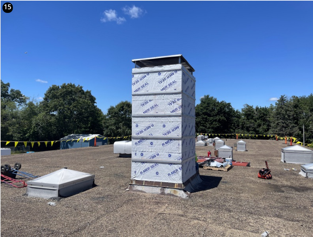
Chimney primed, wrapped and hat channeled
