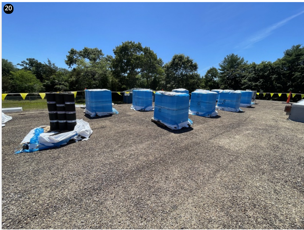
20 Overview - Proper material storage on the roof
