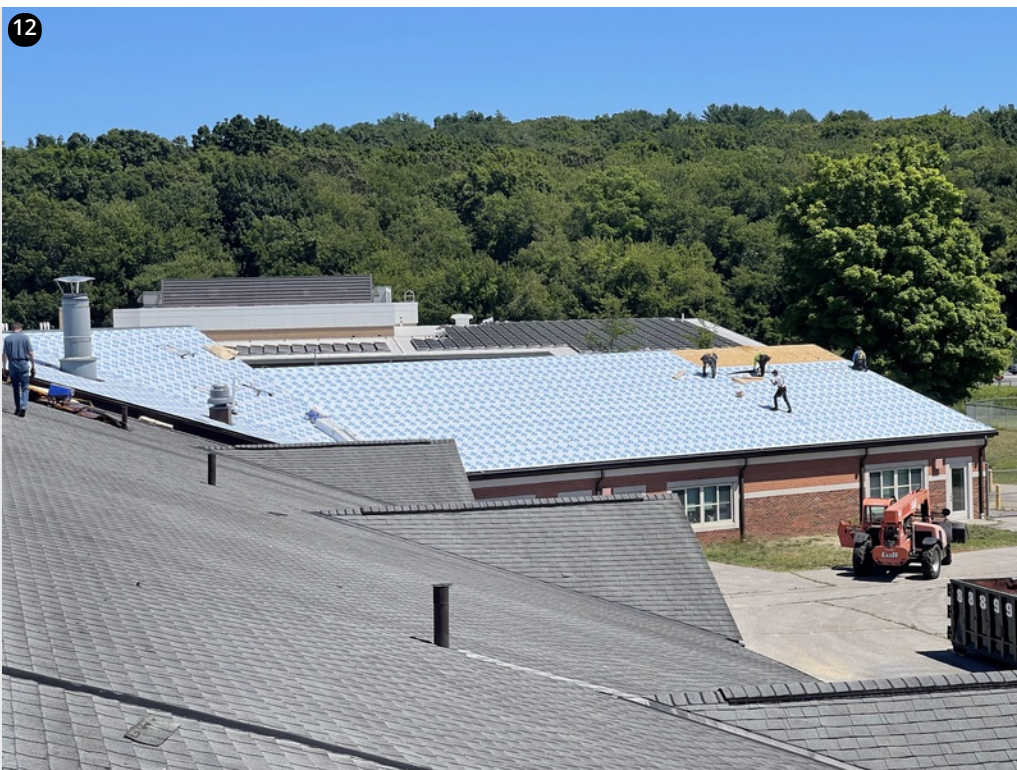
The shingle crew ripped the furthest interior section and finished the valley
