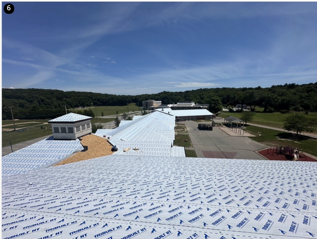
Overview- 99% completed ice and water installation
