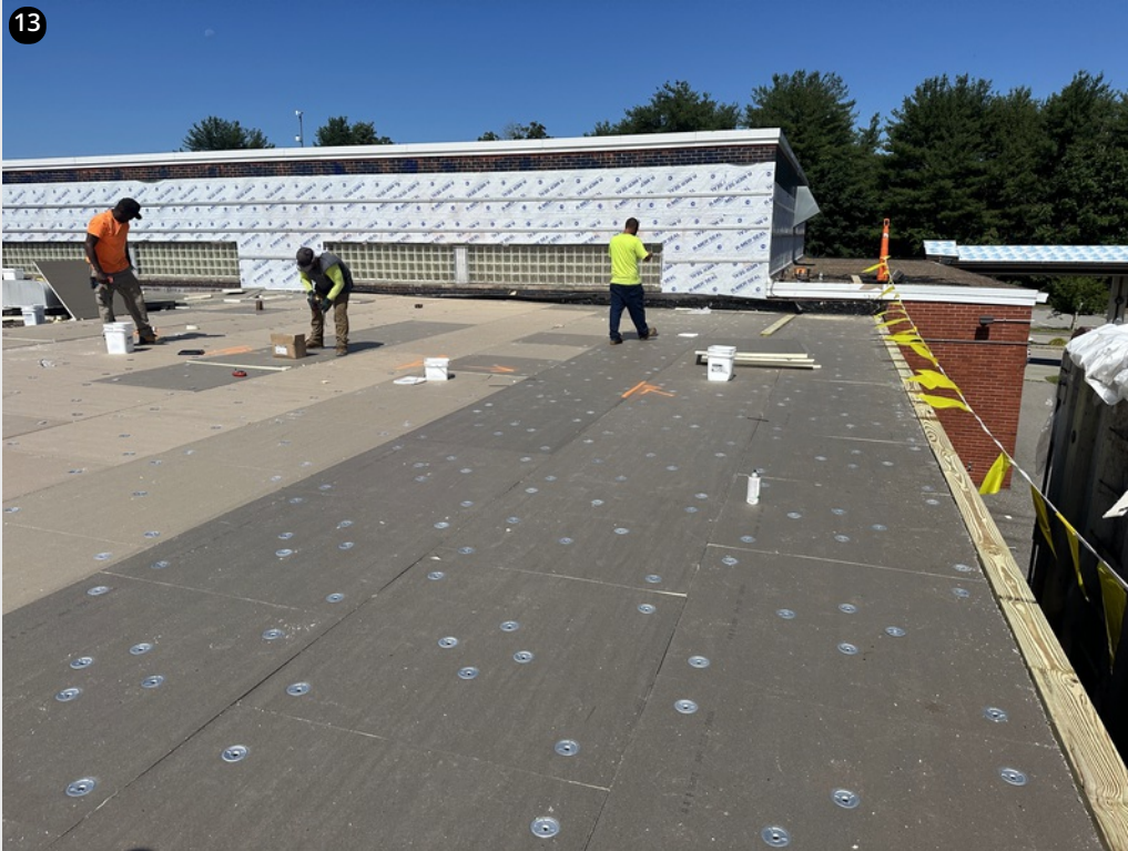
Section closest to the cafeteria - Insulation installed
