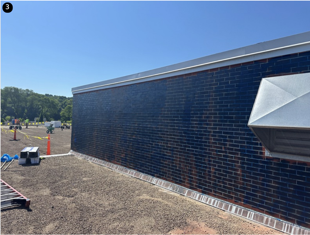
Primed masonry wall
