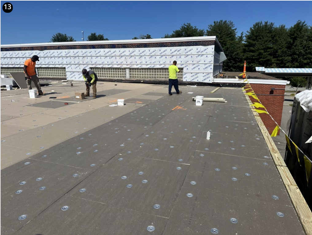
Section closest to the cafeteria - Insulation installed
