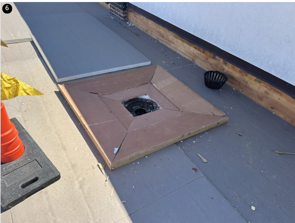
Drain sump built up with insulation
