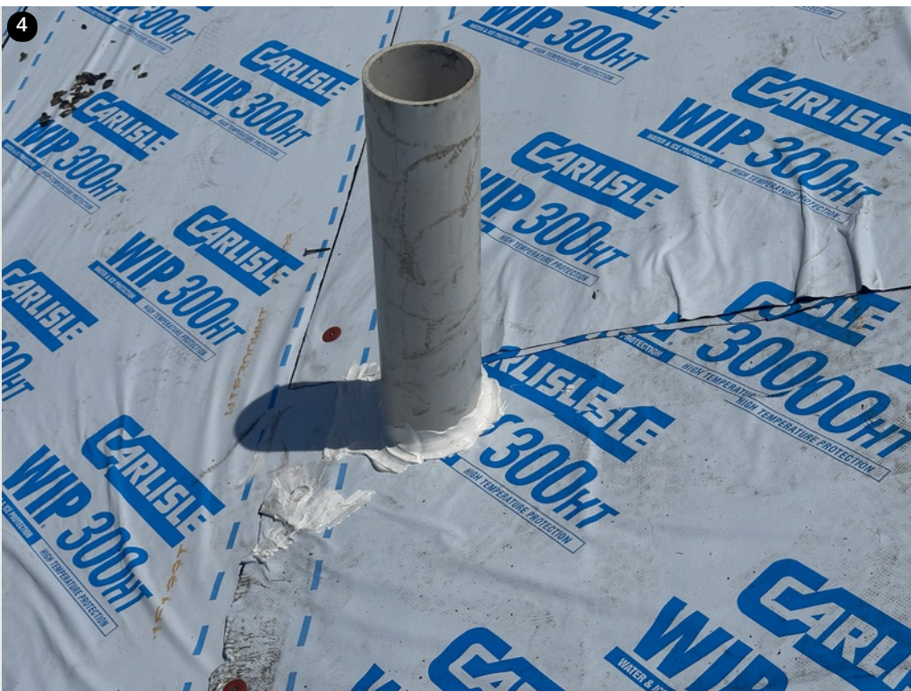
All penetrations tied into ice and water layer using proper sealant
