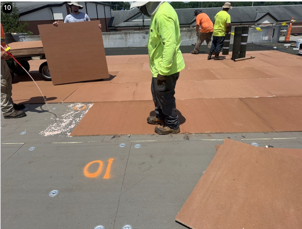
Coverboard being installed in foam adhesive as specified
