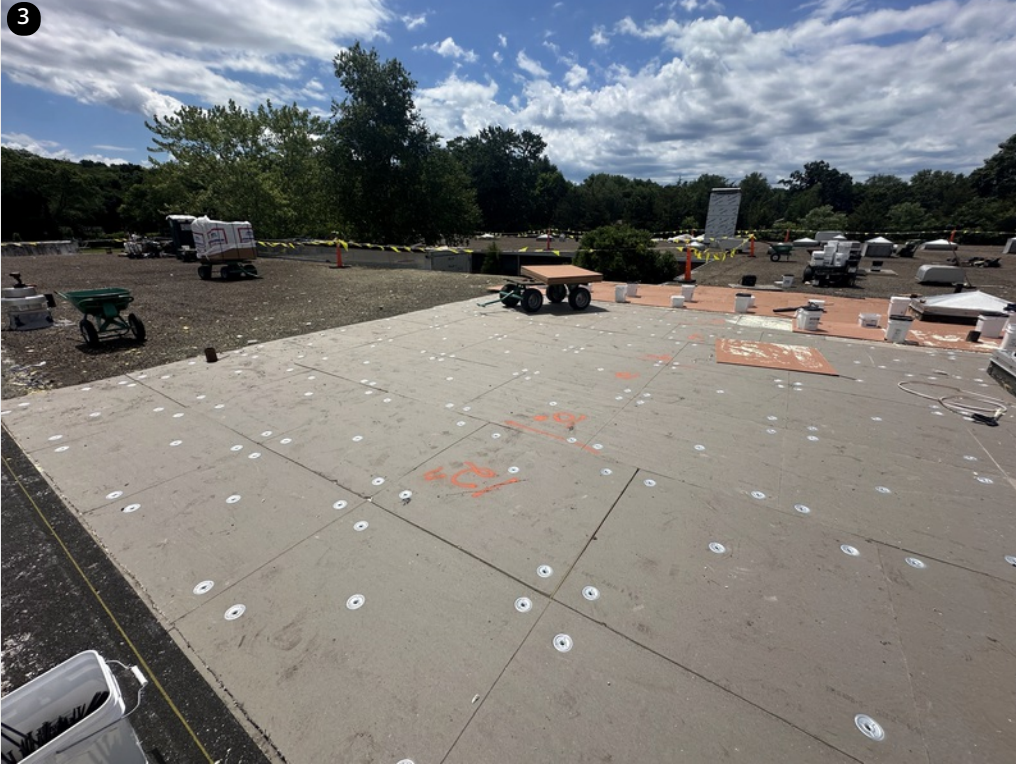
Overview- Fastening pattern on insulation boards
