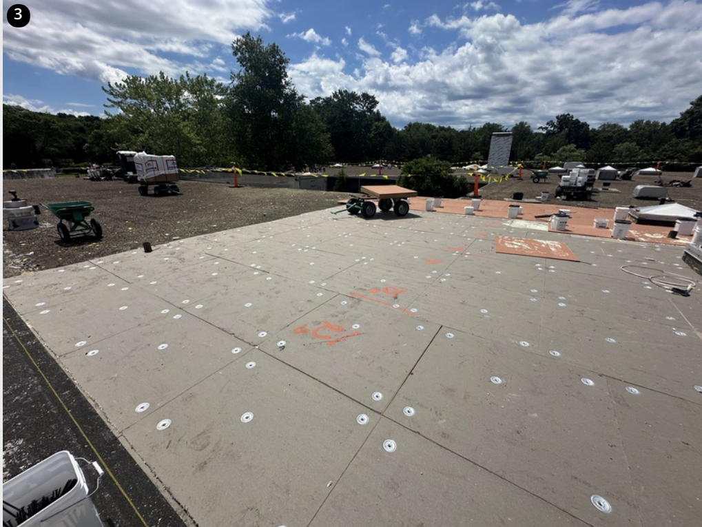
Overview- Fastening pattern on insulation boards
