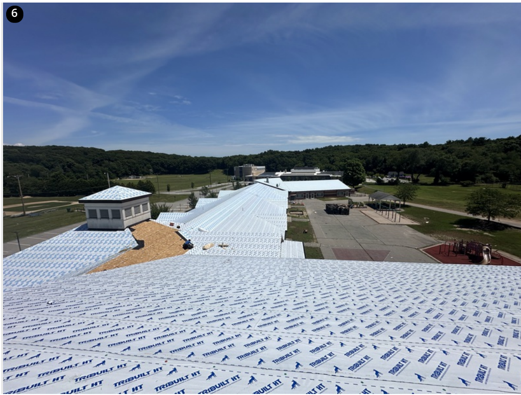
Overview- 99% completed ice and water installation
