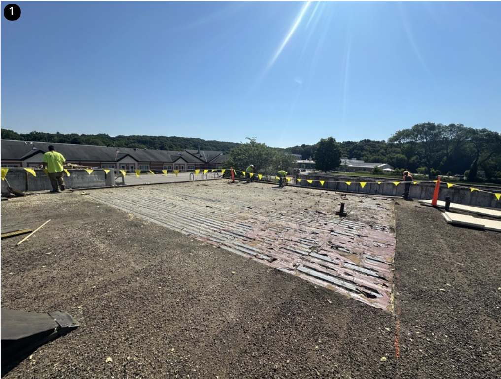
First area ripped to metal deck
