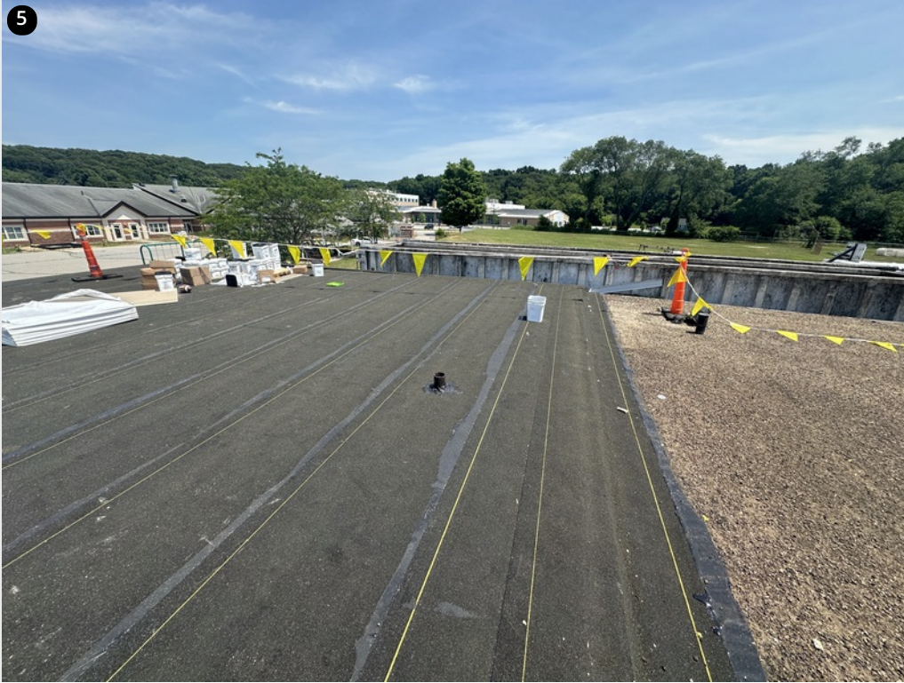
Base sheets installed over insulation and coverboard- Good bleed out at lap seams
