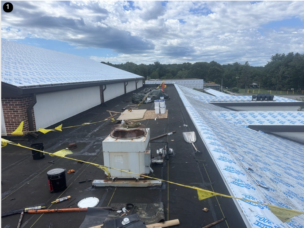
Overview- Completed base sheets on low slope area
