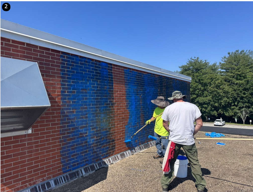
Crew applying primer to masonry wall in preparation for ice and water layer
