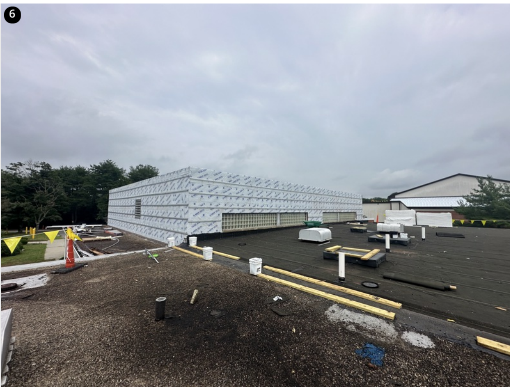
Masonry wall completely covered with ice and water- Hat channels installed
