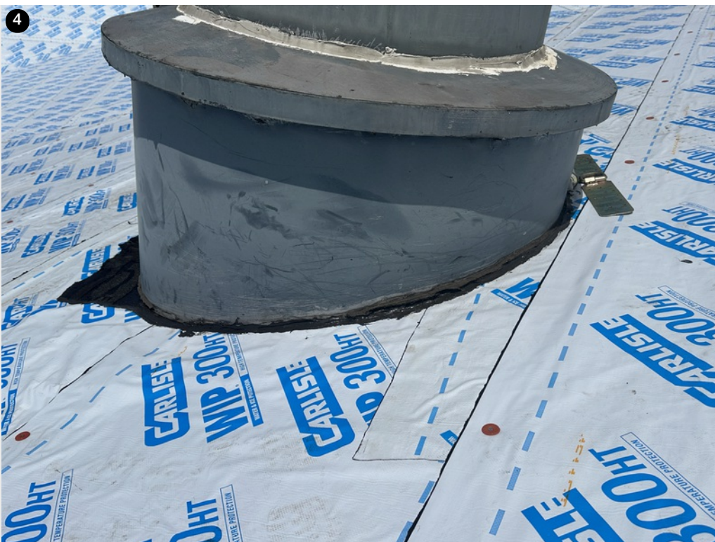
All penetrations tied into ice and water layer with appropriate sealant
