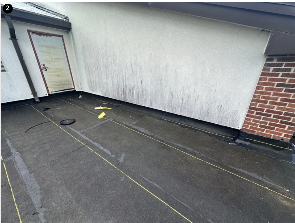
Completed base sheets near roof access door- Great bleedout at lap seams- Completed base flashing plys
