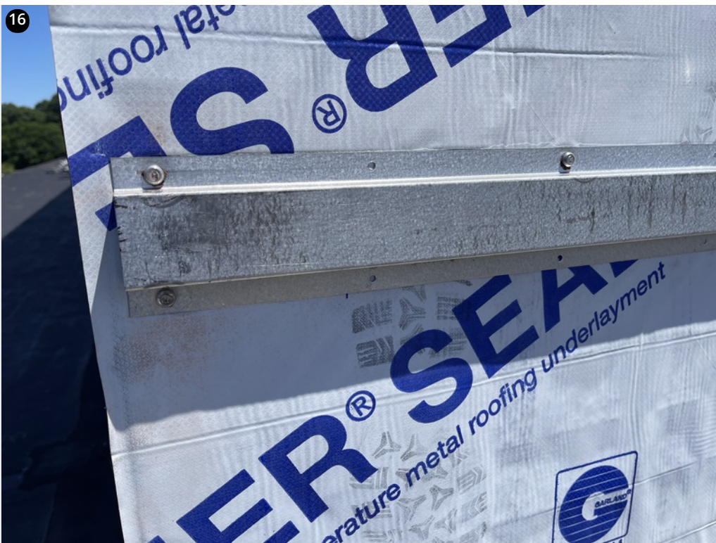
Hat channels for wall panels installed properly
