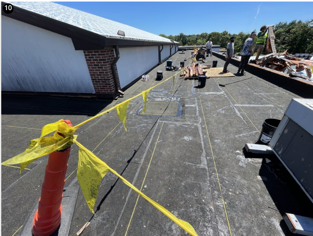
Low slope roof section base sheet is completed and drains are temped in
