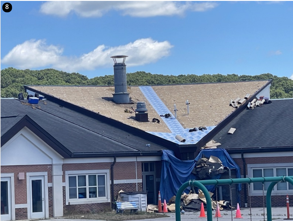
Valley section ripped to deck- Valley reinforced with ice and water layer
