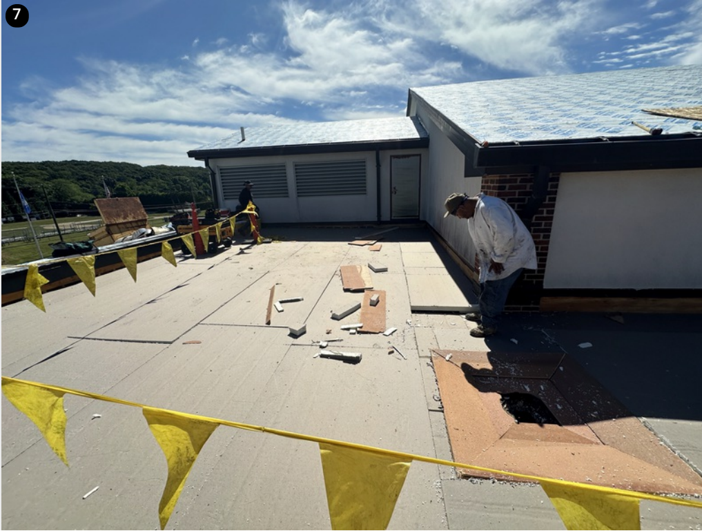
Insulation laid out on ripped EPDM section
