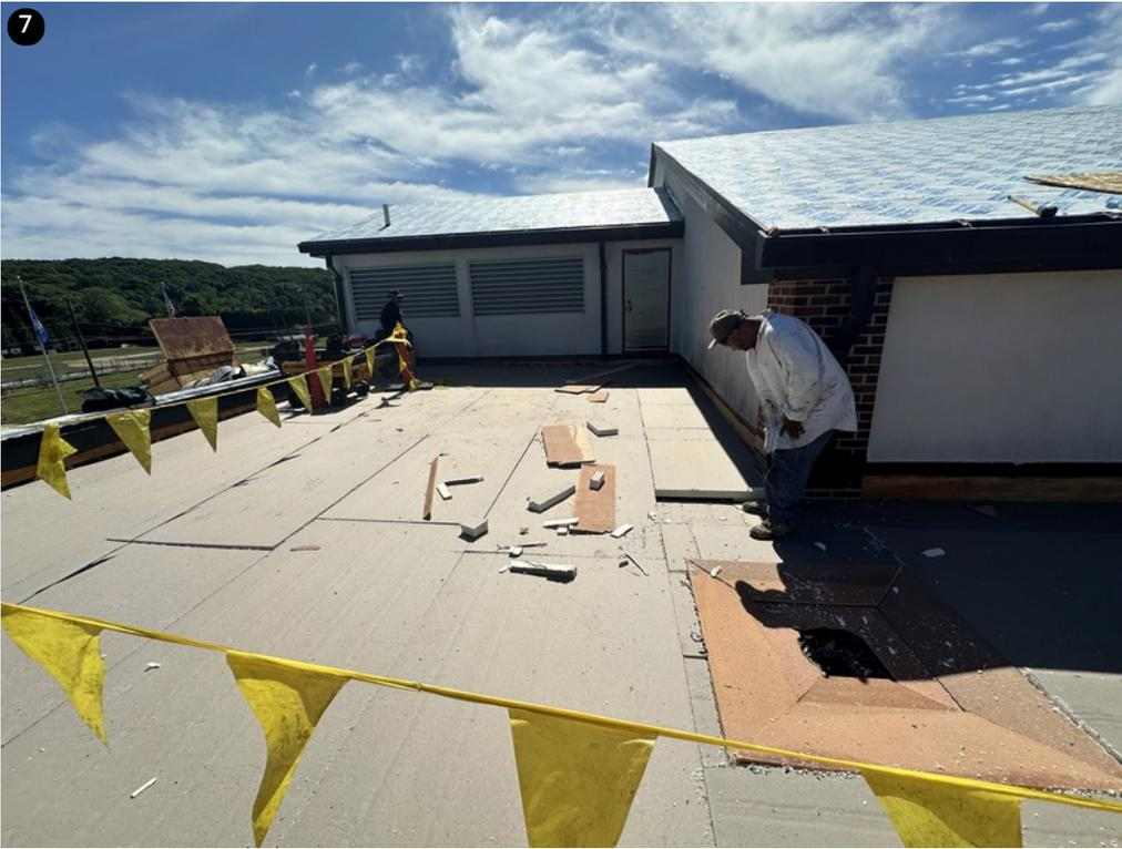
Insulation laid out on ripped EPDM section
