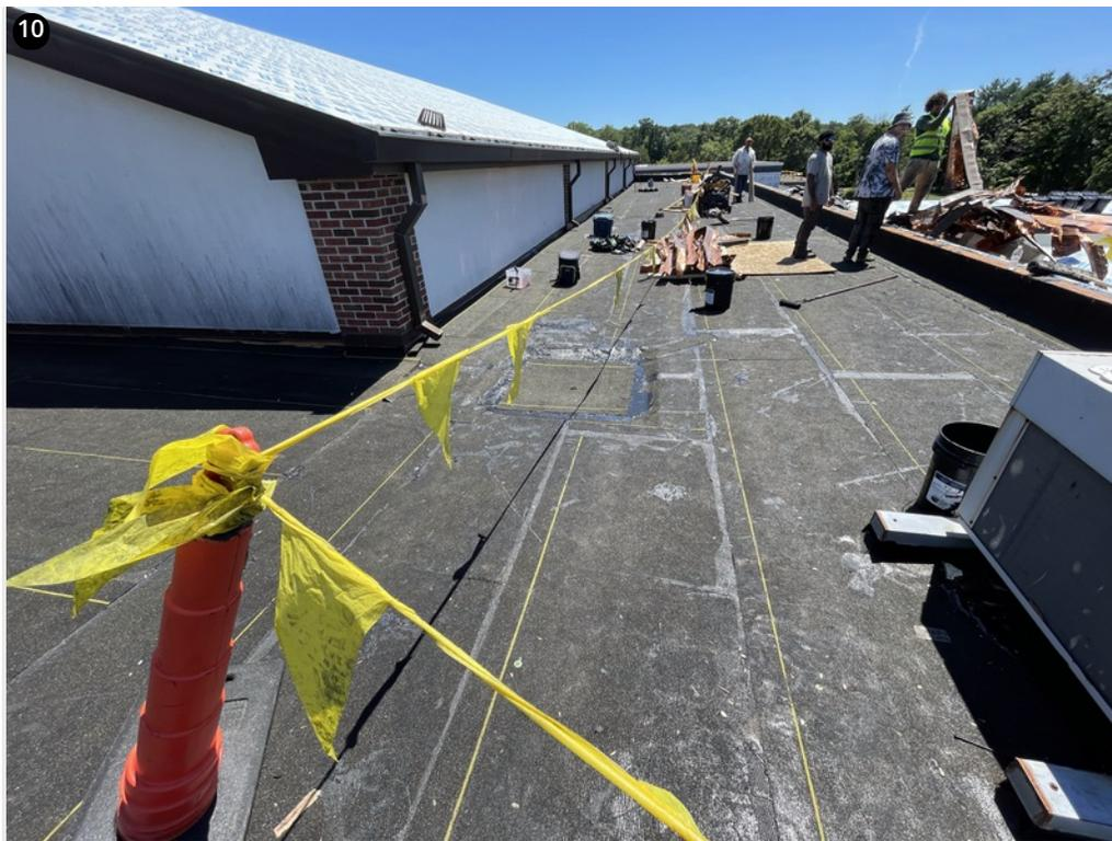
10 Low slope roof section base sheet is completed and drains are temped in
