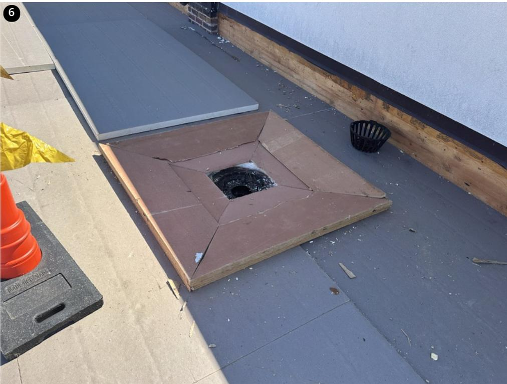
Drain sump built up with insulation
