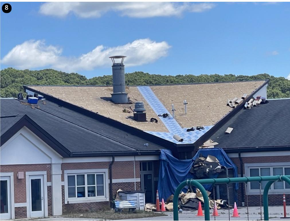
Valley section ripped to deck- Valley reinforced with ice and water layer
