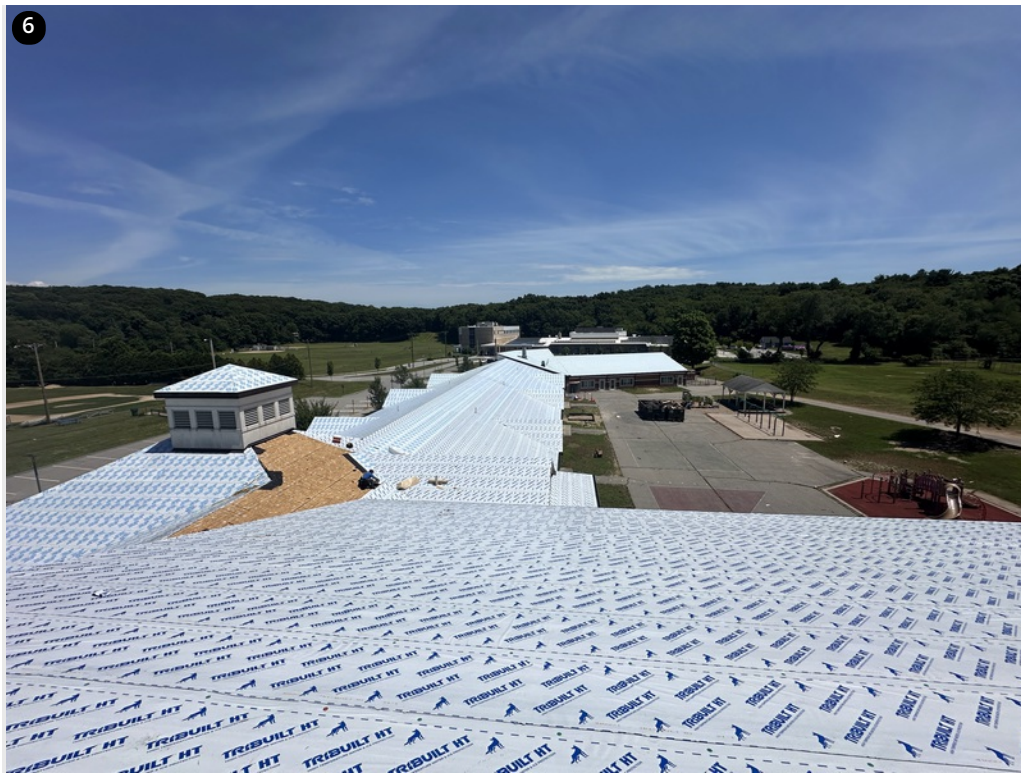
Overview- 99% completed ice and water installation
