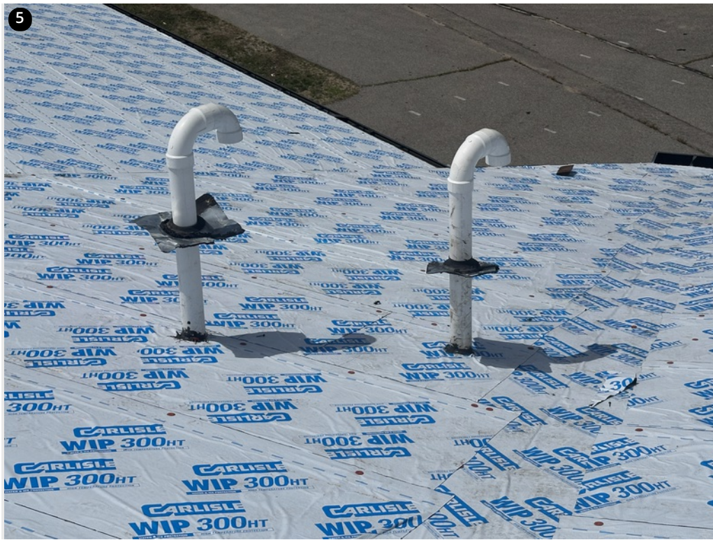
Ice and water layer installed under existing vent pipe flange
