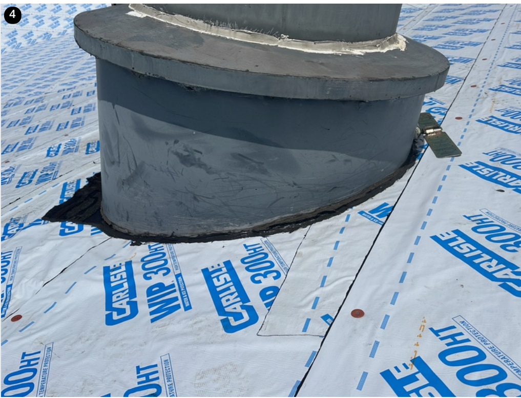
All penetrations tied into ice and water layer with appropriate sealant
