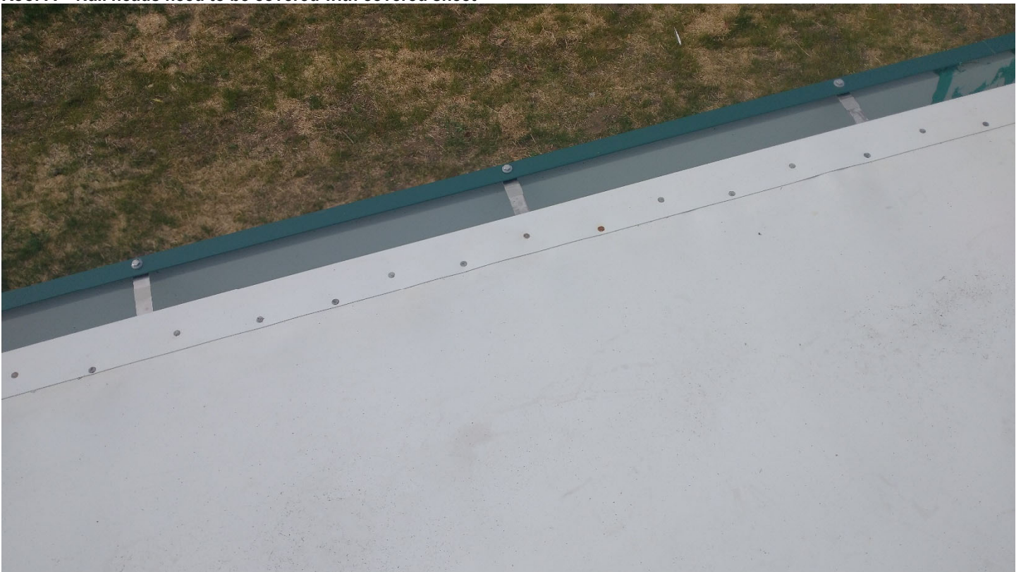
Roof A – Nail heads need to be covered with covered sheet
