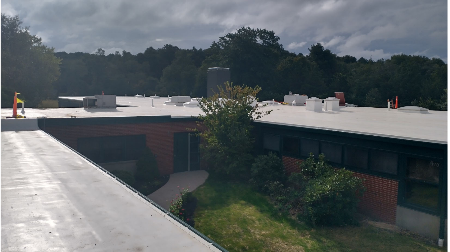
Roof A – Looking northwest
