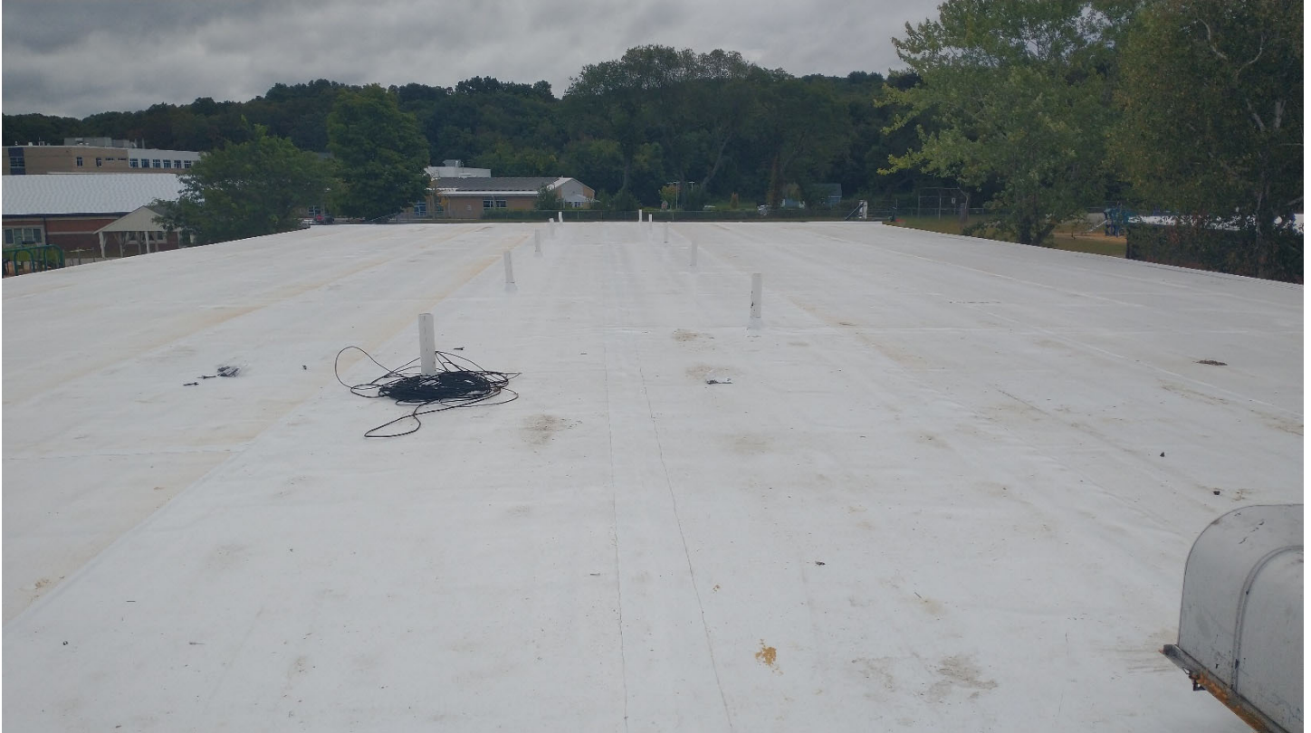
Roof A – Nail heads need to be covered with covered sheet
