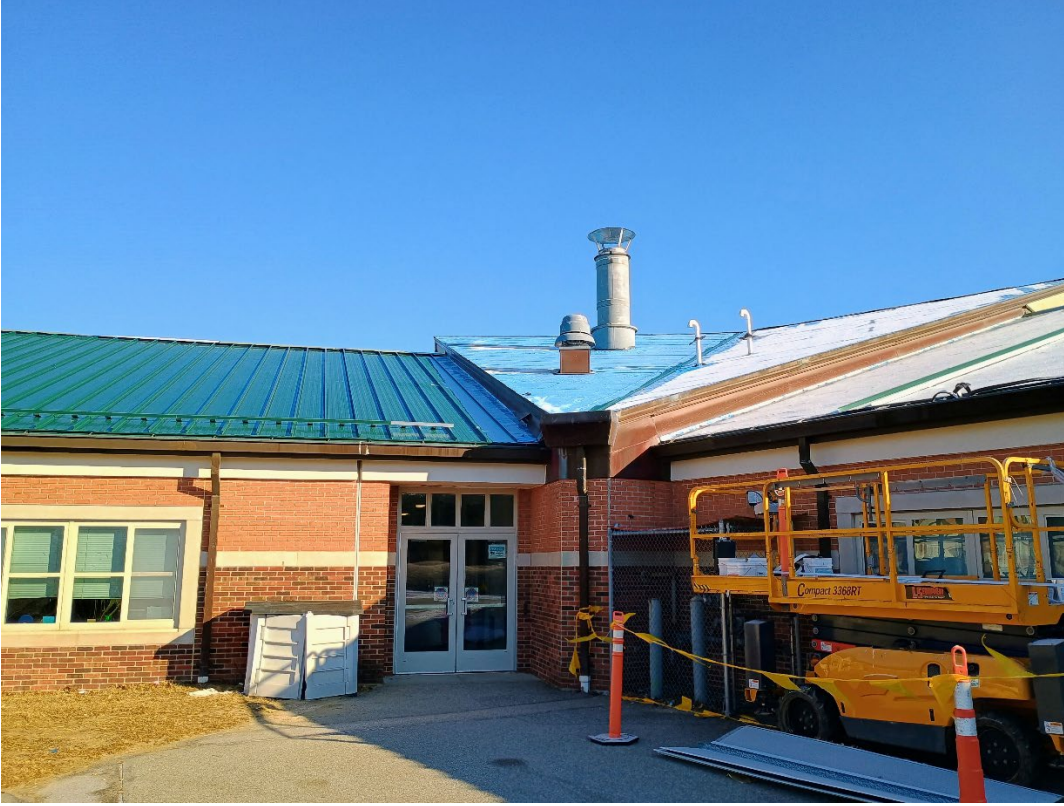
Roof E – Area of where new peel & stick membrane has been applied over the new existing peel & stick
