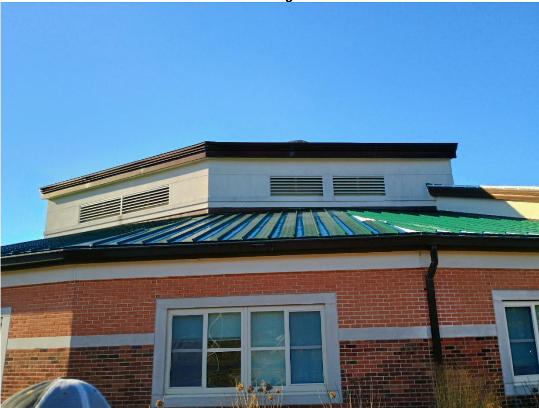
Roof E – Panels that need to be removed and longer screws need to be installed
