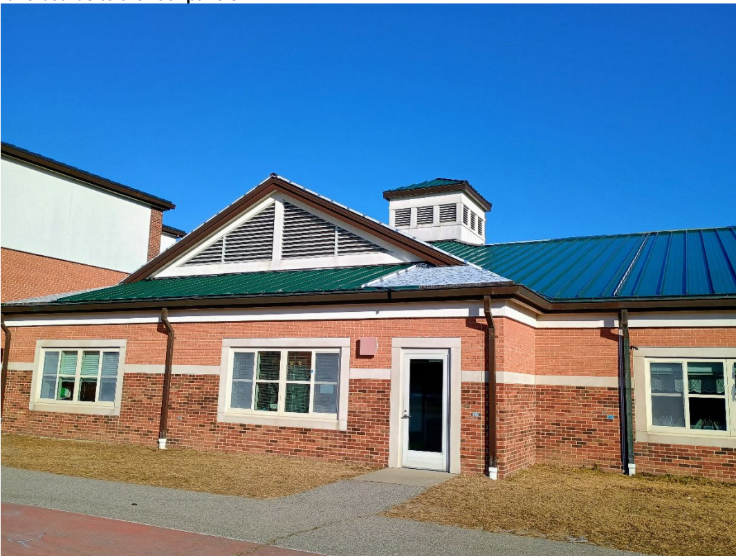
Roof A - One of the areas where Garland needs to produce a solution for the meeting of the rake boards to the roof panels
