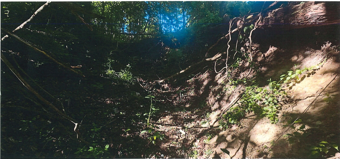
View Looking up Ditch from Adjacent to House
