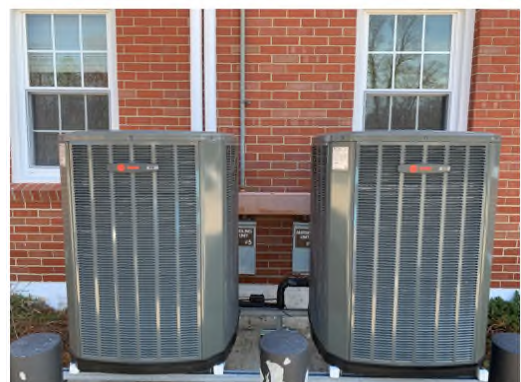
Town Hall HV/AC System Replacement
