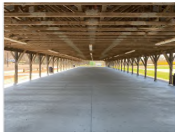
Concrete Floor Pole Barn Lower Town Green
