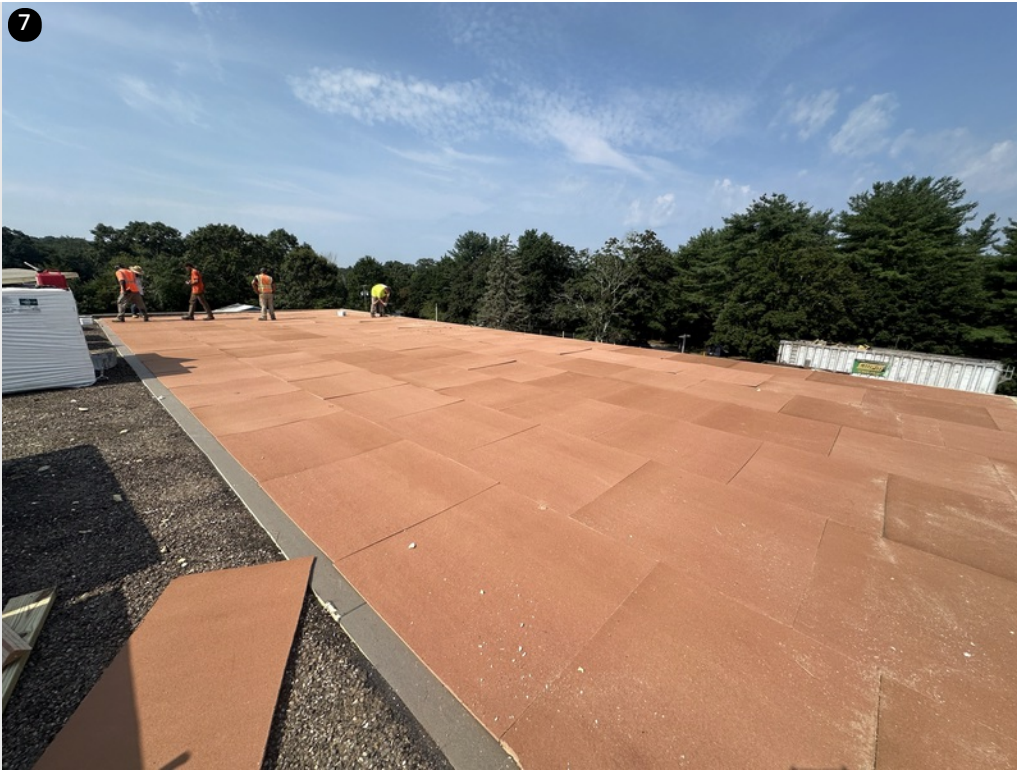
Upper roof section ripped to deck- 5" of insulation and coverboards being installed
