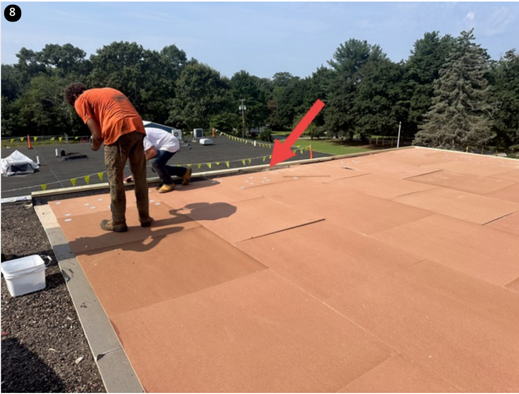
Overview of slope on upper roof section
