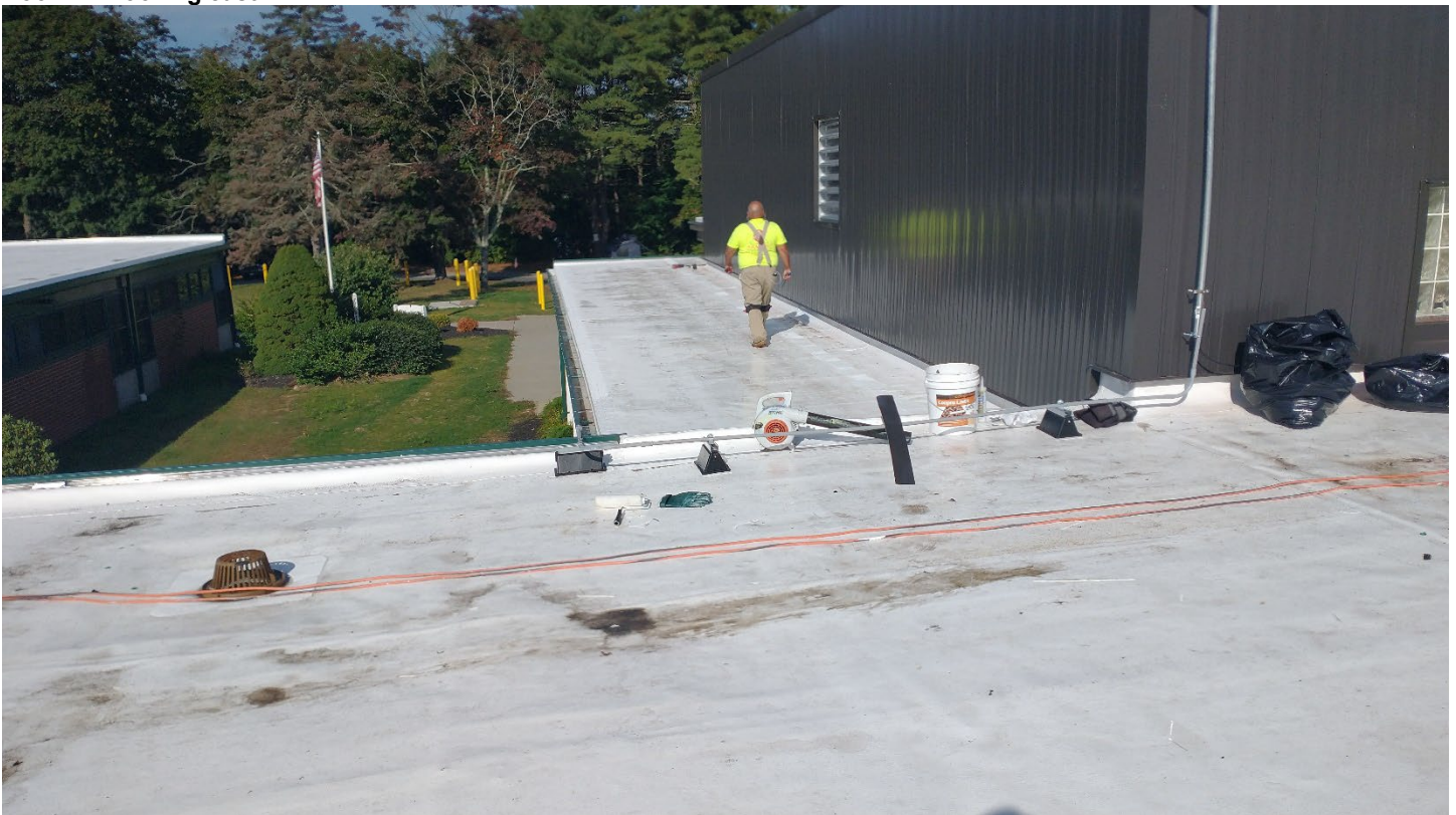
Roof D – Looking east
