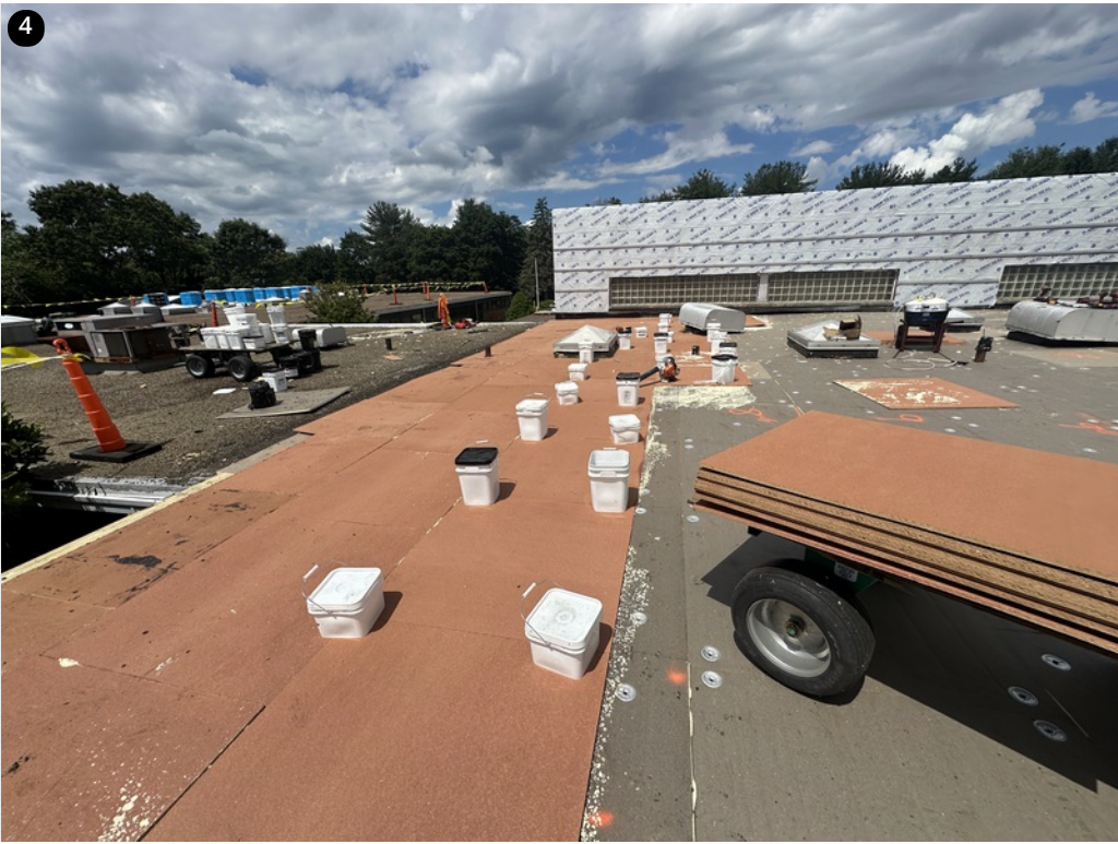
Crew using buckets of fasteners to weigh down adhered cover board
