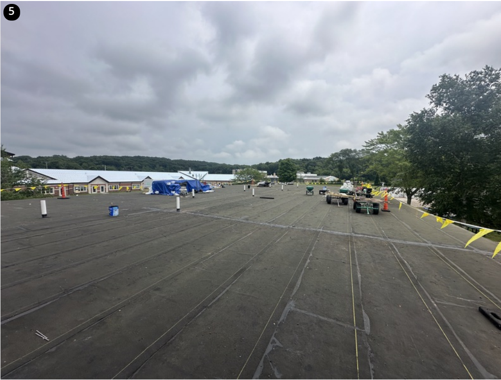
Overview- Completed base sheets on playground side
