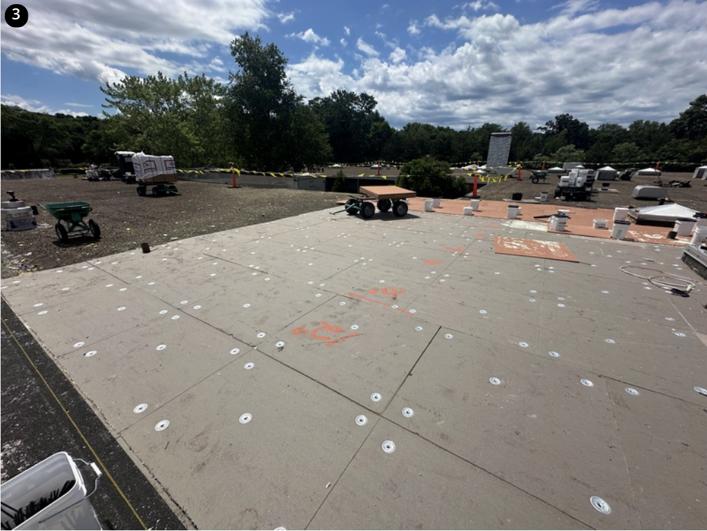
Overview- Fastening pattern on insulation boards
