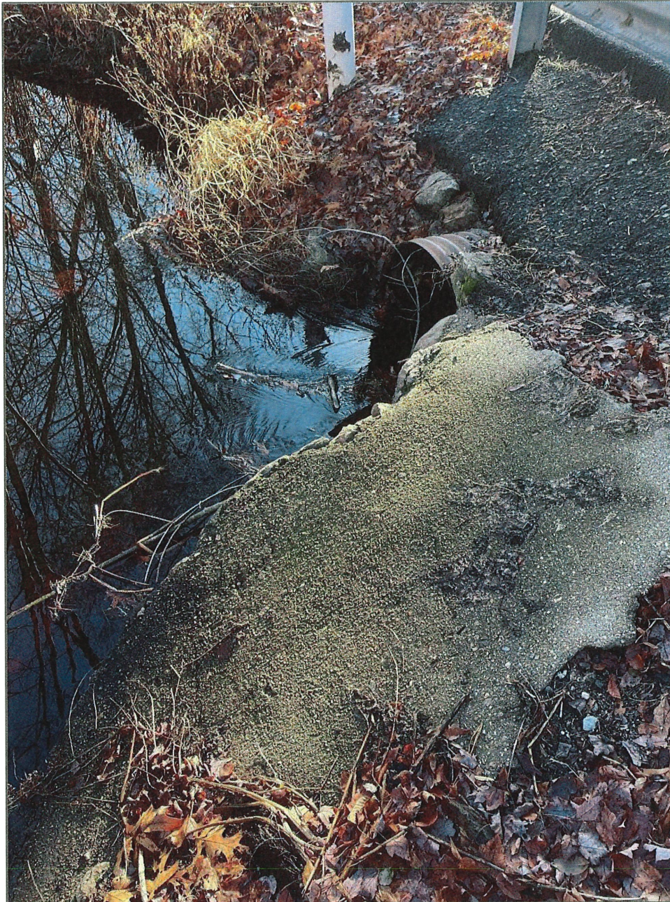
Photo 8: Auxiliary spillway inlet
