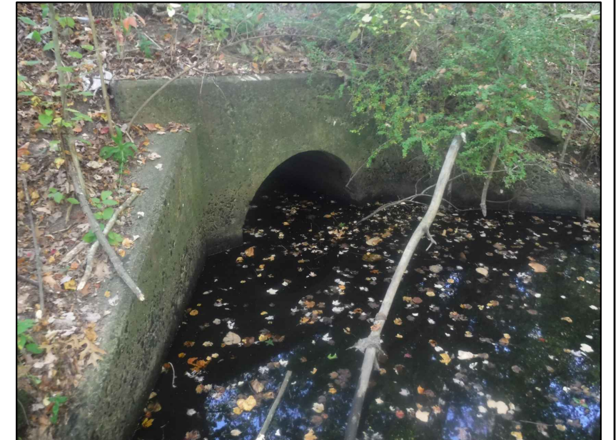
UPSTREAM (48" RCP SQUARE EDGE WITH HEADWALL)
