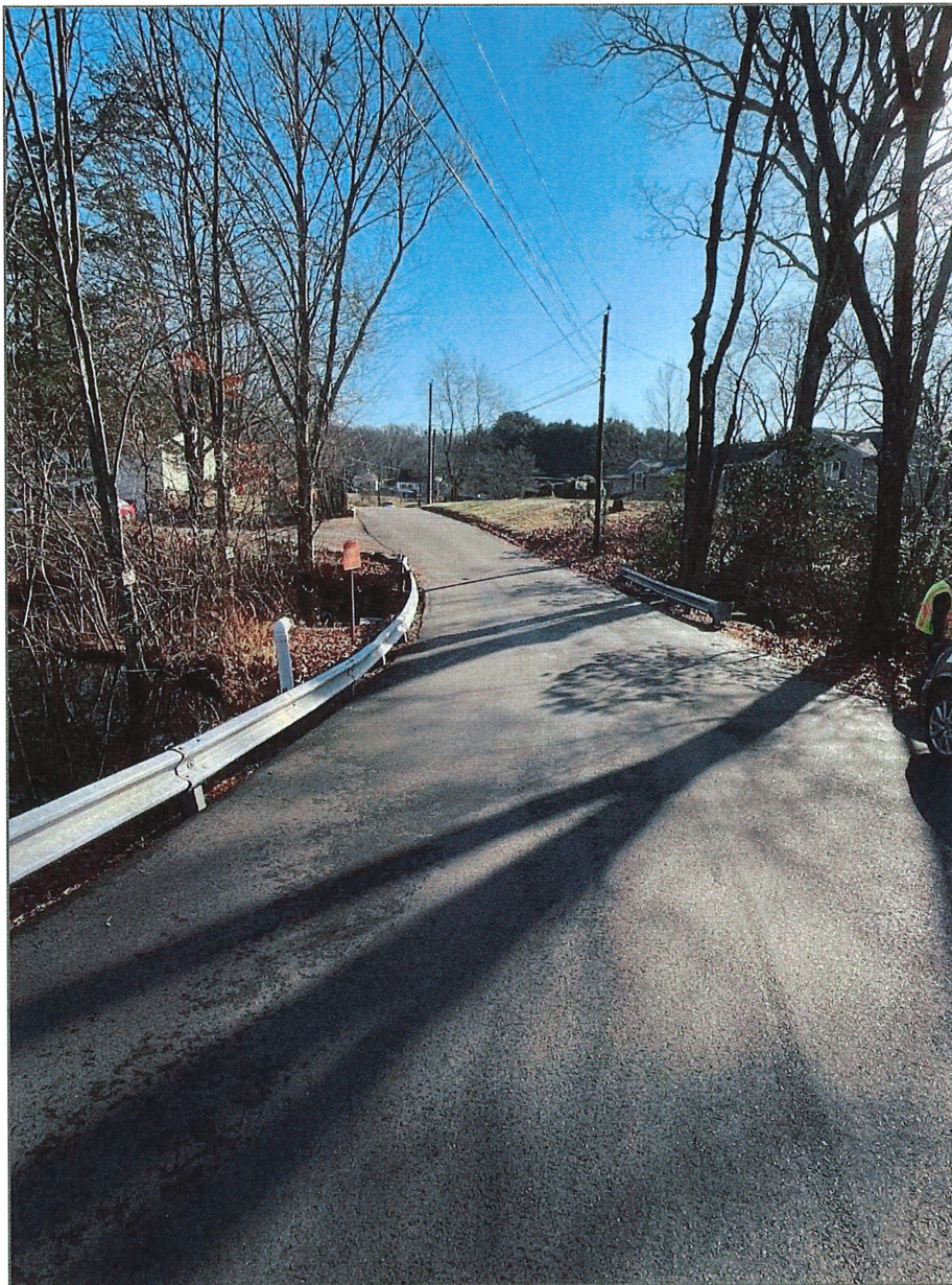
Photo 4: Roadway across dam embankment and beyond left abutment
