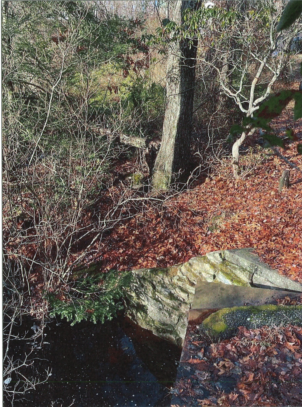
Photo 2: Downstream face of embankment
