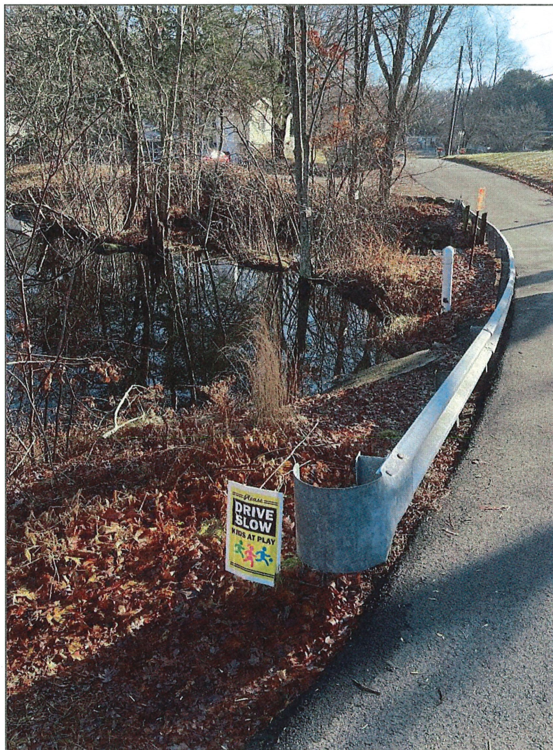
Photo 1: Upstream face of embankment
