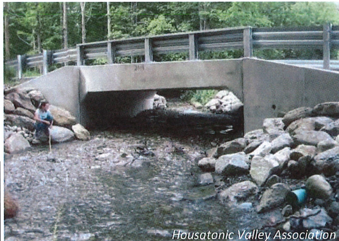
Success! A culvert replaced with a bridge on Churchill Brook in Pittsfield, MA allows wildlife to migrate and storm flows to pass through safely.
