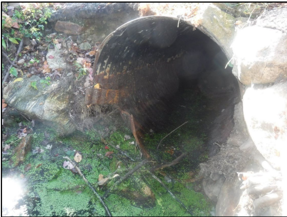
36" Corrugated Metal Pipe Inlet (Upstream)
