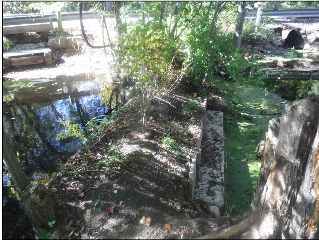
VIEW LOOKING SOUTHWEST FROM BERM TOWARDS DAM AND OUTLETS
