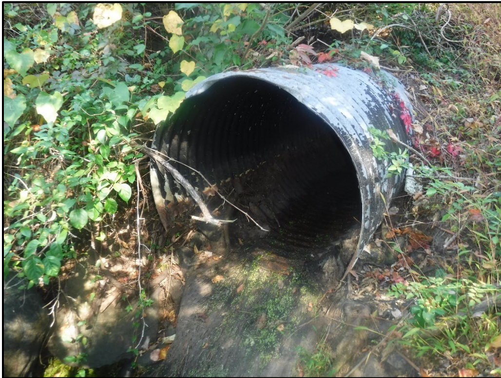
36" Corrugated Metal Pipe Outlet (Downstream)
