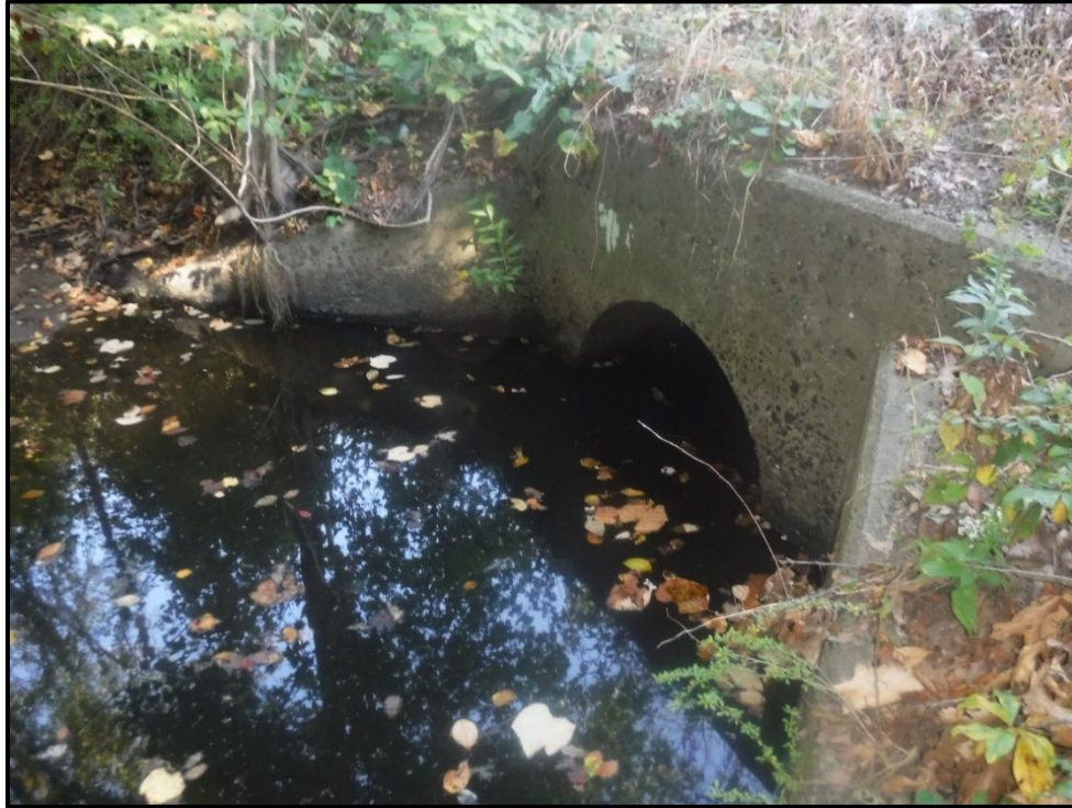
Route 12 Crossing Outlet
