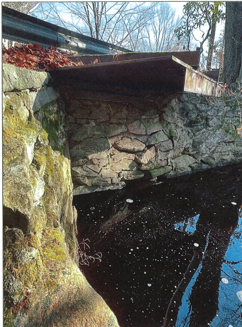
Photo 7: Principal spillway outlet
