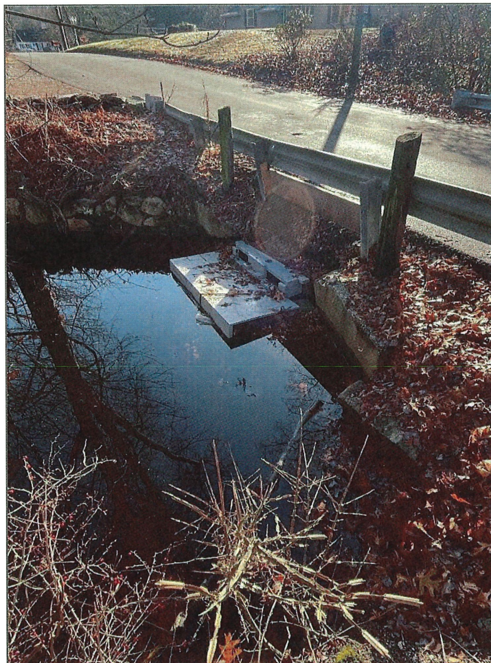
Photo 6: Principal spillway inlet with cover
