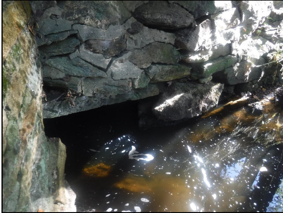
Multi-Stage Structure Outlet (Downstream)
