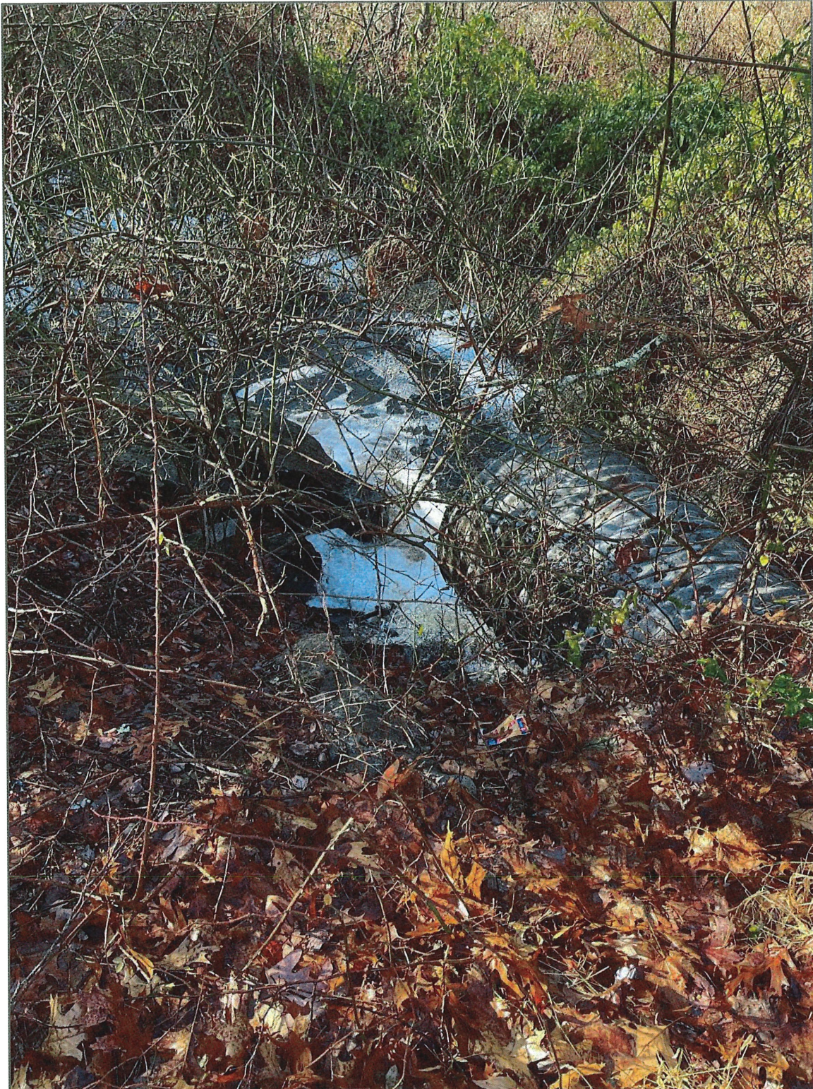
Photo 9: Auxiliary spillway outlet
