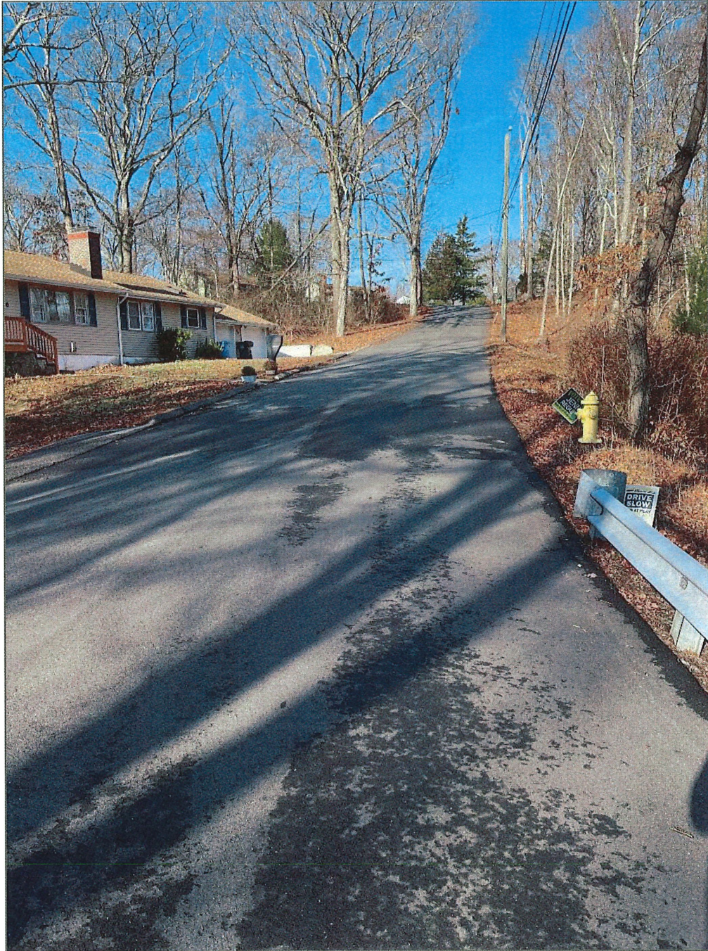
Photo 3: Roadway approach to right abutment and hydrant position
