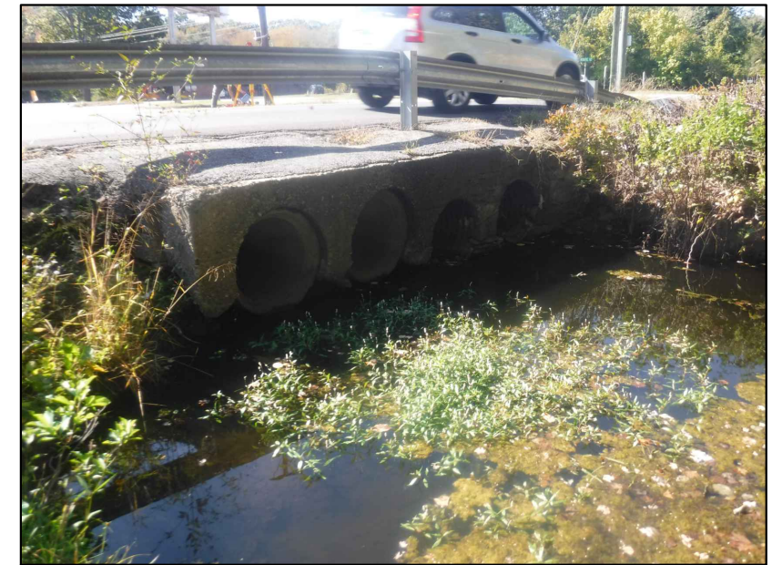
UPSTREAM (4 x 24" RCP SQUARE EDGE WITH HEADWALL)
