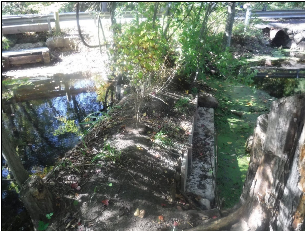
Earthen and Concrete Berm Separating the two Outfalls
