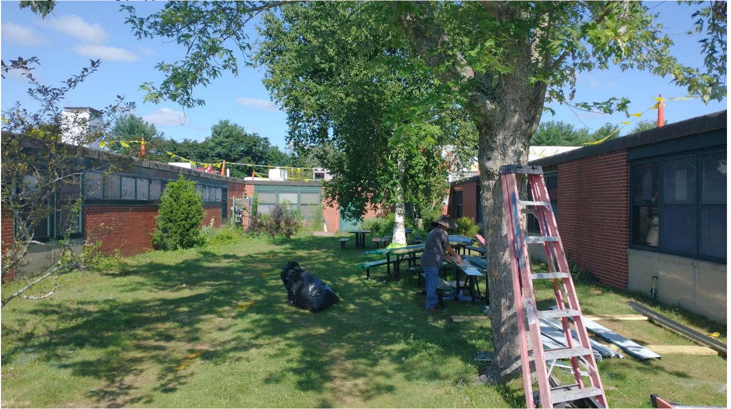
Roof edge trim being prepped for installation
