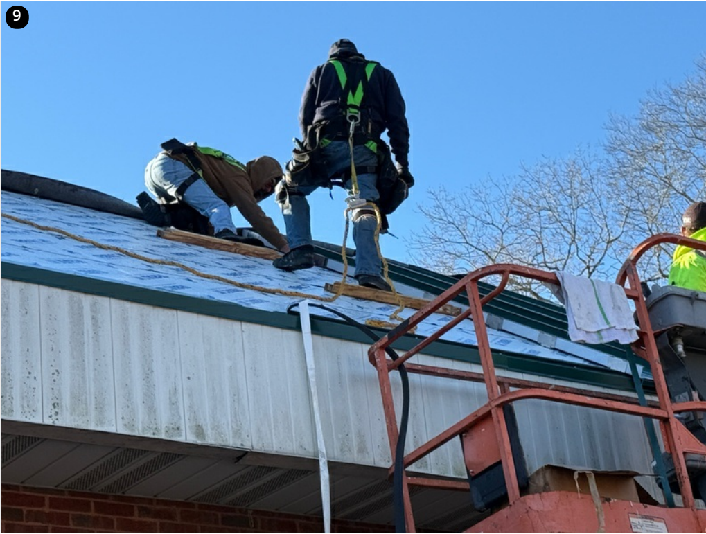
Crew fastening clips on North side 11/27/24
