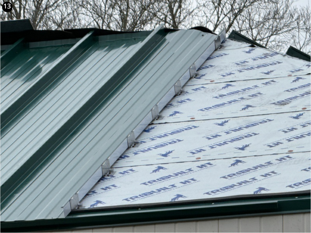
Clips installed 11/29/24
