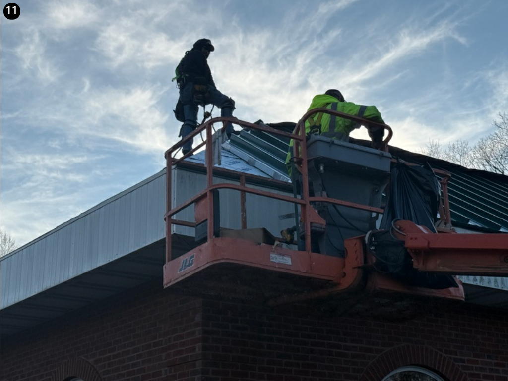
Crew installing panels on North East corner- 11/27/24
