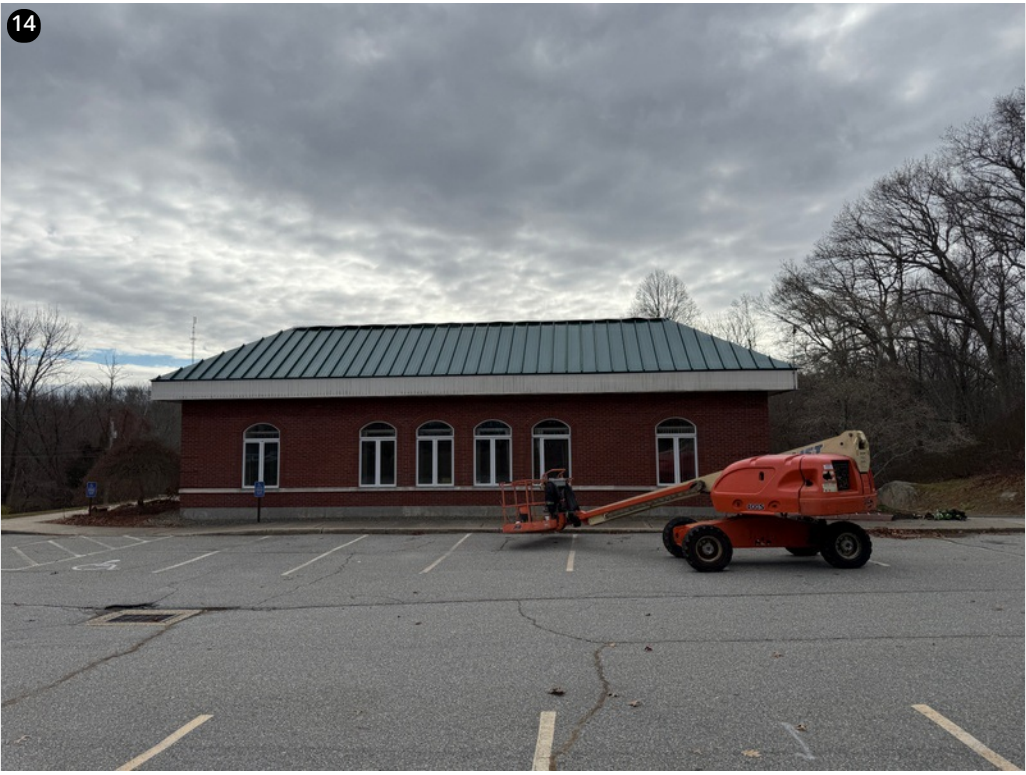
Overview- North side completed
