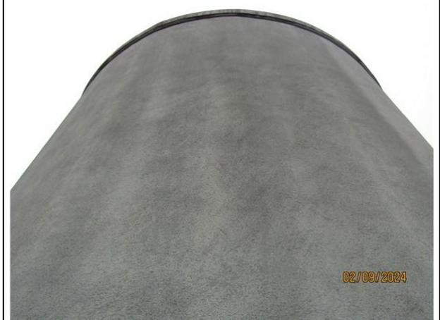
6) Typical condition of the exterior tank shell free of cracking and spalling
