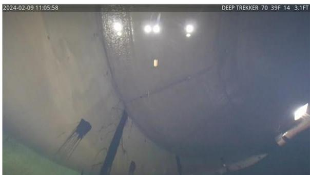
33) 1:54 - Interior roof free from cracking and spalling
