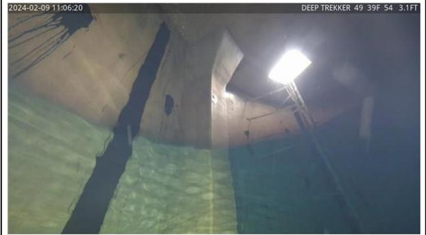
34) 2:16 - Interior overflow pipe encased in concrete
