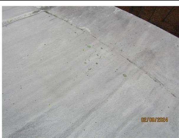
19) Exterior roof free of cracking and spalling
