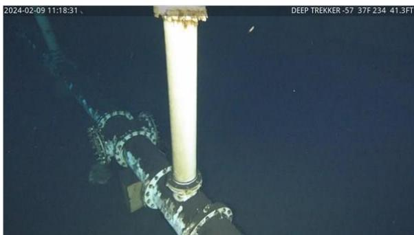
45) 14:27 - Combination inlet and outlet tree running horizontally across the tank floor
