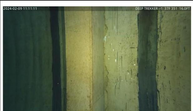
40) 7:08 - Concrete casing around interior overflow pipe
