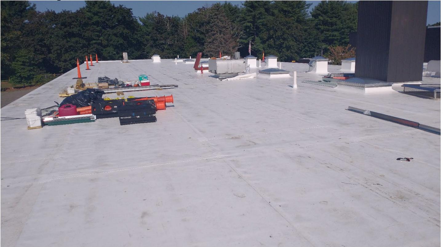
**Roof D – Rubber membrane seams need to be secured below metal siding**
