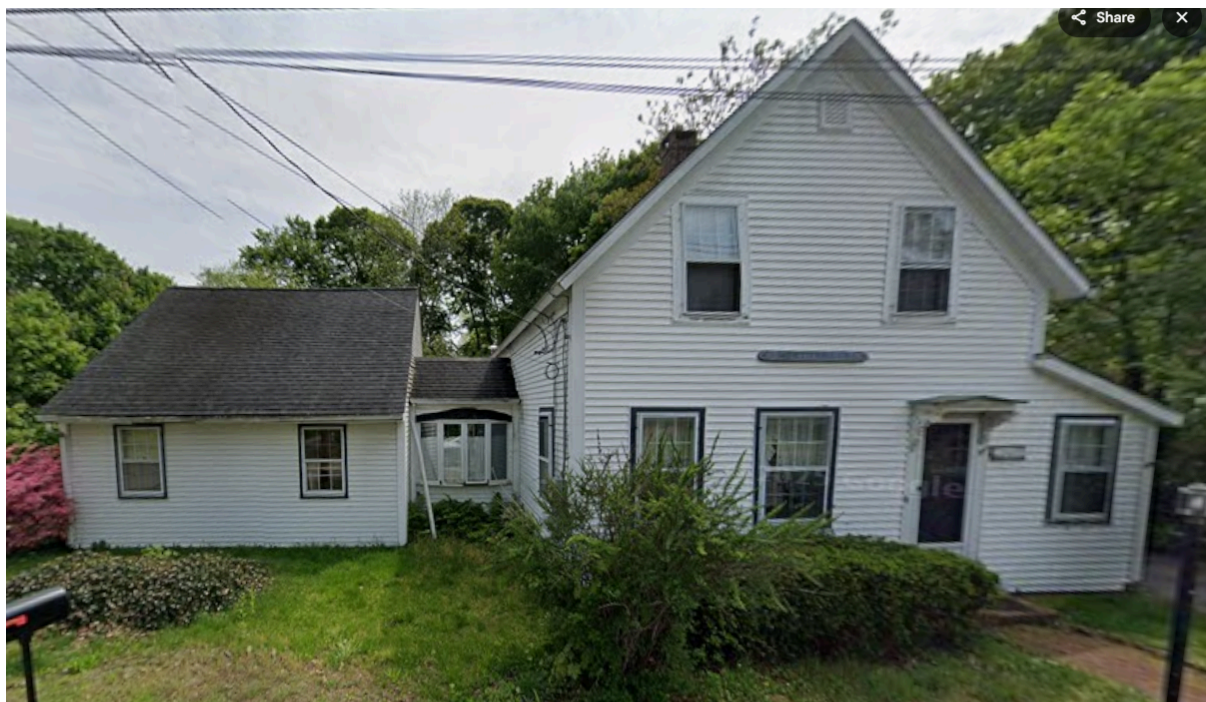
19th-century vernacular - John Bradford House, c. 1850
