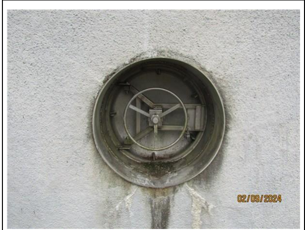
4) 1 of 2 lower shell manholes
