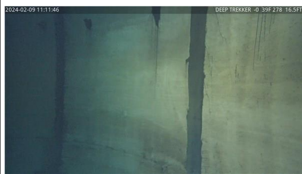
41) 7:42 - Intact shell substrate free of cracking and spalling
