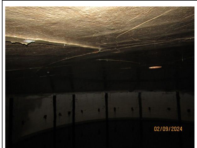
28) Typical condition of the interior roof
