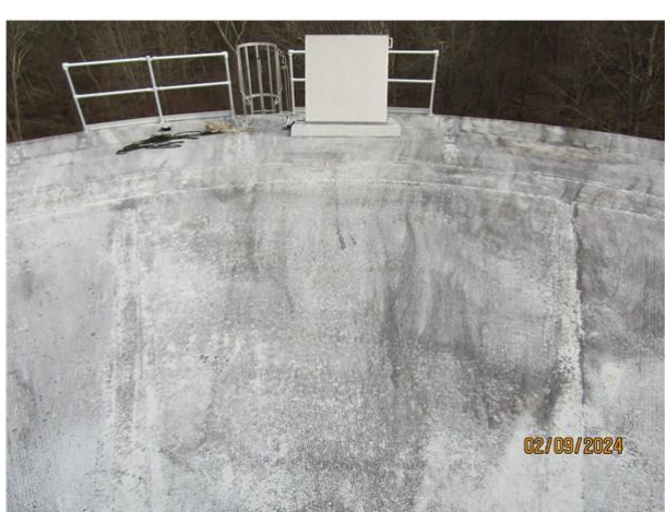
13) Roof railings and hatch
