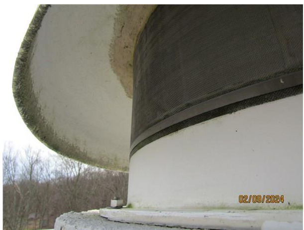
15) Intact fine mesh screening
