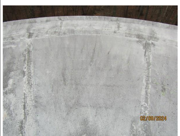
16) Typical condition of the exterior roof
