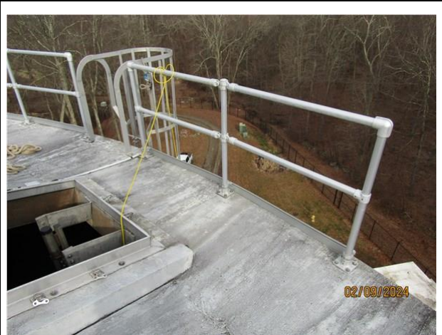
22) Perimeter roof railings flanking the shell ladder
