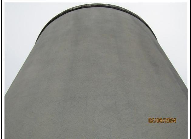
11) Tank shell free from visible cracking and spalling
