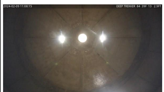
36) 4:11 - Typical condition of the interior roof free of spalling and cracking
