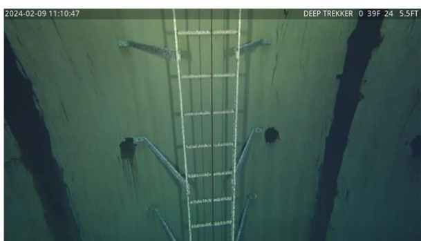
39) 6:44 - Typical condition of the interior ladder
