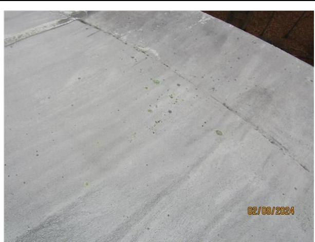
19) Exterior roof free of cracking and spalling
