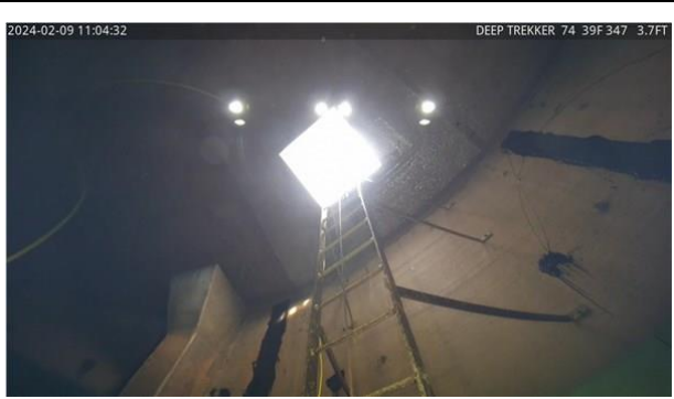
31) 00:29 - Perimeter roof hatch with ladder underneath
