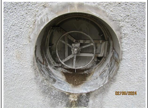
5) 2 of 2 lower shell manholes
