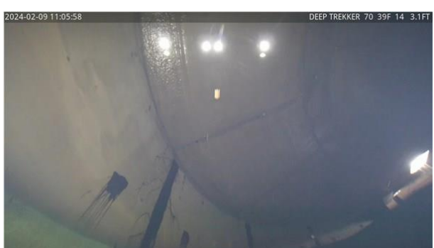
33) 1:54 - Interior roof free from cracking and spalling
