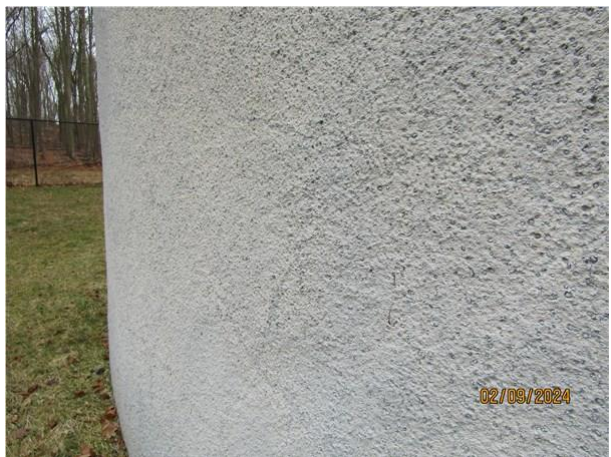
8) Intact shell surfacing material free of adhesion loss
