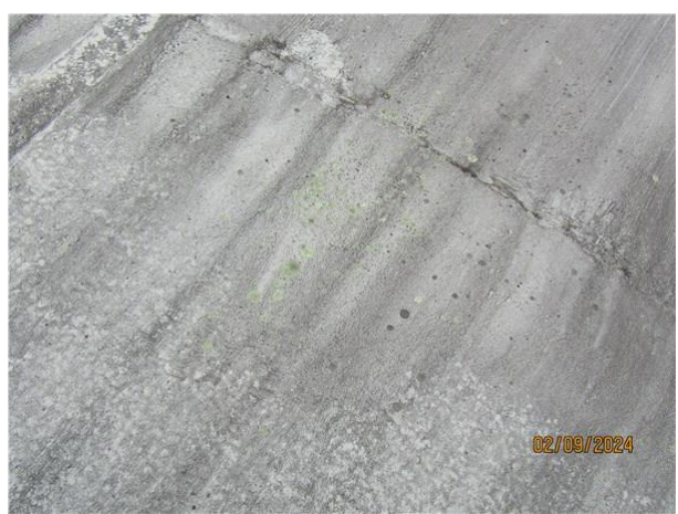
20) Typical roof seam
