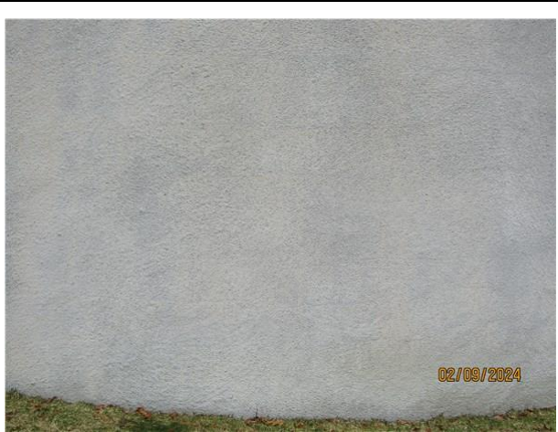
7) Typical condition of the exterior tank shell
