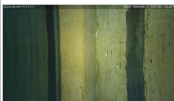
40) 7:08 - Concrete casing around interior overflow pipe
