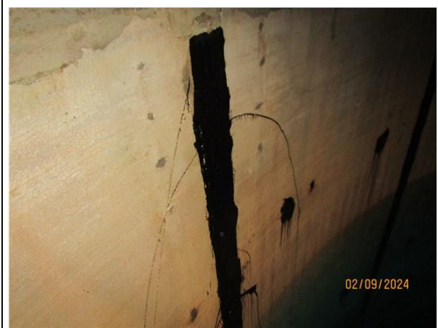
27) Typical condition of the interior above water shell
