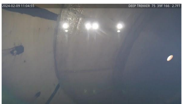
32) 00:51 - Typical condition of the above water shell and roof
