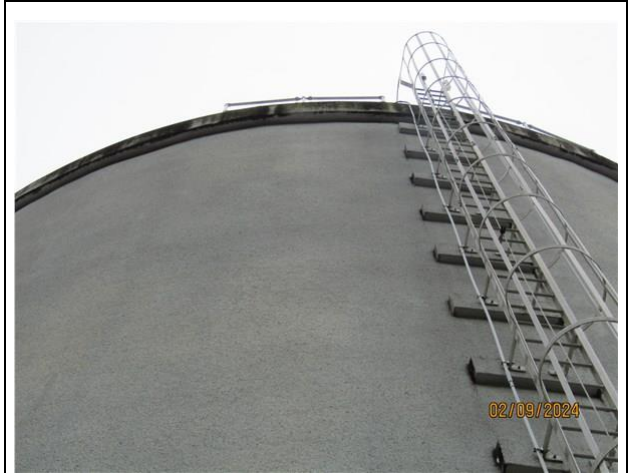
10) Typical condition of the upper shell
