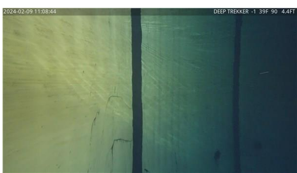
37) 4:40 - Typical condition of the submerged interior shell
