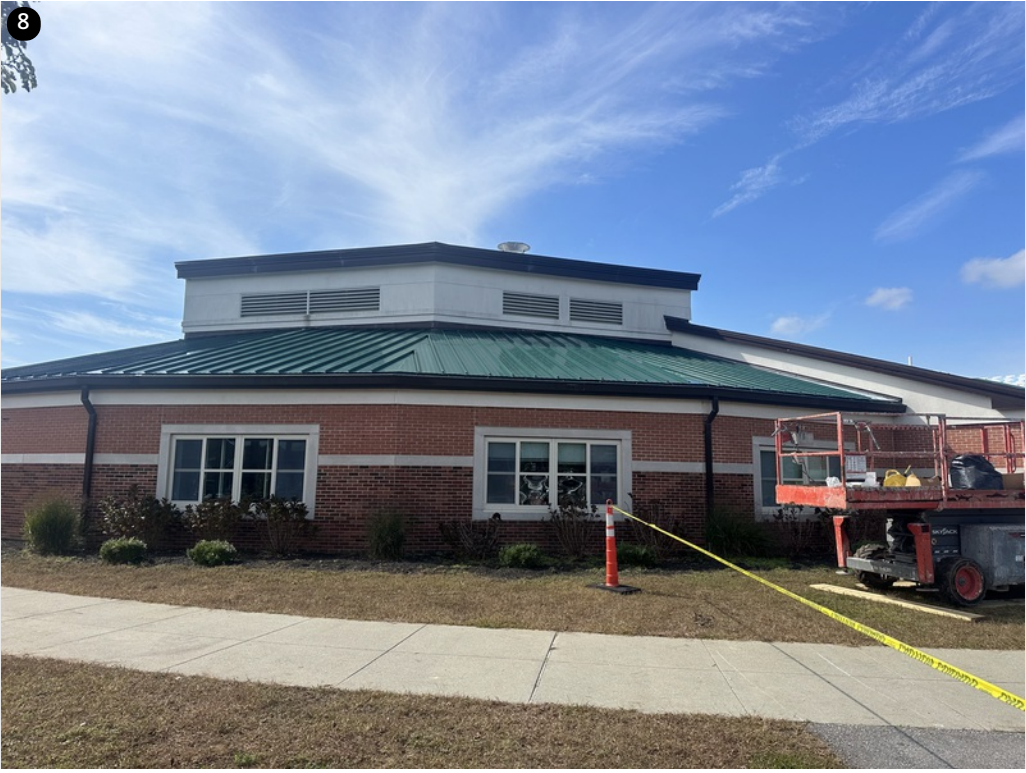
Ground level overview
