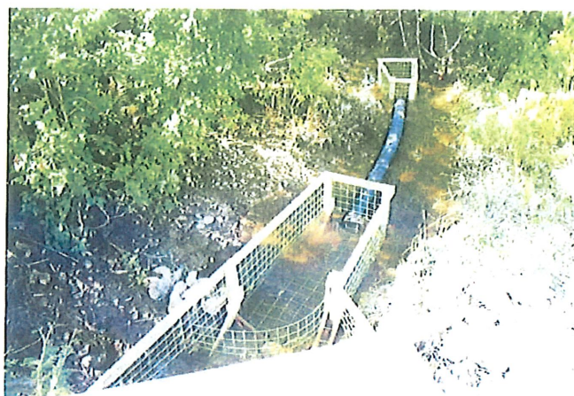
A Double Filter System™ composed of two Beaver Deceivers™. The initial fence has a Turtle Door™ (also used by other animals) on the left side (see photo below). The low, arched fence in the middle guides animals to the hole. The stones at the top prevent beavers from floating debris through the hole and into the culvert.
