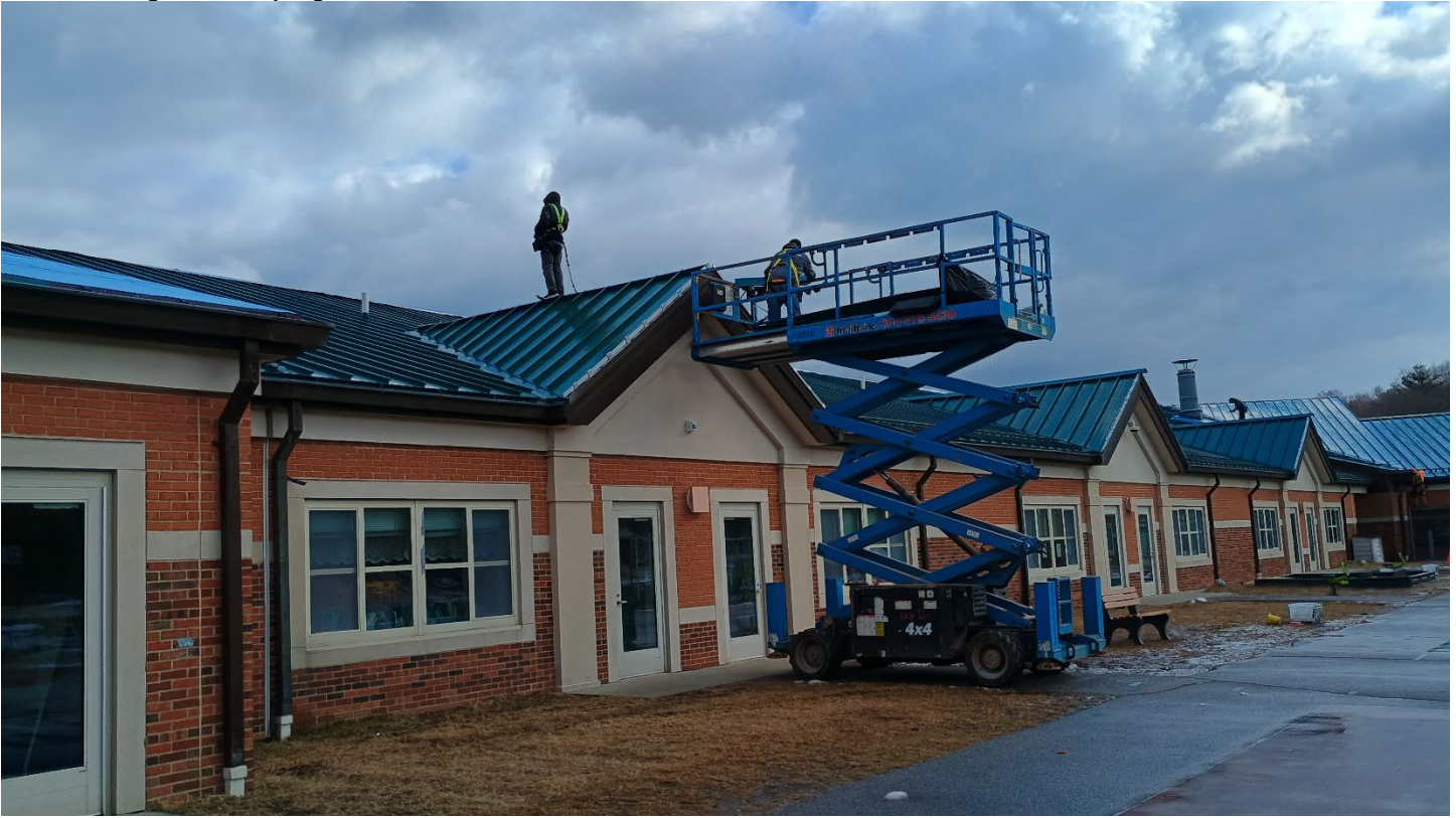
Roof D – Ridge work in progress
