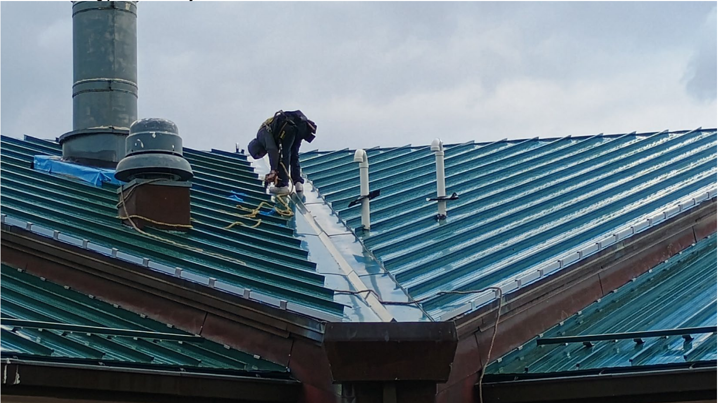
Roof E – Securing panels to valley
