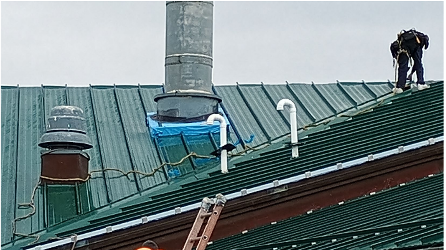
Roof E – Box out of roof exhaust
