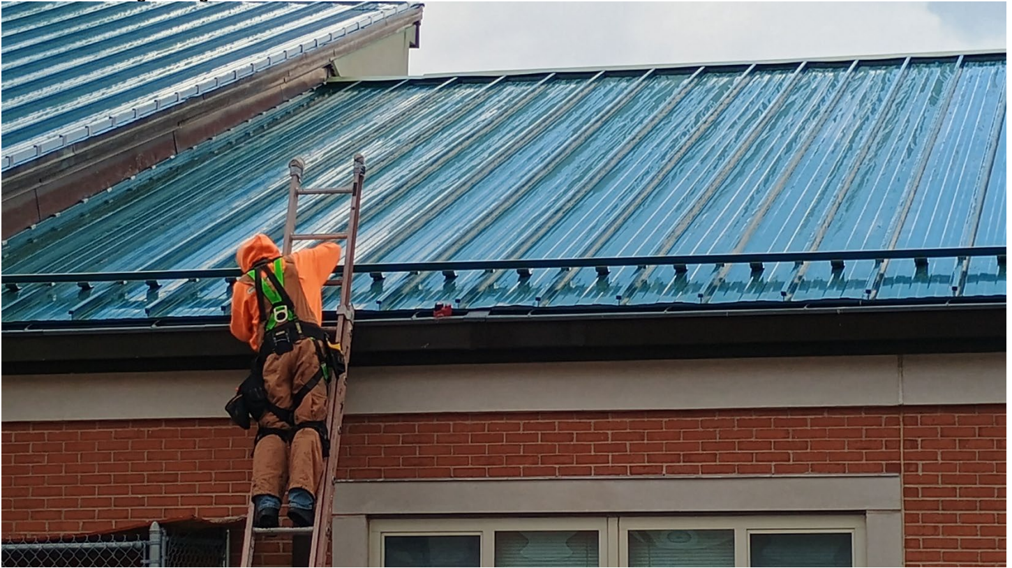
Roof F – Installing snow guards
