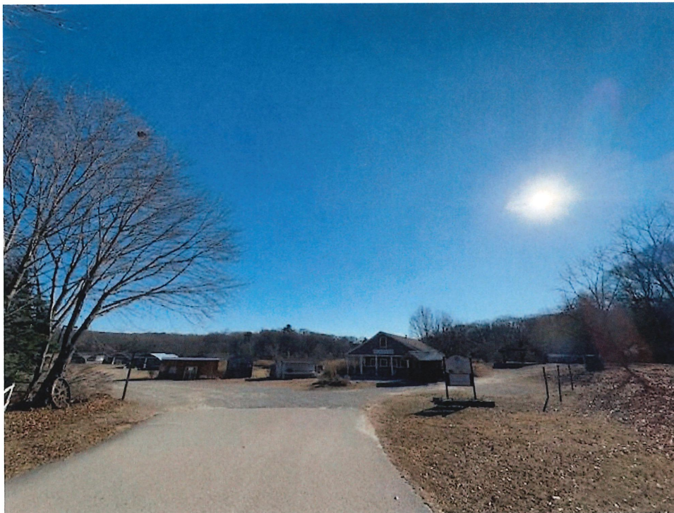
Photo 4: Site entrance and Sweet Hill Farms structures slated to be removed.
