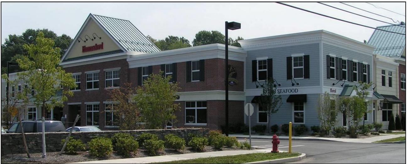
Big box developments should replicate historical Village character by creating individual storefronts. (Photo Credit: Laberge Group.)
