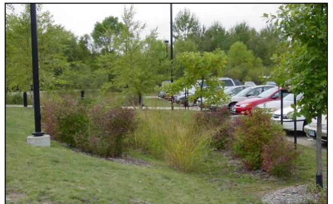
Rain gardens are bio-retention areas designed to absorb stormwater runoff. (Picture Credit: www.urbanwaterquality.org , 2009.)
