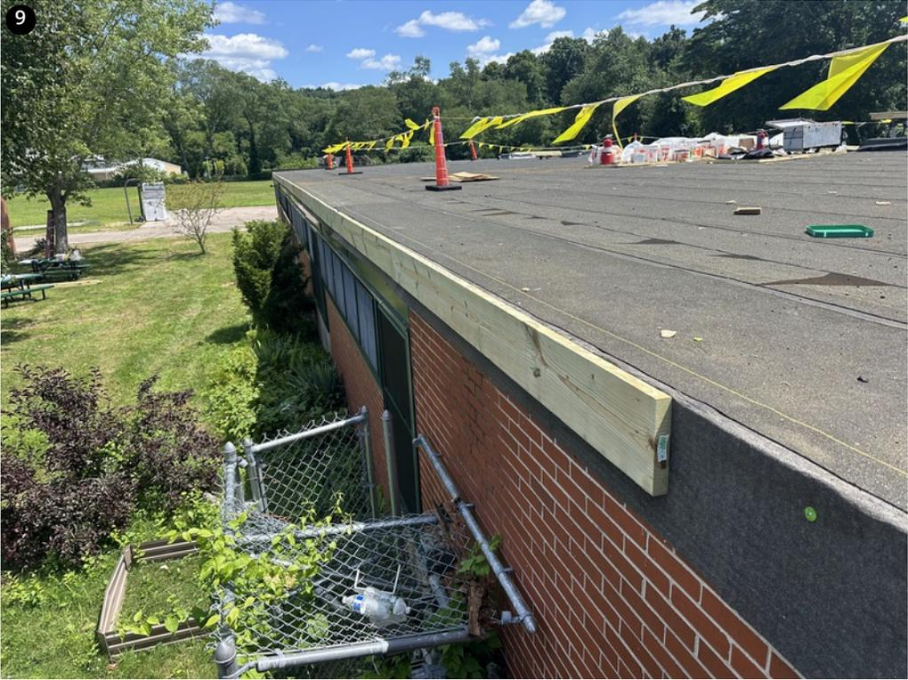
9 Fascia blocking has been installed around the perimeter-Will be covered with ice and water
