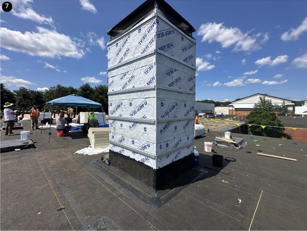
7 Chimney with completed ice and water application- Hat channels are secured- Base flashings completed with cant strips in place
