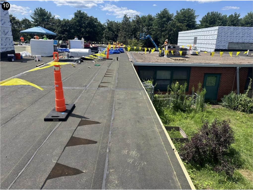
10 Field- Good bleed out at lap seams- Sheets lapped correctly for slope- Fascia blocking installed
