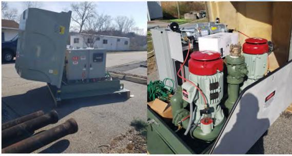
New Skid Mounted Sewer Pumps
