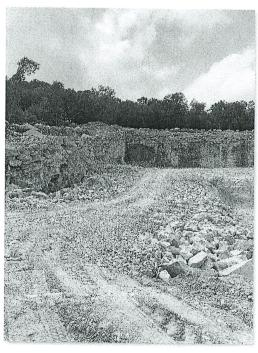
Topography on the site ranges from an elevation of approximately El 82 at the floor of the existing exaction to El 220 in the southwestern corner of the property. The proposed work consists of extending the excavation operations to the south of the current operation. The largest proposed cut is approximately 160 feet northeast of the southwest corner with a depth of cut of approximately 80 feet, with the base at El 110.
