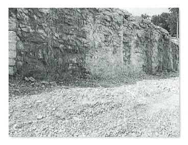
In the photograph to the left, showing a portion of the rock race, groundwater can be seen in some portions of the rock and other areas are dry. The amount of water fro these fissures flowing into the excavation are small and does not require pumping. At the time of the visit, there was no standing water on the floor of the excavation, indication that the cuts do not intersect a standing water table in the area and the only water is flowing in from the faults in the bedrock.
