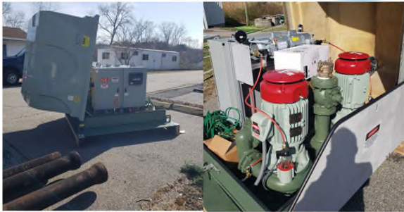
New Skid Mounted Sewer Pumps Wastewater Treatment Facility
