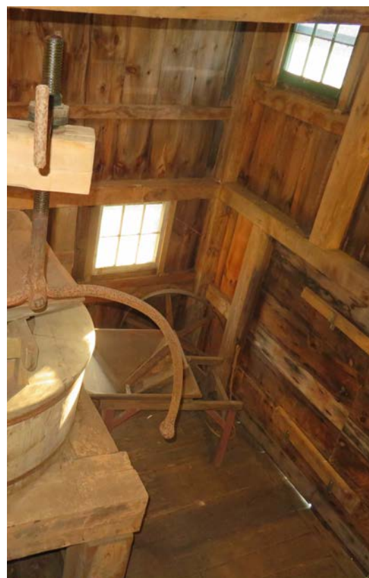
Left: Exterior of east elevation; Right: interior of south east corner showing horizontal girts and board supports.
