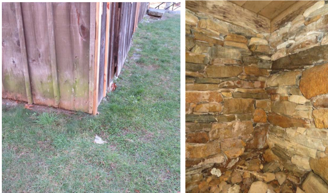
North gutter, west end; Left: grade where gutter is discharging; Right: inside face of foundation wall at northwest corner showing dampness and fungal growth on sill above.
