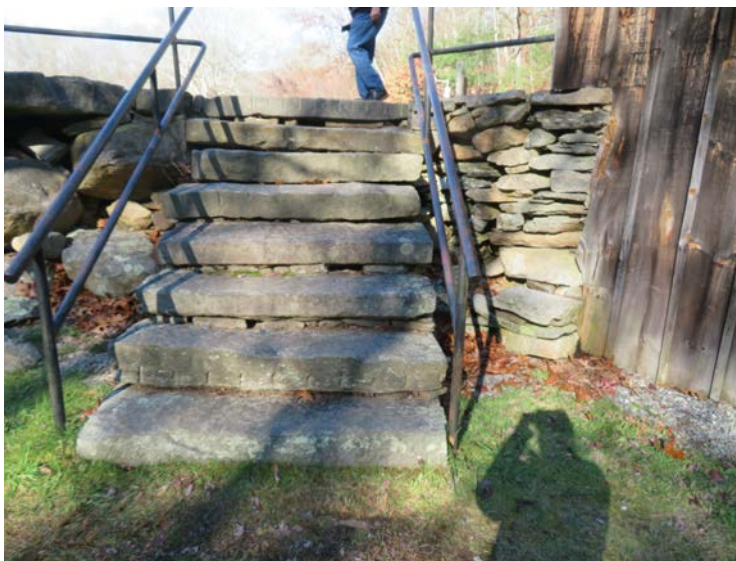
Displacement of steps and dry laid retaining wall at lower level below eroded areas above
