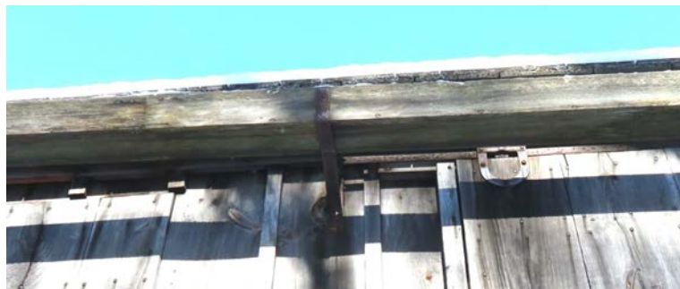
South gutter showing box gutter shape, weathering, biological growth and brackets.
