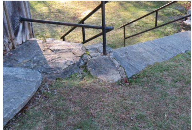
Erosion at west side of building, to north and south of door threshold
