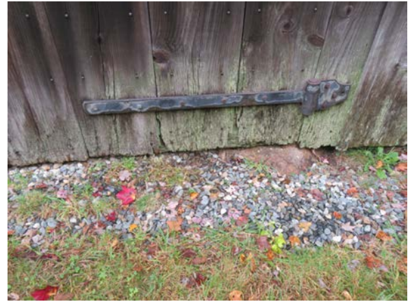
Central double doors at south elevation (lean-to) showing siding deterioration and sill / threshold deterioration behind.
