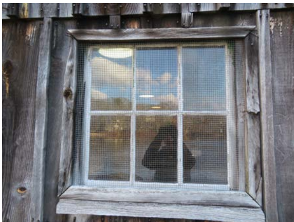
Exterior original mill window with wood mounted screen. Sill is weathered with dry end grain.
