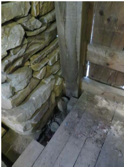
Left: Bottom of east wall post just above decking over raceway, post base is concealed below decking; Right: Deterioration of east end of decking sill over north wall of raceway looking east to gate to tail race, the post base is not apparent in this image but deterioration of deck sill is suggestive.
