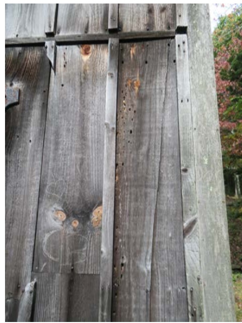
Left: Termite damage at the grist mill frame; Right: tell-tale termite trails / holes at siding at the east end of the south elevation.
