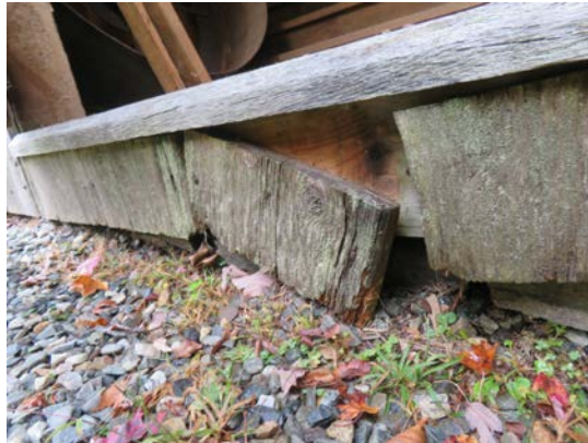
Siding and foundation below grist mill exterior doors. Siding nails have failed, but sill behind appears to be in good condition.
