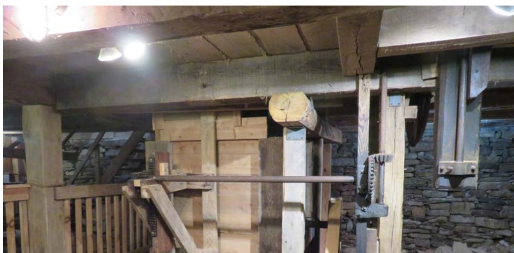
Top: overall view of fender beam from the east showing two saw guides extending below; Middle: north end of fender beam; Bottom: south end of fender beam including newer intermediate post supported on north raceway wall below.
