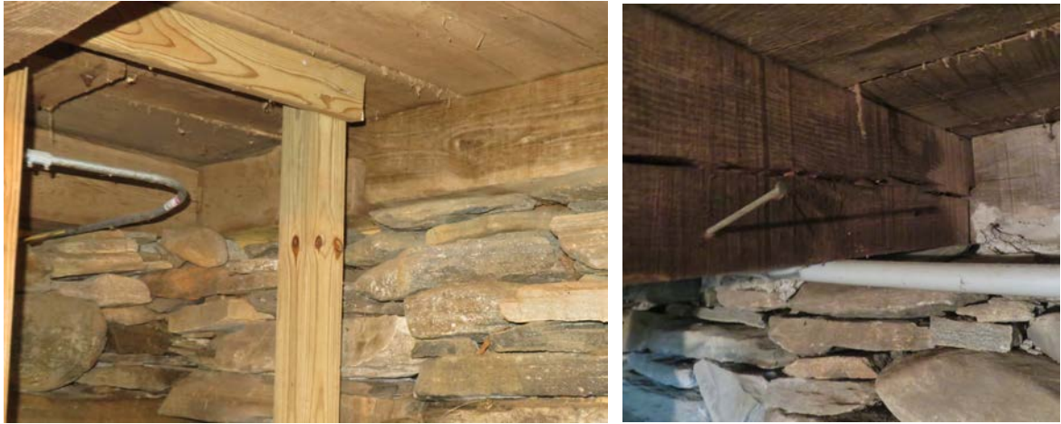
Left: Northeast corner from basement showing sill corner tenon (possibly bent); Right: East end of north beam show shear crack parallel with tenon (stress concentration).
