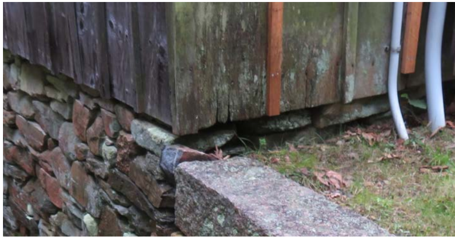
North gutter, east end, showing deteriorated board siding and erosion in masonry.
