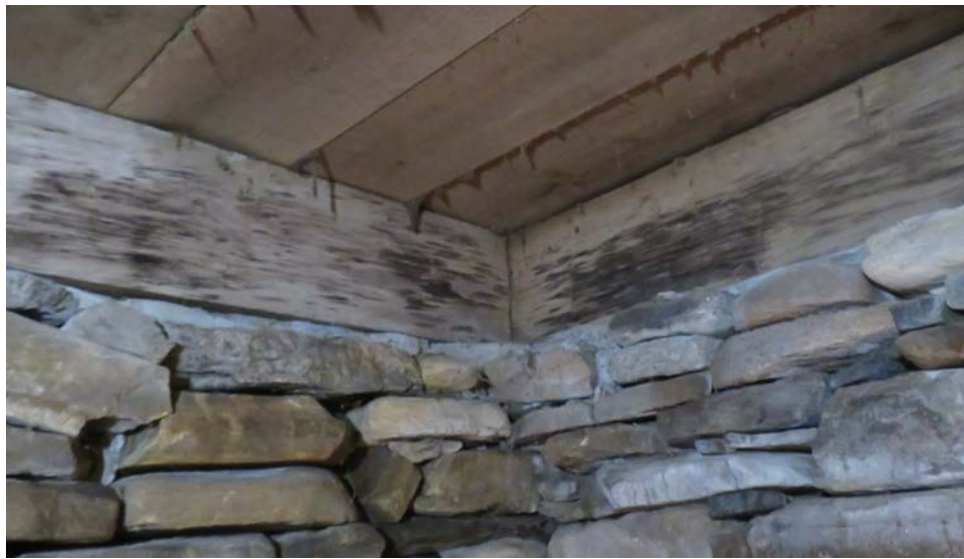
Northwest corner of sills from the basement showing black staining presumed to be fungal growth.
