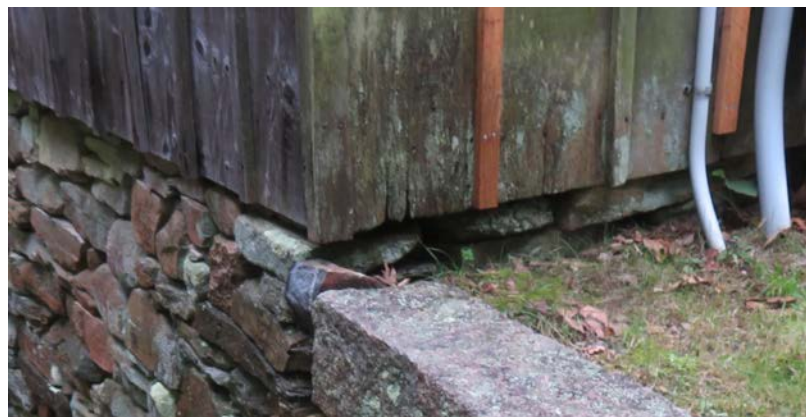
Exterior of northeast corner showing siding deterioration.
