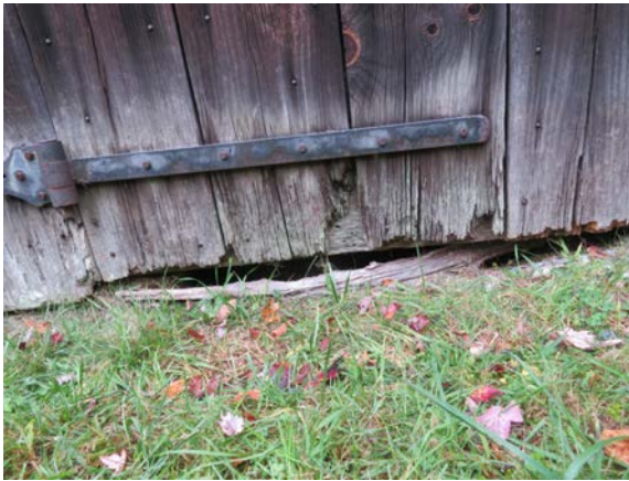
Central double doors at south elevation (lean-to) showing siding deterioration and sill / threshold deterioration behind.
