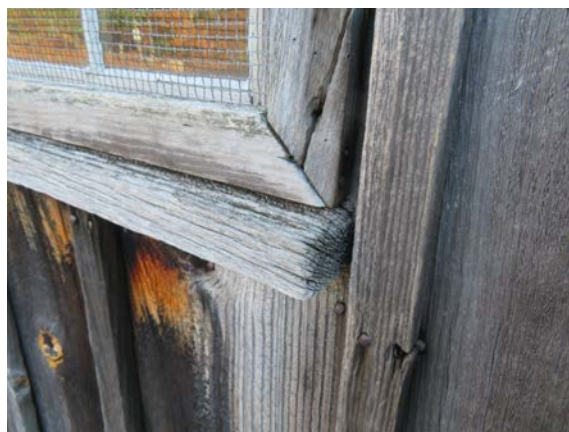
Exterior original mill window with wood mounted screen. Sill is weathered with dry end grain.
