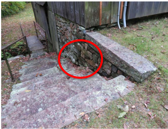
Top: Overall view of damage; Bottom Left: Bulge in foundation wall; Bottom Right: Shifting and movement of bottom 3 steps due to erosion of soil below.
