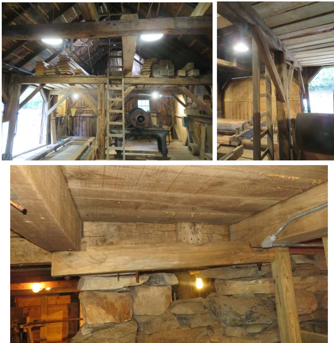
Overall Loft and Loft-West support line. Left: Loft-West north bay showing replacement post; Right: Loft-West middle post with hung beam support below.
