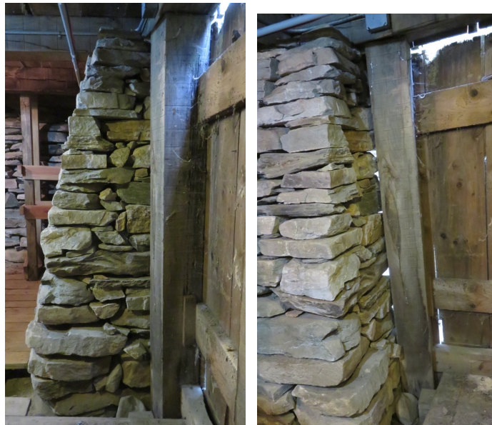
Left: Northeast corner from basement showing sill corner tenon (possibly bent); Right: East end of north beam show shear crack parallel with tenon (stress concentration).
