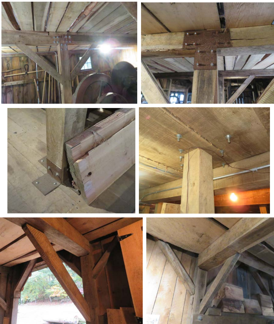
Loft-Central support line. Top: Middle post and beam connections at top; Middle: Middle post connection at bottom; Bottom: Beam connections into end post using historic joinery.
