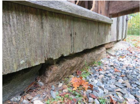
Siding and foundation below grist mill exterior doors. Siding nails have failed, but sill behind appears to be in good condition.
