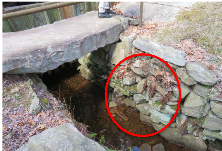
North tailrace wall showing bulge in dry laid masonry
