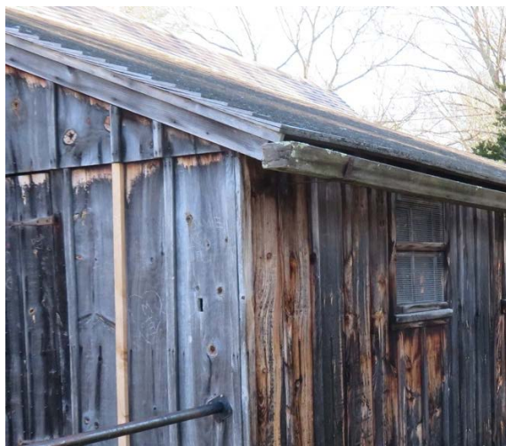
South gutter showing dip (likely missing bracket) toward east end.
