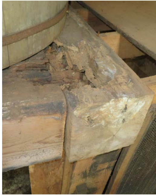
Left: Termite damage at the grist mill frame; Right: tell-tale termite trails / holes at siding at the east end of the south elevation.
