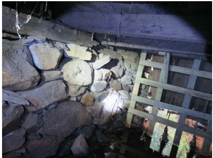
Left: Bottom of east wall post just above decking over raceway, post base is concealed below decking; Right: Deterioration of east end of decking sill over north wall of raceway looking east to gate to tail race, the post base is not apparent in this image but deterioration of deck sill is suggestive.
