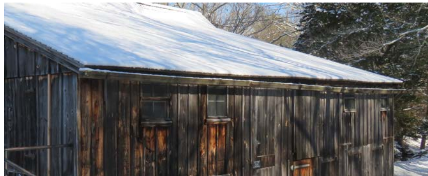
South gutter showing dip (likely missing bracket) toward east end.
