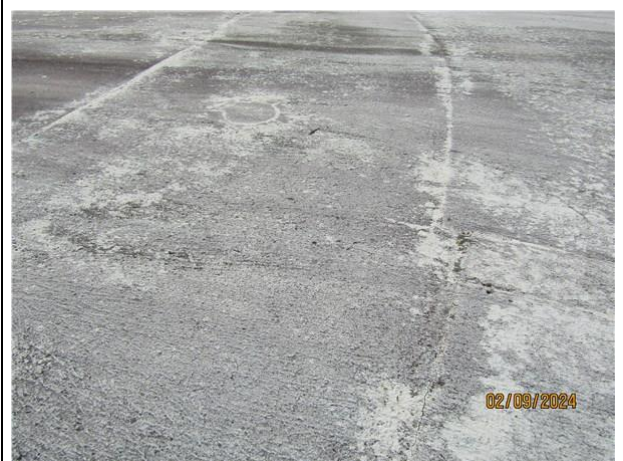
18) Weathering of exterior roof surfacing material
