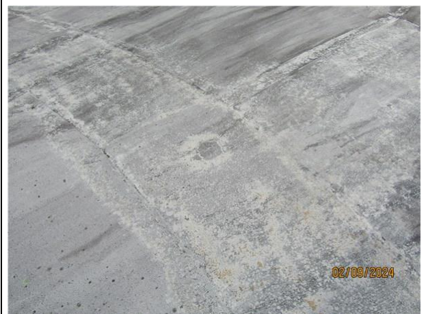
17) Biological staining of the exterior roof
