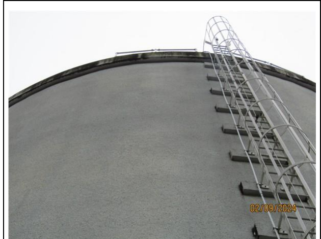
10) Typical condition of the upper shell
