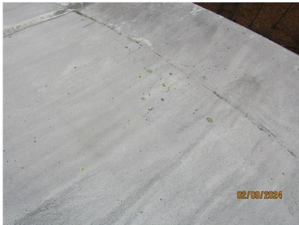
19) Exterior roof free of cracking and spalling
