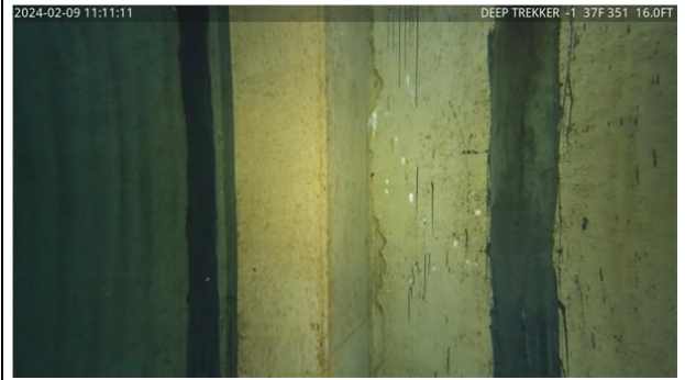
40) 7:08 - Concrete casing around interior overflow pipe
