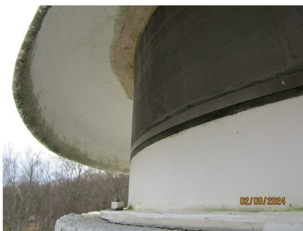
15) Intact fine mesh screening
