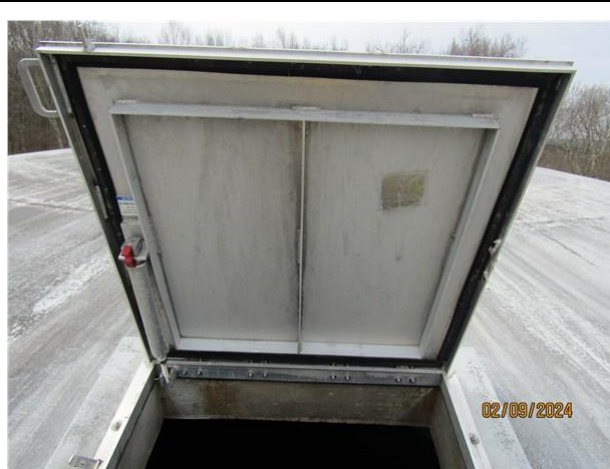
25) Intact hatch cover gasket
