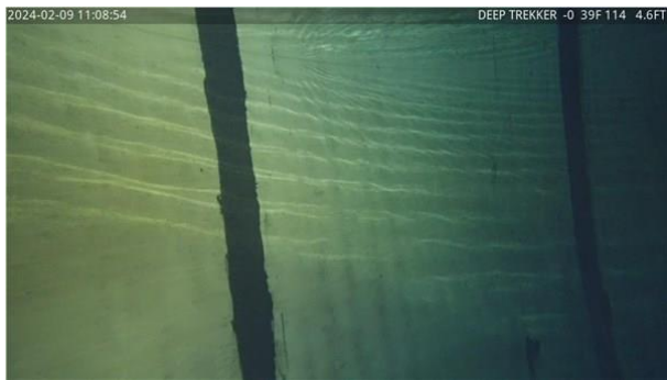
38) 4:51 - Intact seam seal material
