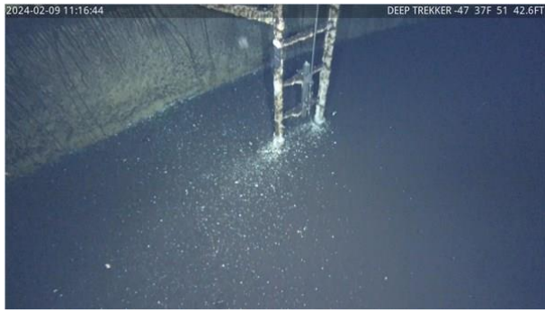
43) 12:40 - Oxidation of interior ladder due to dissimilar metals used on the safety climb
