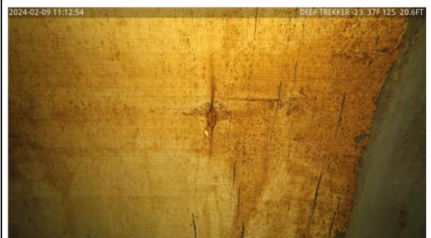
42) 8:50 - Corrosion cell from exposed rebar tie in
