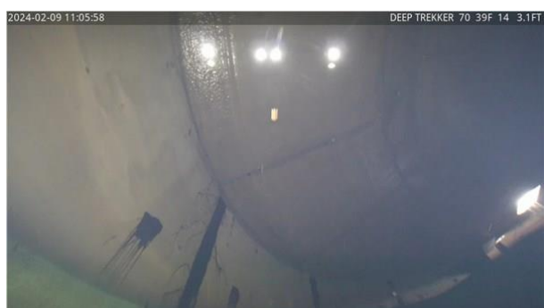
33) 1:54 - Interior roof free from cracking and spalling
