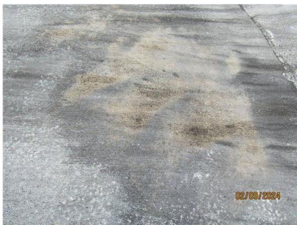
21) Area of discoloration on the exterior roof
