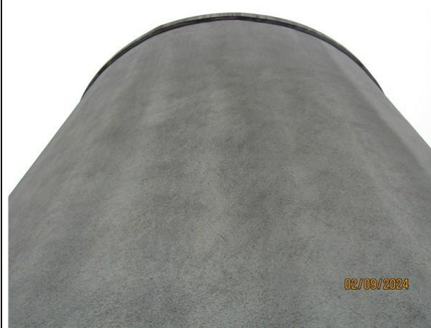
6) Typical condition of the exterior tank shell free of cracking and spalling
