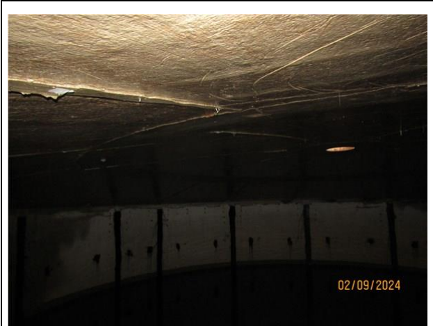
28) Typical condition of the interior roof
