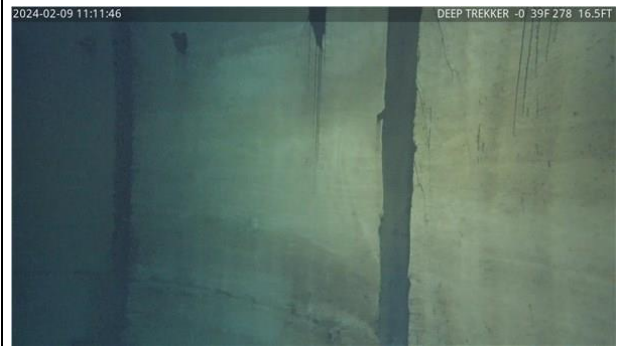
41) 7:42 - Intact shell substrate free of cracking and spalling
