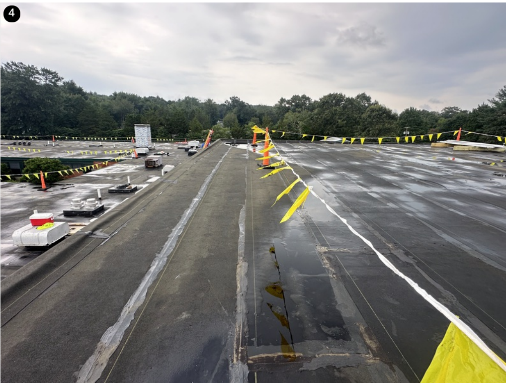
4 Water being displaced around cricket towards corner drains- Drains will be sumpt before cap sheet adhesion
