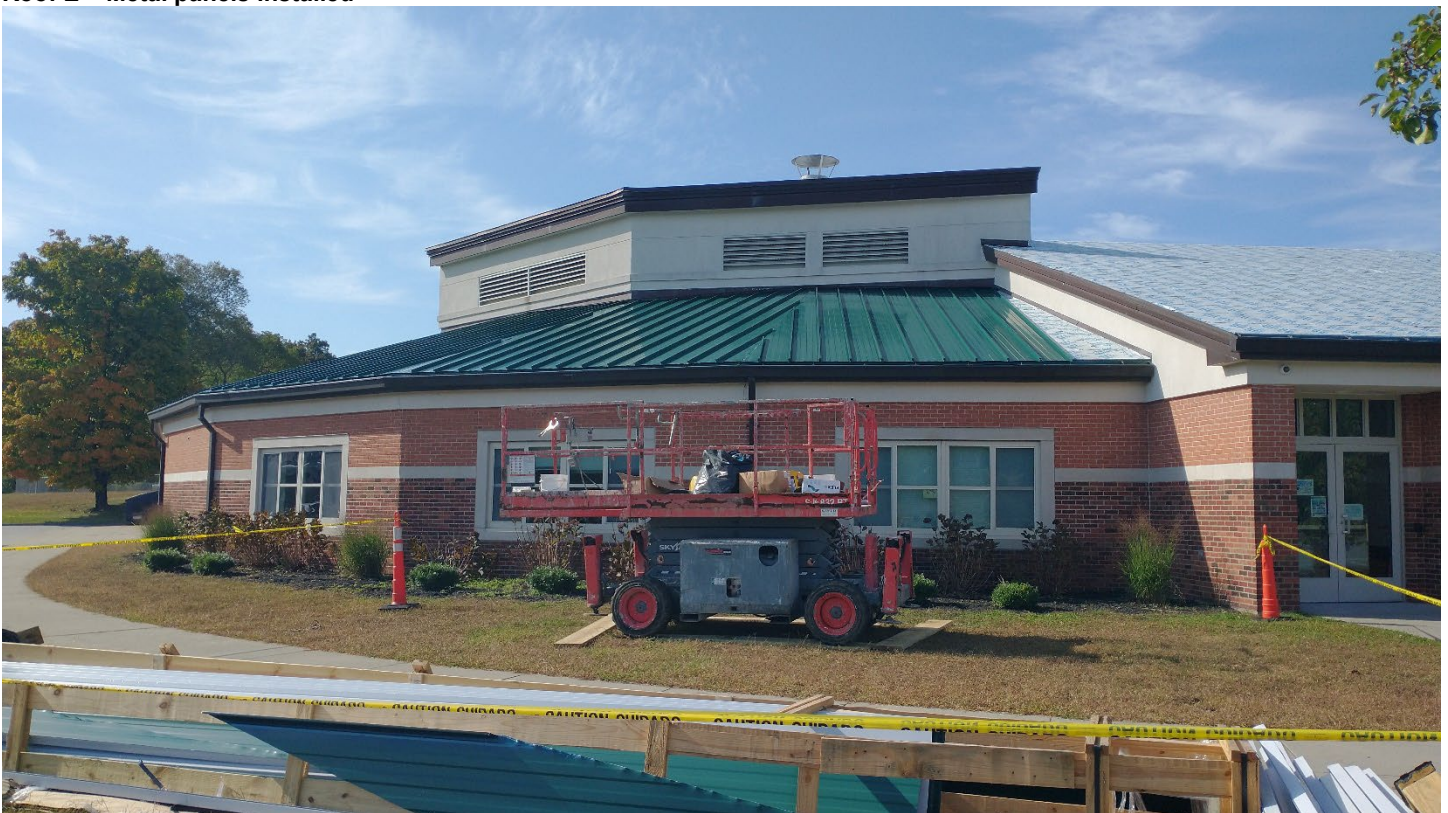
Roof E – Metal panels installed
